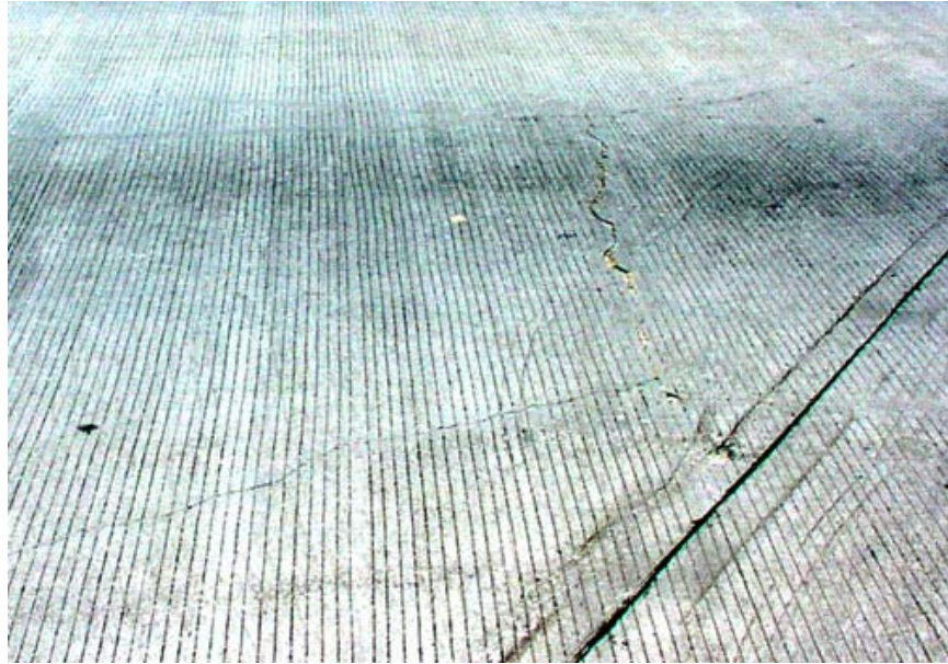
Figure 7. Another Large Crack in Louetta Bridge Deck (Contrast Increased to Highlight Crack)
