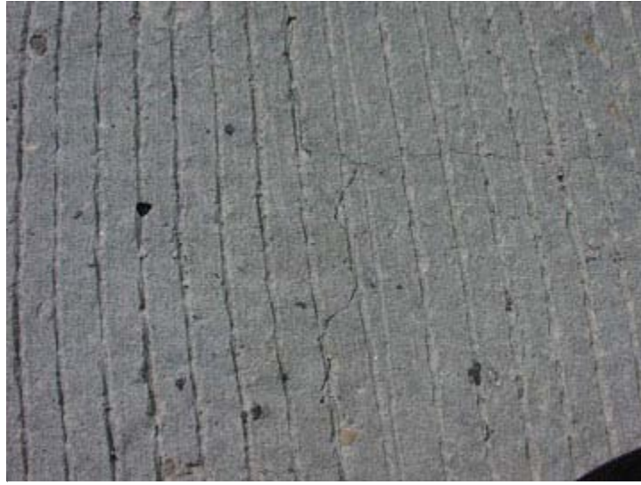
Figure 4. Transverse Cracks in the LP 335 & FM 1061 Bridge in Amarillo
