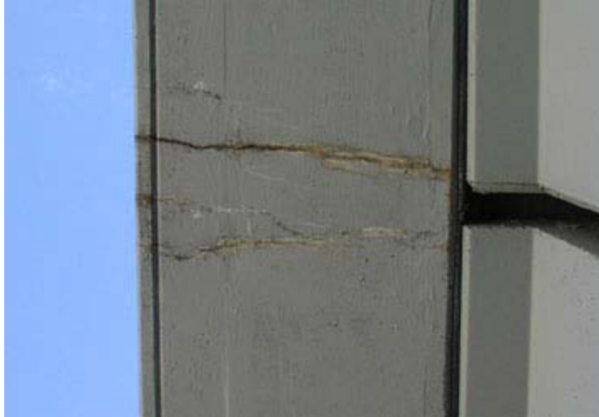
Figure 10. Cracked Soffit Section on Westbound Deck
