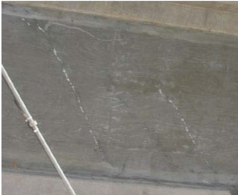
Figure 9. Underside of Cracked Panel in Louetta Bridge
