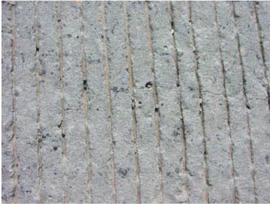
Figure 5. Longitudinal Cracks in the Amarillo Creek Bridge
