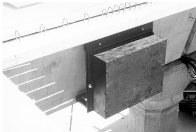
Figure 4.9 Data acquisition system (DAS) box mounted in the bridge
