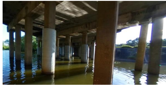
(b) Photography beneath the bridge
