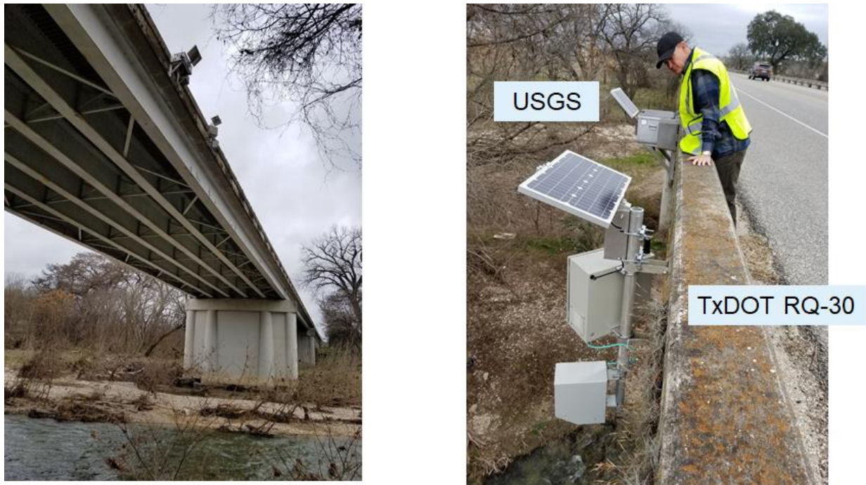
Figure 2-7 Guadalupe River at US-87 near Comfort, Texas
