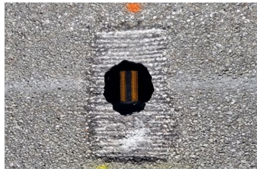
(b) Good Installation with no Residual Bitumen Close to the Marker
