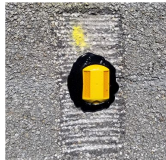
(b) Marker Placed in Bitumen
