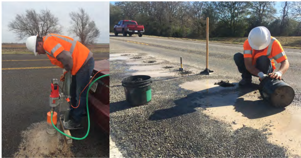
Figure 2.2. Field coring and patching.
