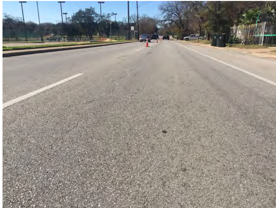
Section #9: 9 years Photo and coring from Dec. 2019 as cracks are beginning to emerge
