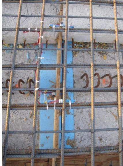
Figure 3- 19 Wood Crack Former
