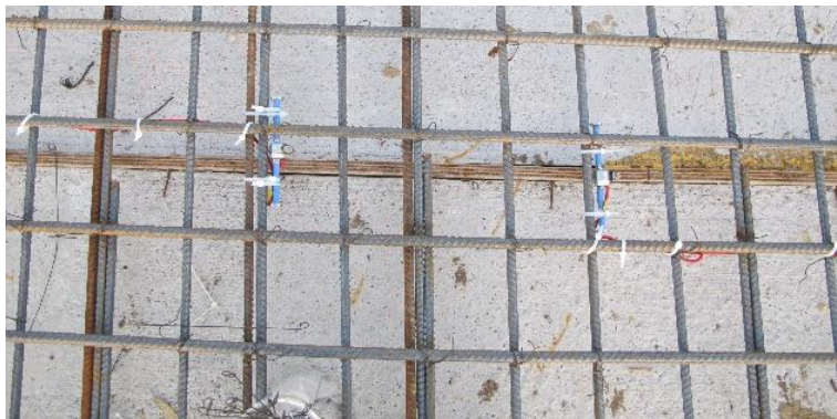
Figure 3- 20 Top Layer Gages over the Crack Former
