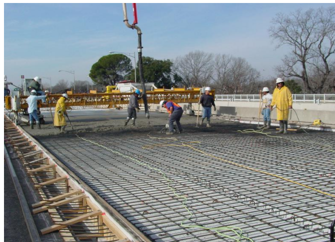
Figure 1-3 Top Mat Reinforcement Over PCPs During Concrete Placement
