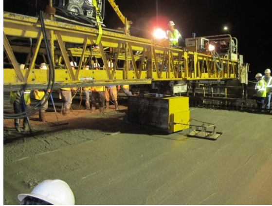
Figure 3- 23 Screed Bridge During Concrete Deck Cast
