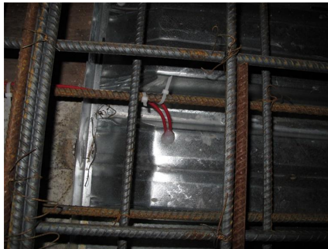
Figure 3- 8 Wires Passing Through The Deck
