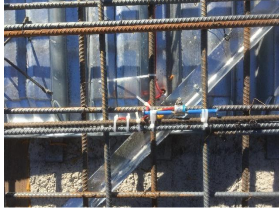
(b) VVG at the edge of a bridge line
