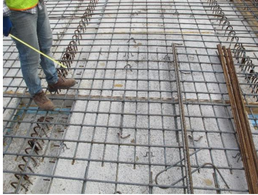
Figure 3- 17 Deck Reinforcing Bars in Bastrop SH71 Bridge
