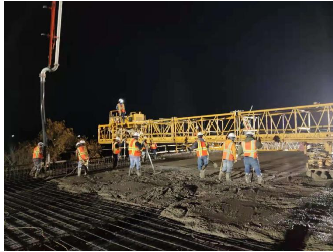
Figure 9- 8 Deck Casting on Feb. 2, 2021
