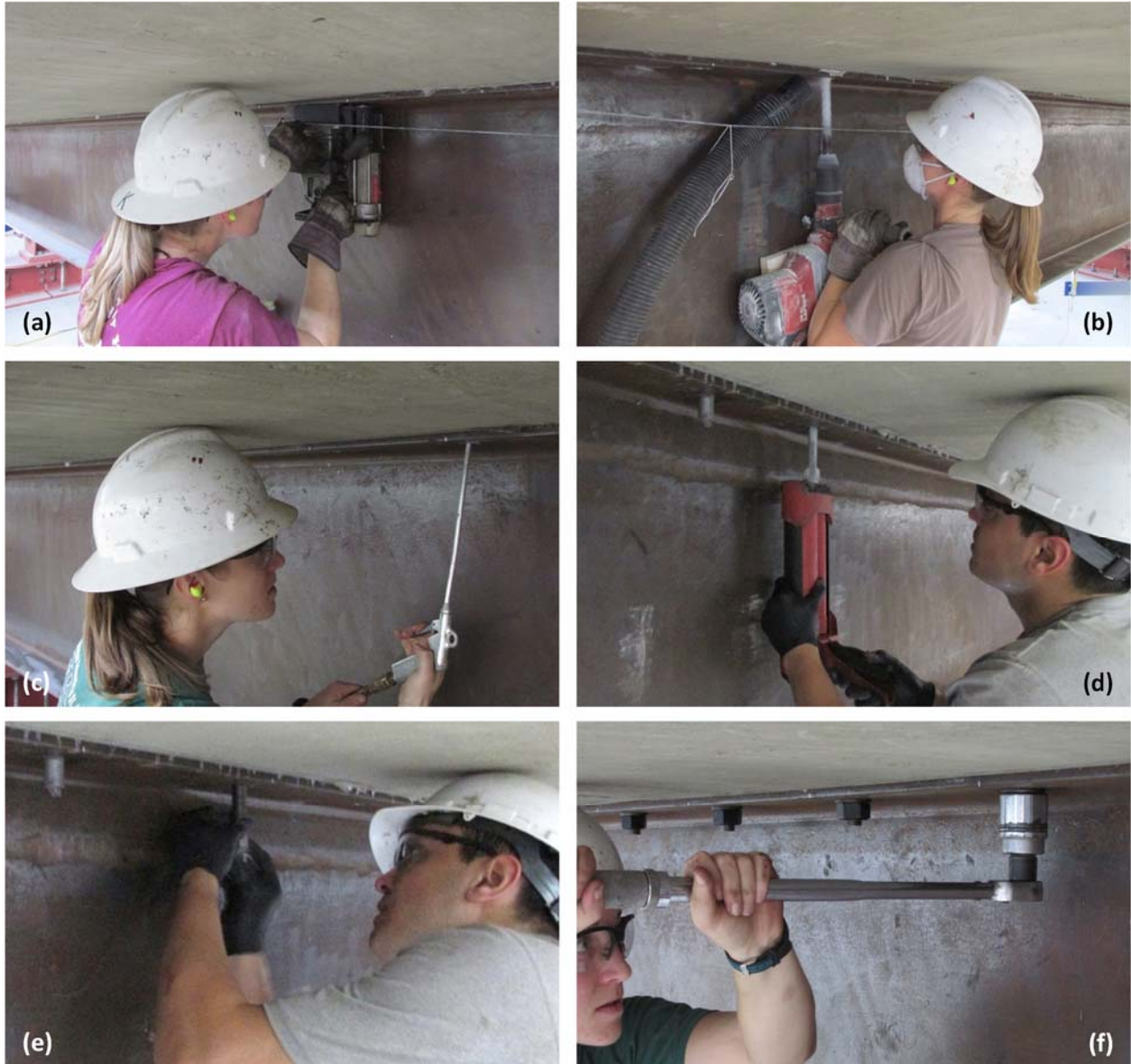
Figure 3.3 Connector Installation
