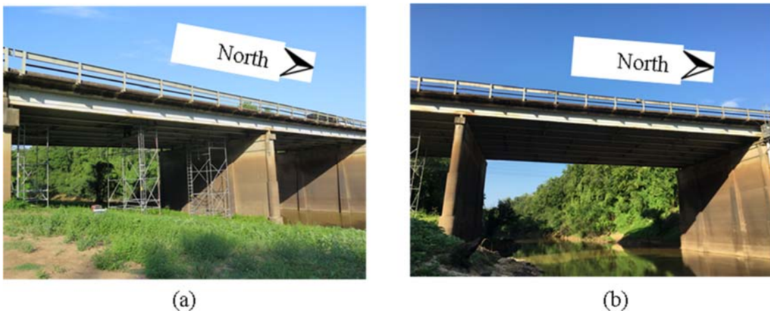
Figure 6.1 Scaffolding Towers Erected for Instrumentation – (a) South Span and (b) Middle Span
