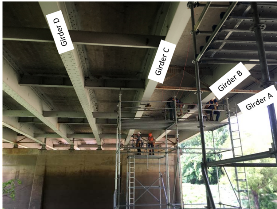
Figure 6.3 Installing Instrumentation on Girders B and C
