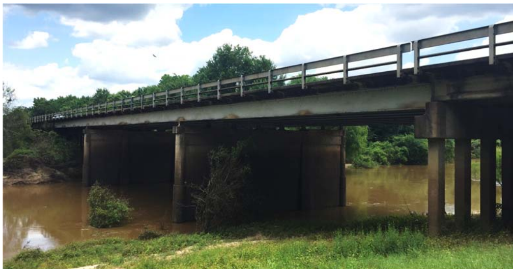
Figure 4.1 Photograph of the Lakeport Bridge
