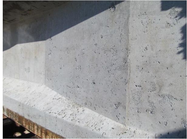
Observed honeycomb in POU girder
