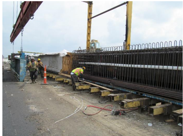
Form removal of Tx62-0SU & close of Tx-0SG
