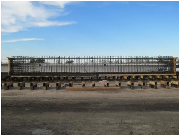
Rebar, PT hardware, and VWGs installation
