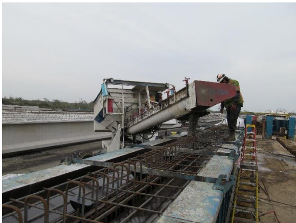
Concrete casting of Tx62-0SG
