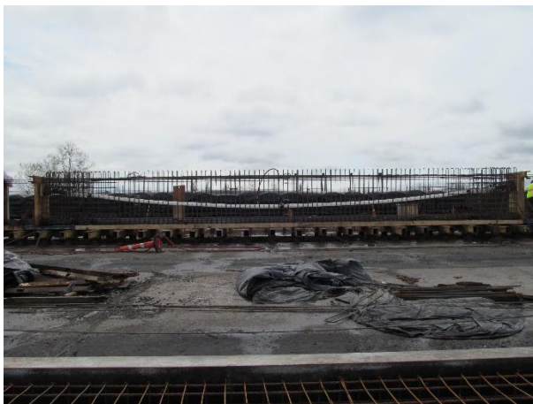
Tx62-P0U girder before concrete placement
