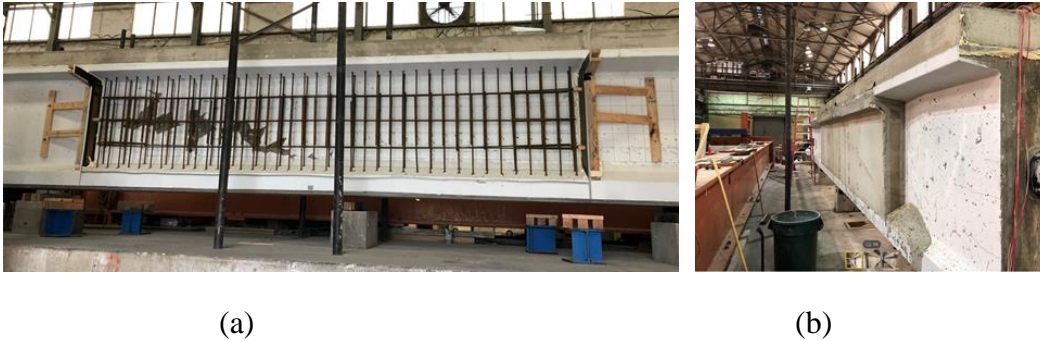
Figure 4.25 CIP Overlay Repair Concrete Placement: (a) Anchored Rebar Cage and (b) Completion of Repair Concrete Placement on Each Damaged Side
