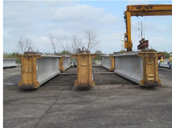
Girders stored in 2 divided rows, ungrouted and grouted
