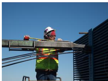
7) Measure elongation of strand at the final strand stressing
