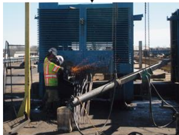
4) Cut redundant strand
