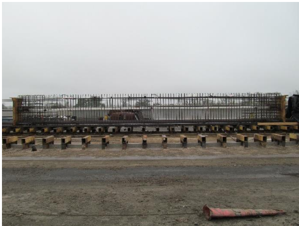
PT, rebar & VWG placement of Tx62-0SG
