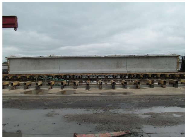
Tx62-0SG girder after side form removal
