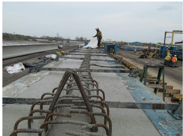
Tx62-0SG covered by curing blanket
