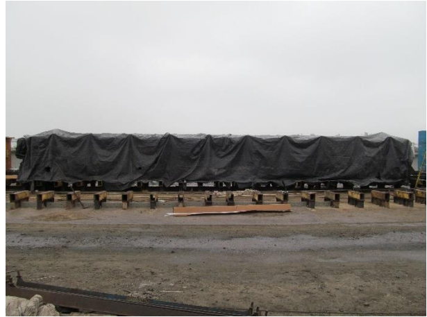
Concrete curing after casting for Tx62-0PU
