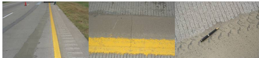
Figure A12. Polymers in Alvarado performed much better than magnesium phosphates after one year
