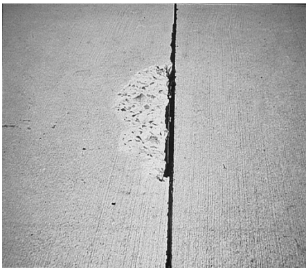
Figure A1. Beginning spall
