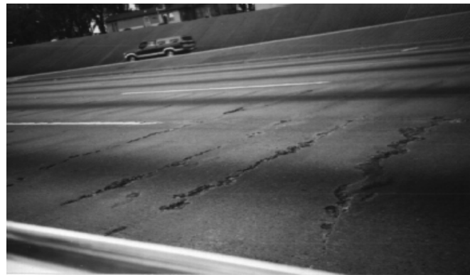
Figure A2. Widespread shallow spalling
