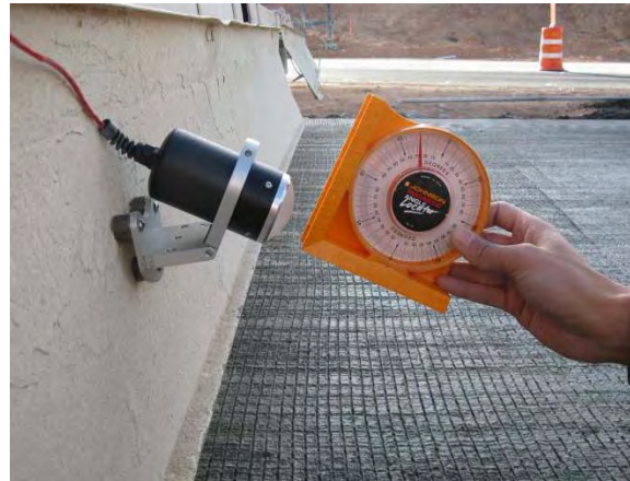
(b) Installation of NDRSS in the front of curing machine
