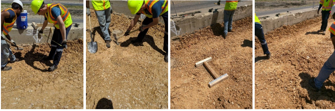
Figure 61. Installation of box-outs
