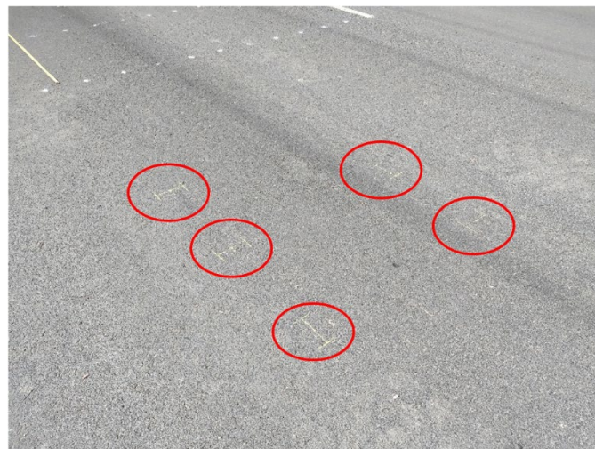
Figure 77. Marking ASG locations
