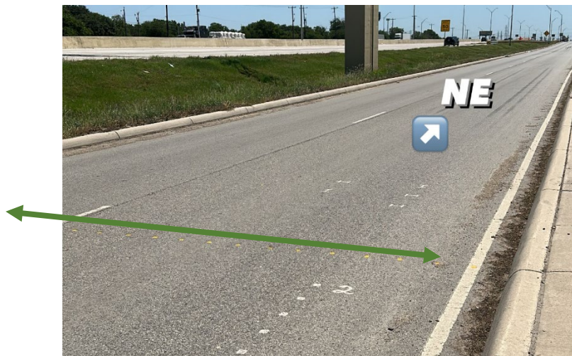
Figure 89. Transverse road section for total station measurement in section 2
