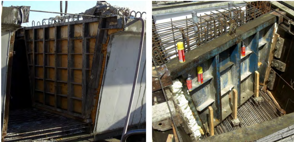
Figure 4.35: Exterior Formwork—Bexar (Left) and Eagle Lake (Right)
