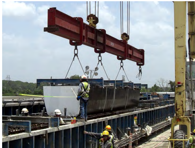
Figure 4.1: Installation of U54 Male Formwork
