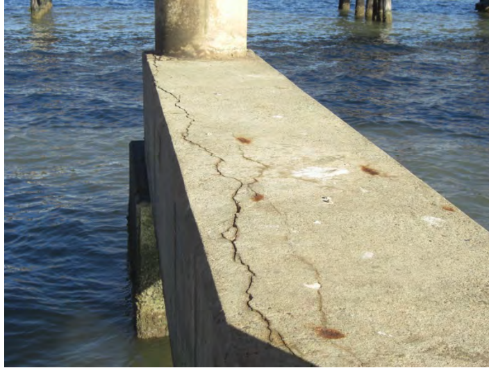
Figure 6.4: Cracking of Tie Beam
