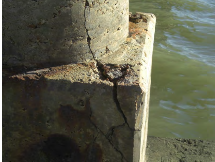
Figure 6.2: Corrosion of Tie Beam and Column
