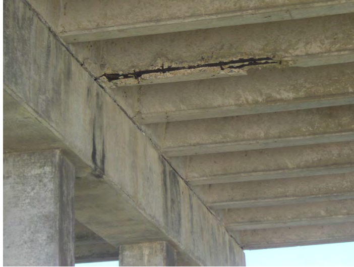
Figure 6.6: Corrosion of Concrete Slab and Girder Span
