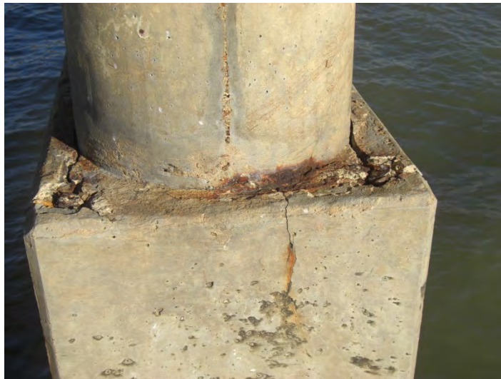
Figure 6.3: Cracking of Tie Beam and Column
