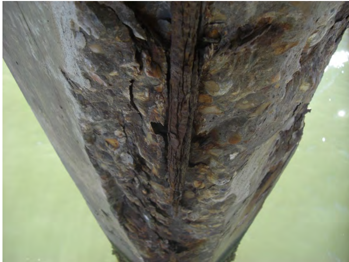
Figure 6.5: Corrosion of Precast Concrete Piling
