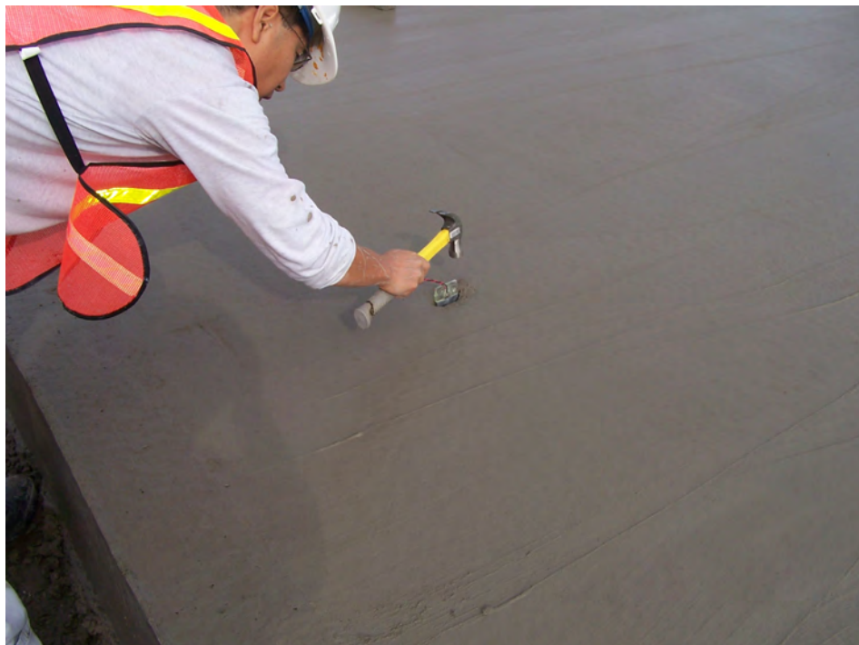
Figure 3.2 Installation of I-button Assembly into Concrete Pavement
