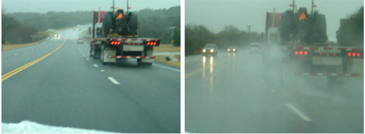
Figure 1.1: Difference in Spray from Conventional and PFC Pavements
