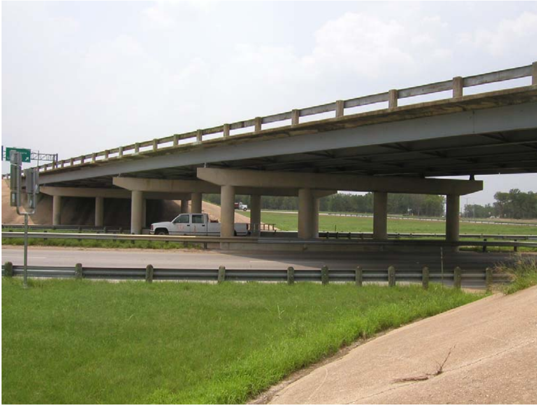
Figure 2.5: Texas 71/US 183 Overpass
