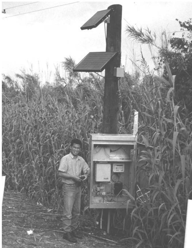
*Figure 2.15 Aluminum cabinet and solar panel mounted on wooden pole*
