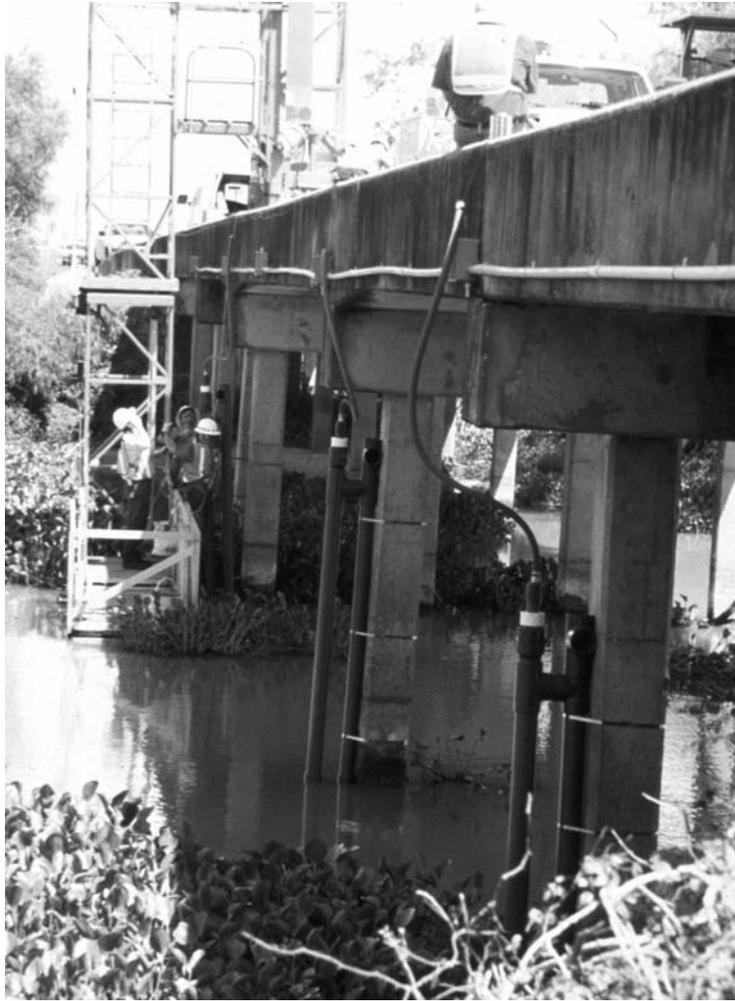
*Figure 2.10 Snooper crew during installation*
