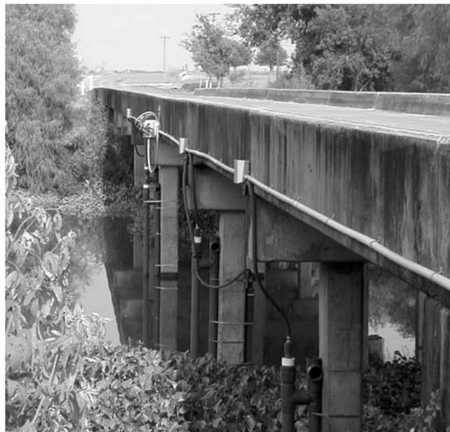
Figure 3.4 H-240 enclosure and sensor assemblies
