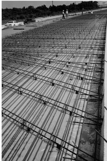
**Figure 1.12 Metallic crack inducer located on top of longitudinal rebar**
