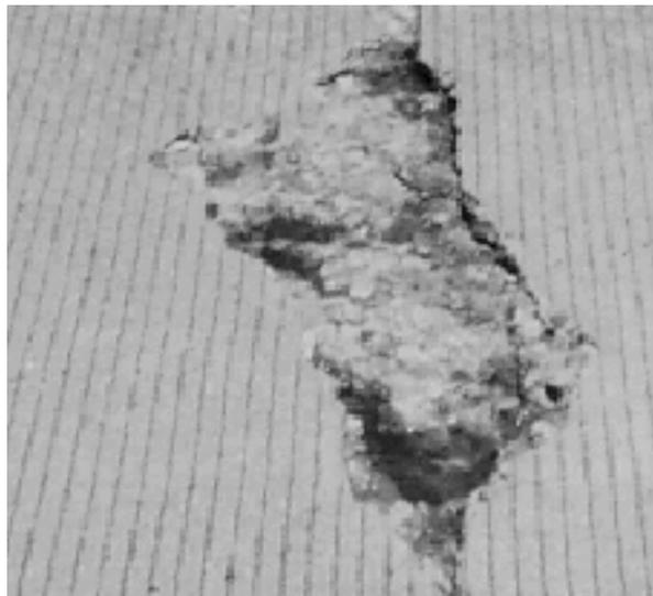
*Figure 2.3 Example of deep delamination spalling*
