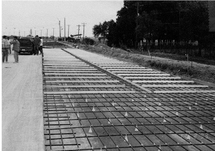
*Figure 1.7 Type I crack inducer located in TS1*
