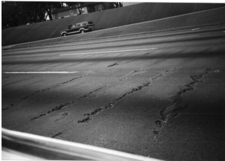
*Figure E1 Typical spalling of a pavement*
