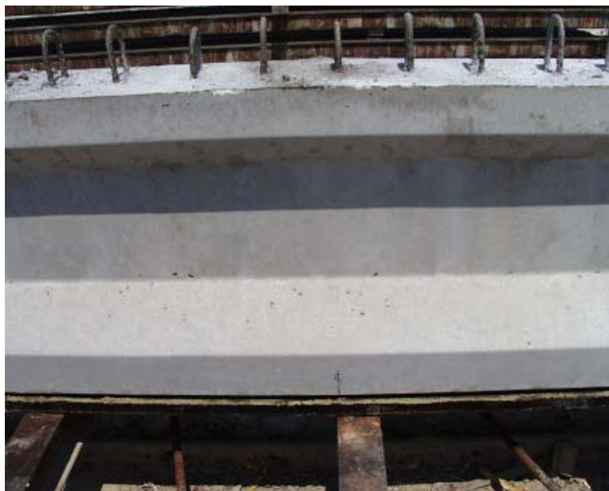
Figure 1 Finish of Girder with 8000 psi Concrete Mix
