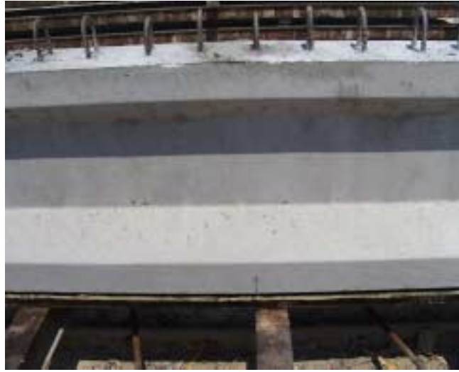
Figure 5.10 Finish of Girder with 8000 psi Concrete Mix
