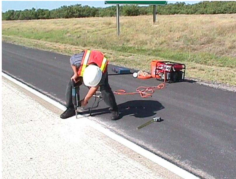
Figure 4.1 Generator and drill used for drilling the concrete pavement
