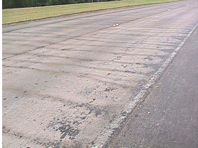
Figure 4.8 Image of CRCP underneath the AC layer that was milled off
