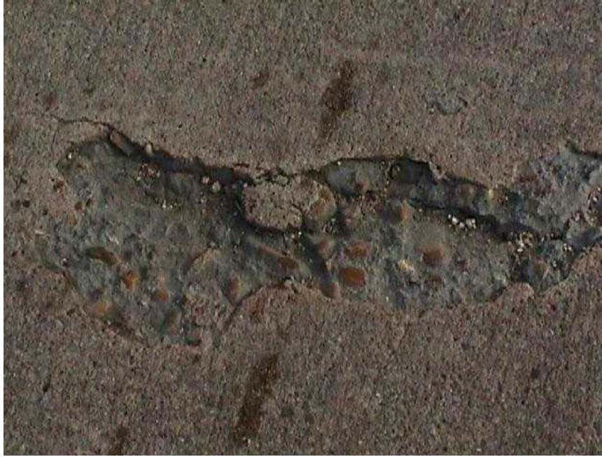
Illustration 5 Severe spall found in the SRG section
