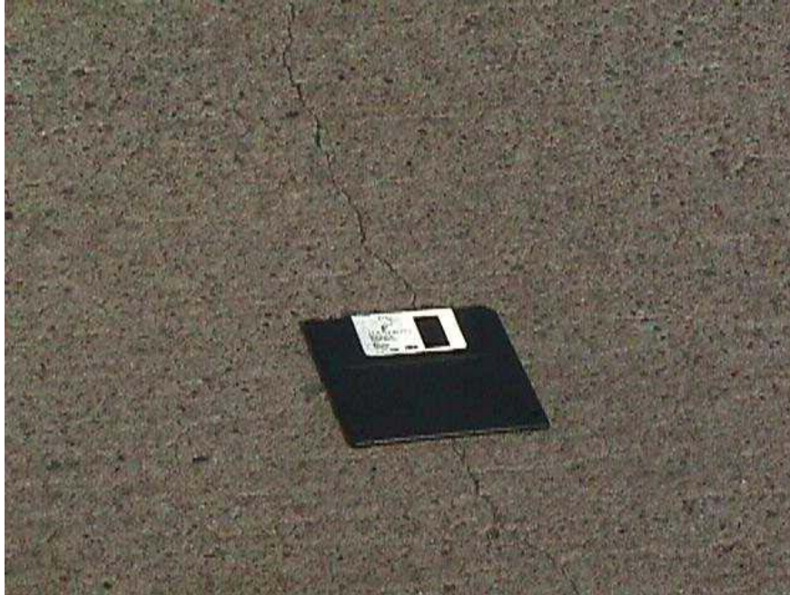
Illustration 7 Common transverse crack found in the LW section
