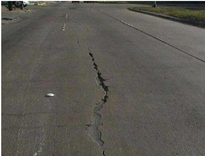
Illustration 2 Longitudinal crack found in the SRG section
