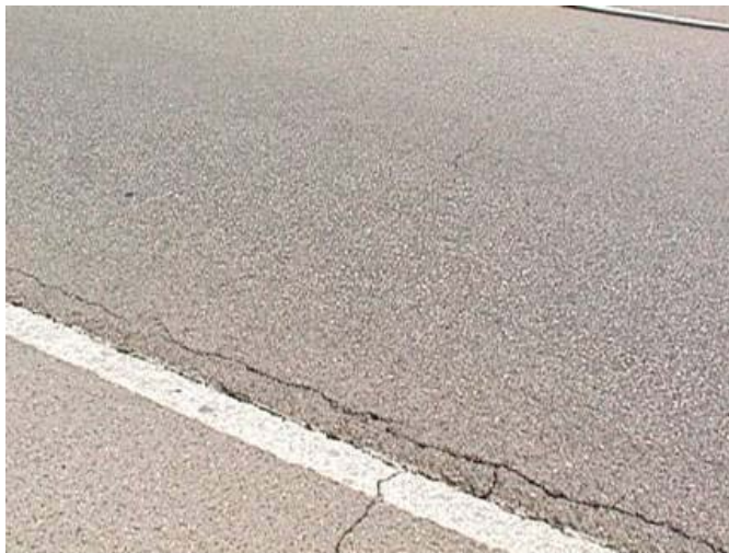
Figure 4.14 Longitudinal crack in Section 17006-1 on SH 6 in Brazos County
