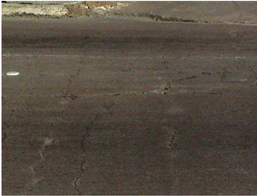
Illustration 1 Transverse cracking and spalls found in the SRG section
