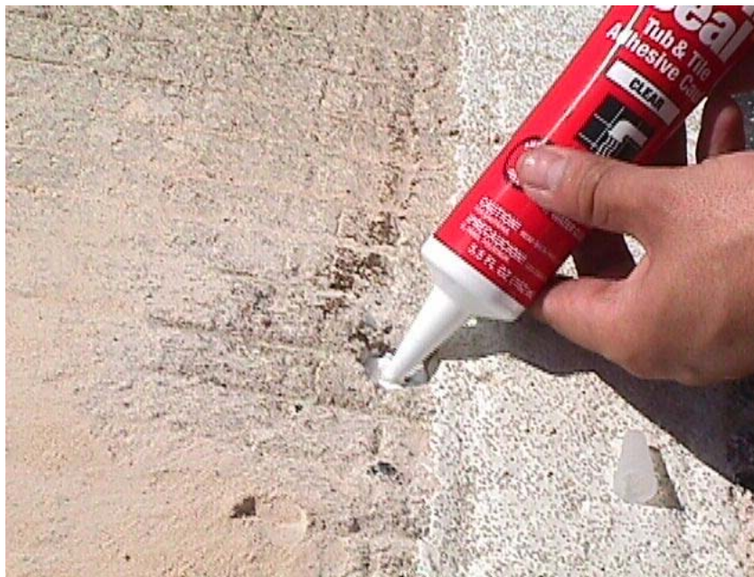
Figure 4.6 Filling silicone used to protect the connecting wire inside the hole
