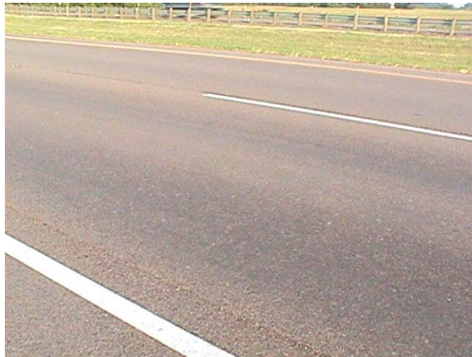
Figure 4.7 Shallow rutting (<0.5 in.) and flushing of asphalt on Section 13010-1
