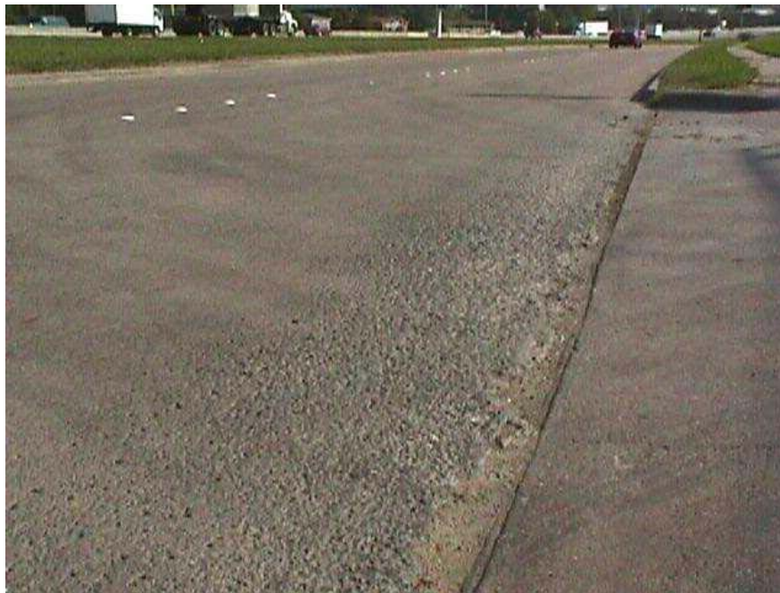
Illustration 8 Localized raveling of the concrete of the LW section
