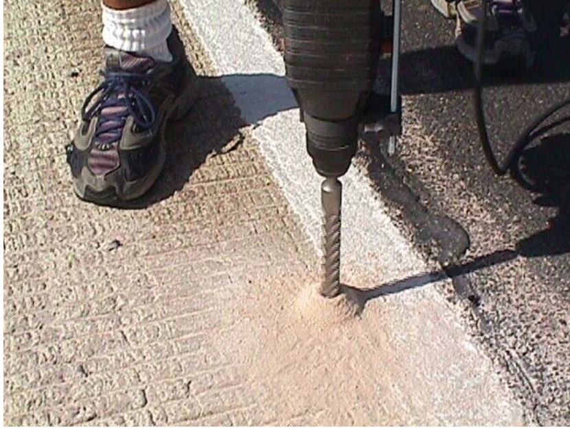
Figure 4.2 Heavy-duty \frac{3}{4} in. diameter bit used in drilling operations
