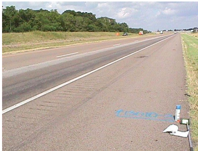
Figure 4.9 Image of rutted and flushed wheel paths of the outside lane
