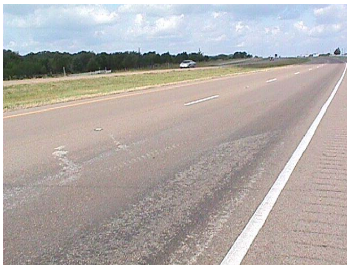
Figure 4.10 Ending zone of distressed asphalt layer, Section 13010-4
