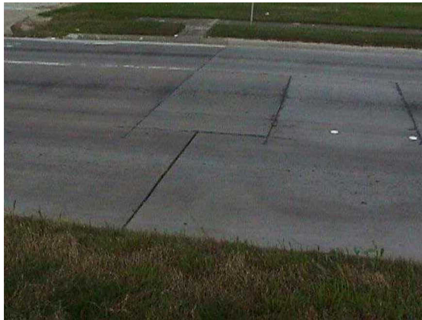
Illustration 4 Portland cement patch (PCC) found in SRG section
