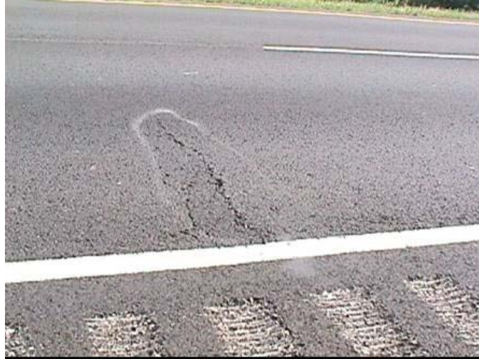
Figure 4.19 AC Overlay distress in Section 19020-8
