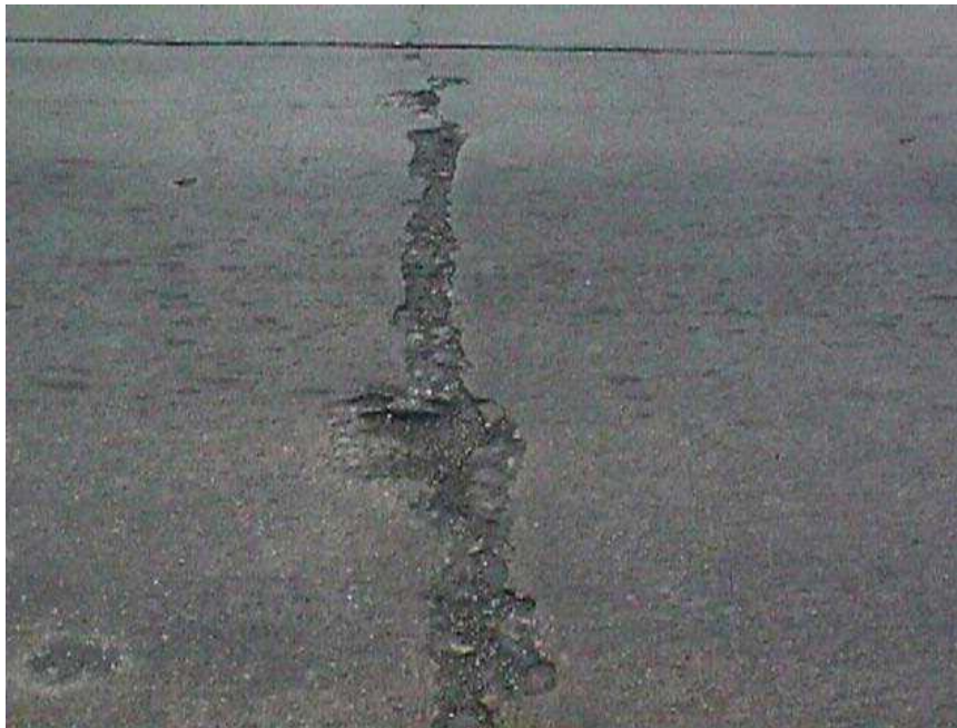
Illustration 6 Spalled transverse crack found across the lane, SRG section
