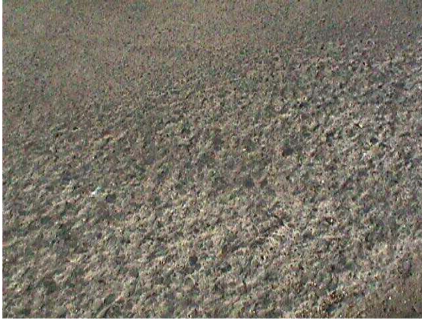
Illustration 9 Zoomed image of the raveled concrete in the LW section
