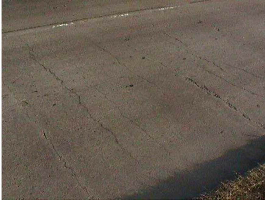
Illustration 3 Transverse cracking pattern for the SRG section
