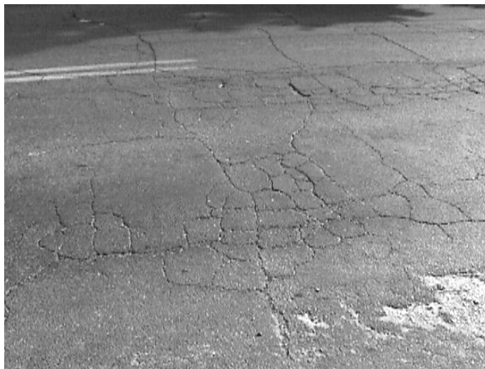
FIGURE E.9 ALLIGATOR CRACKING
