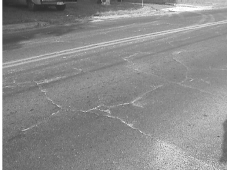
FIGURE E.10 BLOCK CRACKING
