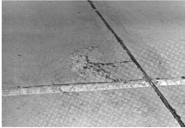
FIGURE E.7 DURABILITY D-CRACKING
