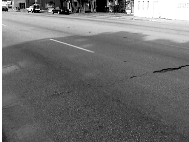
FIGURE E.4 SPALLED CRACK
