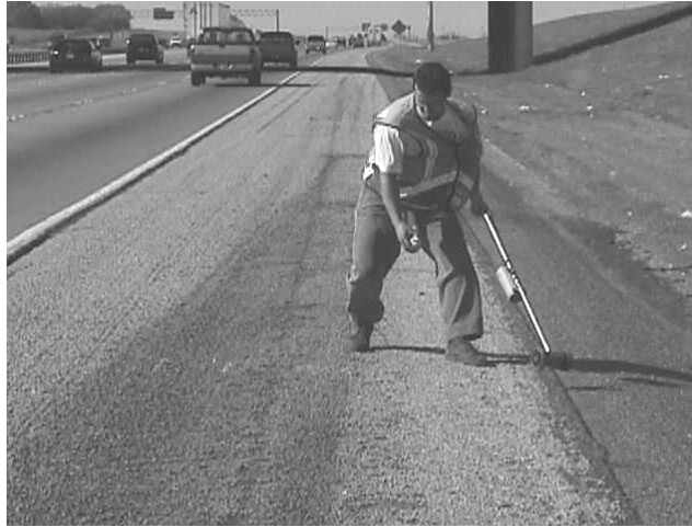
Figure F.2 Surveyor painting the CFTR number of a section
