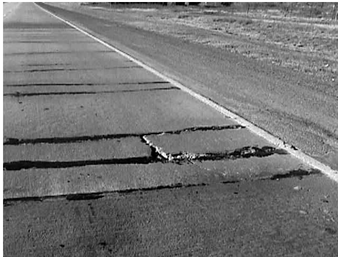
FIGURE E.6 SEVERE PUNCHOUT
