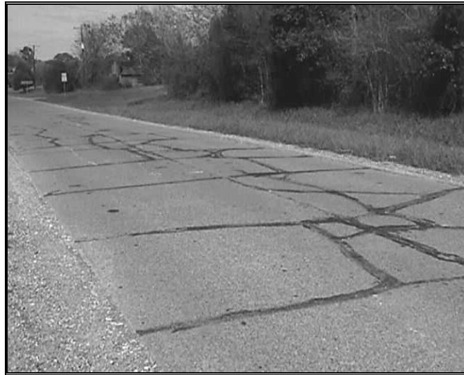
FIGURE E.2 TRANSVERSE AND LONGITUDINAL CRACKS
