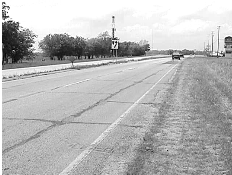
FIGURE E.11 REFLECTION CRACKING
