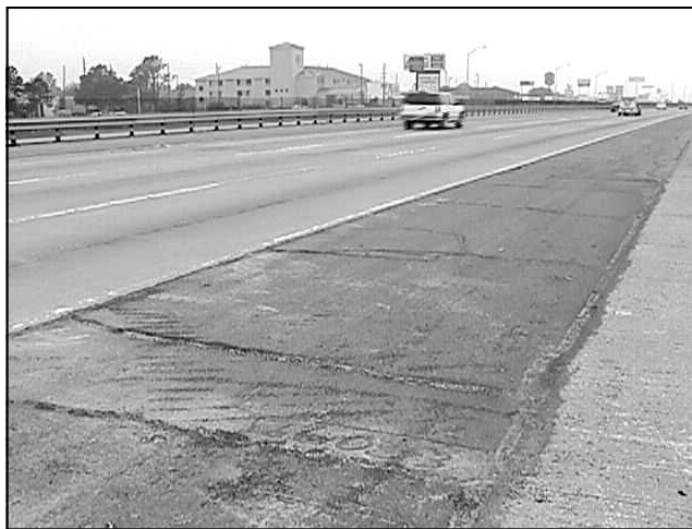
FIGURE E.8 CRACKED AND SPALLED SHOULDER
