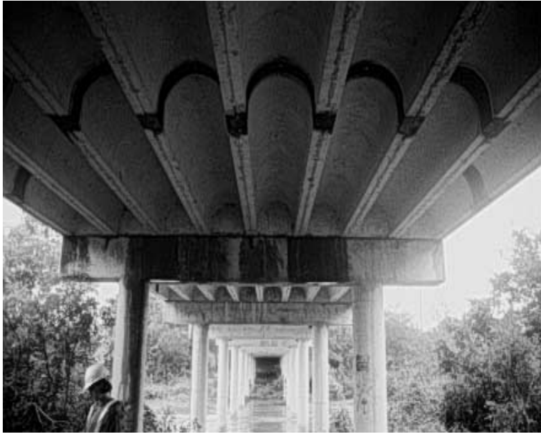
Figure 3.2 Photograph of Pan-Girder Bridge in Buda, Texas Indicating Uneven Surfaces on Bottom of Joists
