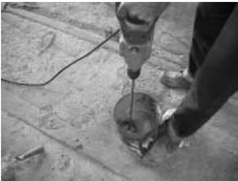
c) Mixing epoxy paste
