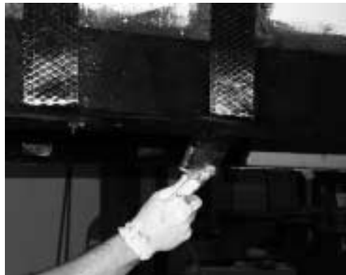
f) Coating placed sheets with epoxy
