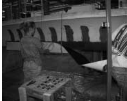
e) Eliminating air bubbles from sheets
