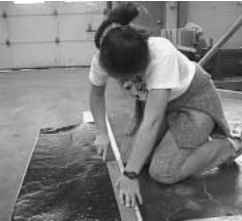
c) Applying epoxy to surface
