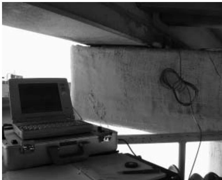
Figure 7.2 PR-Monitor test setup for Structure #12
