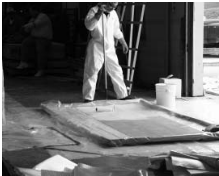
Figure 8.3 Saturating glass fabric with epoxy resin
