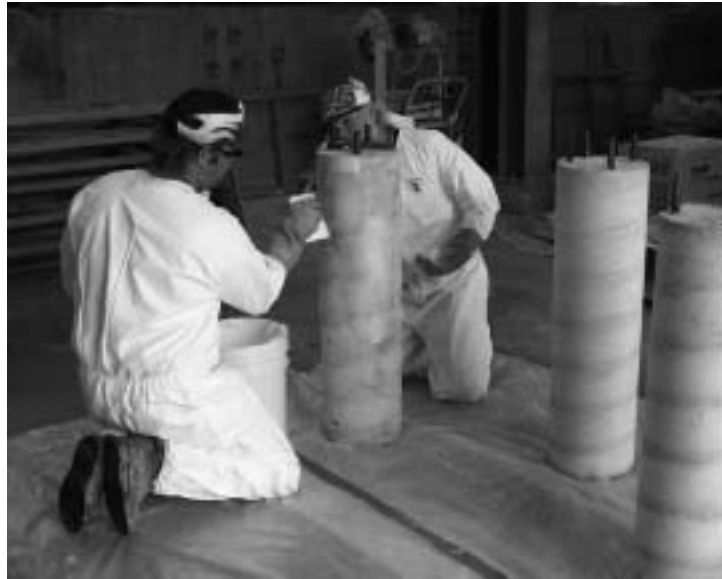
Figure 8.2 Filling voids with a thickened epoxy filler
