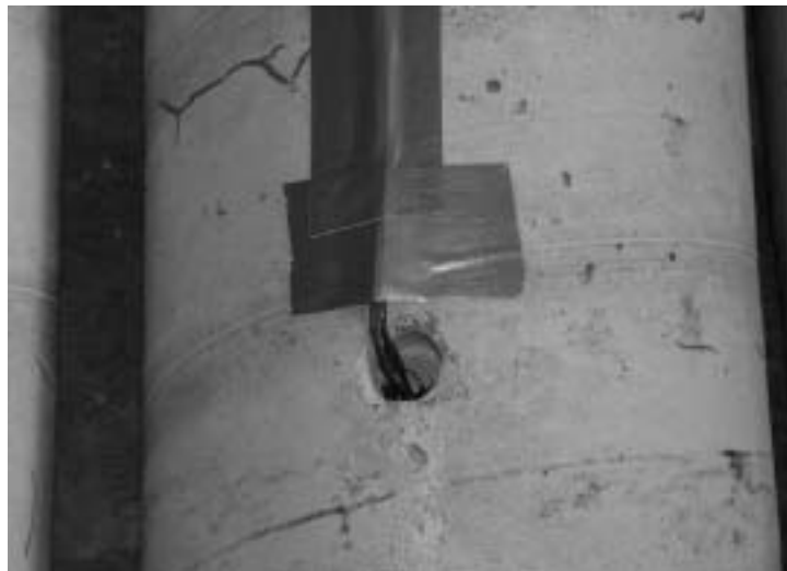
Figure 8.6 Installation of the embedded electrodes
