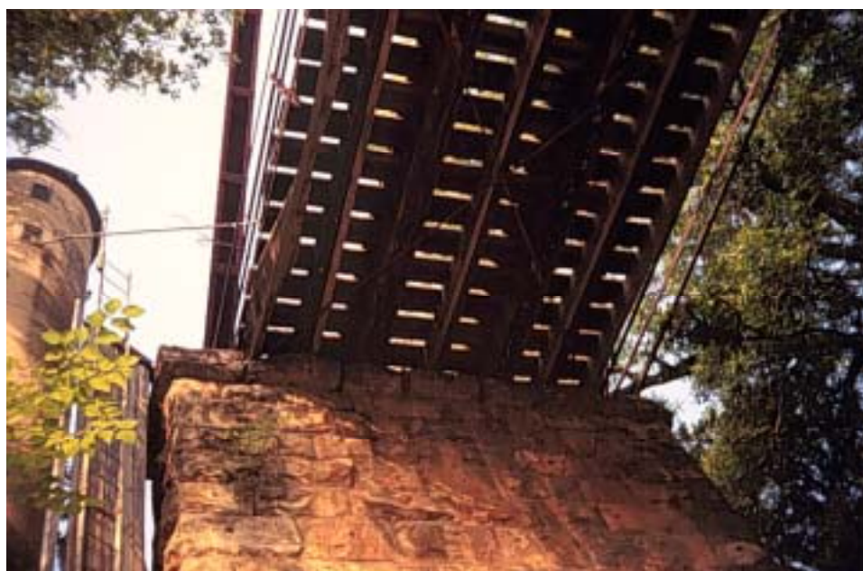
Figure A.29: Timber stringers of the main truss span resting on the south pier
