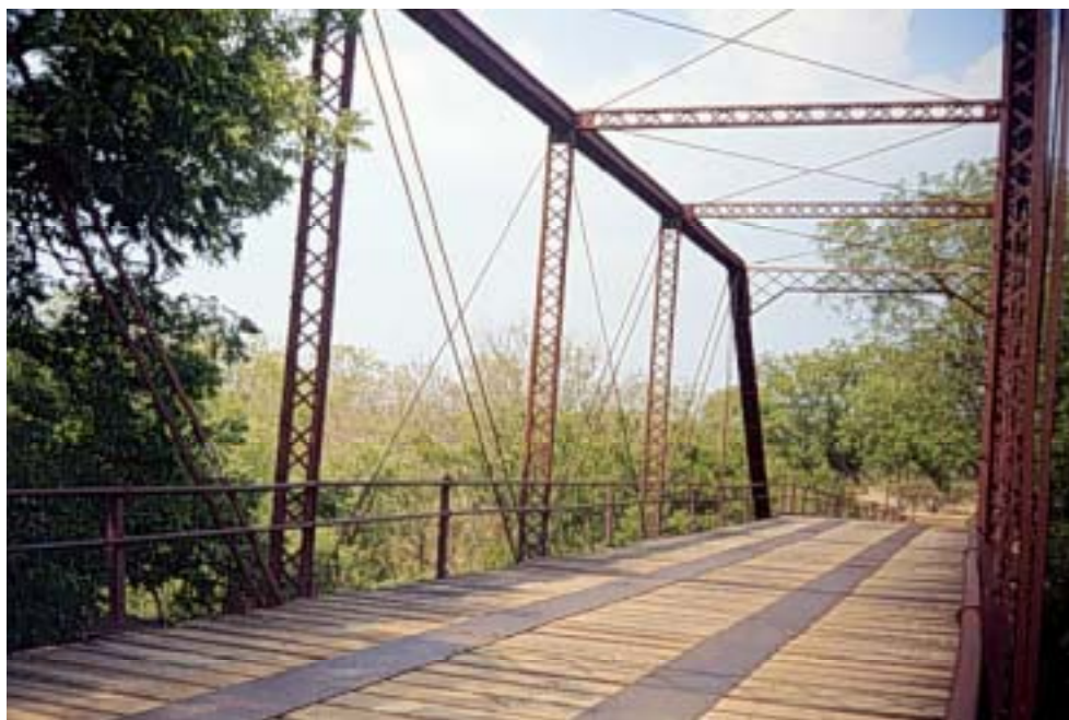
Figure A.5: Upstream truss
