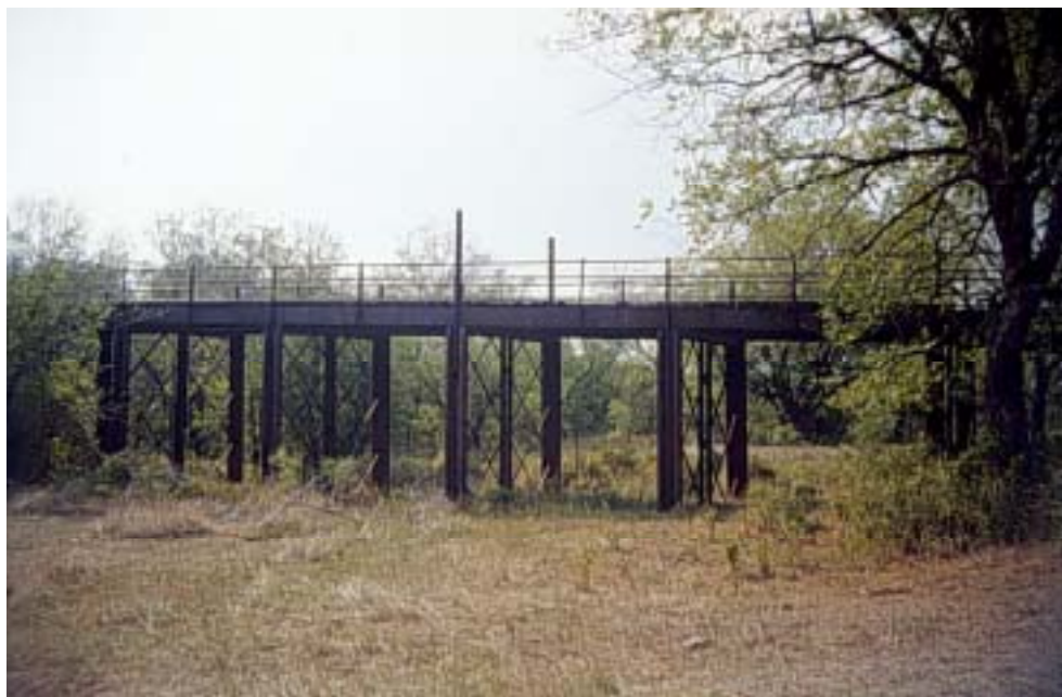
Figure A.4: North approach span
