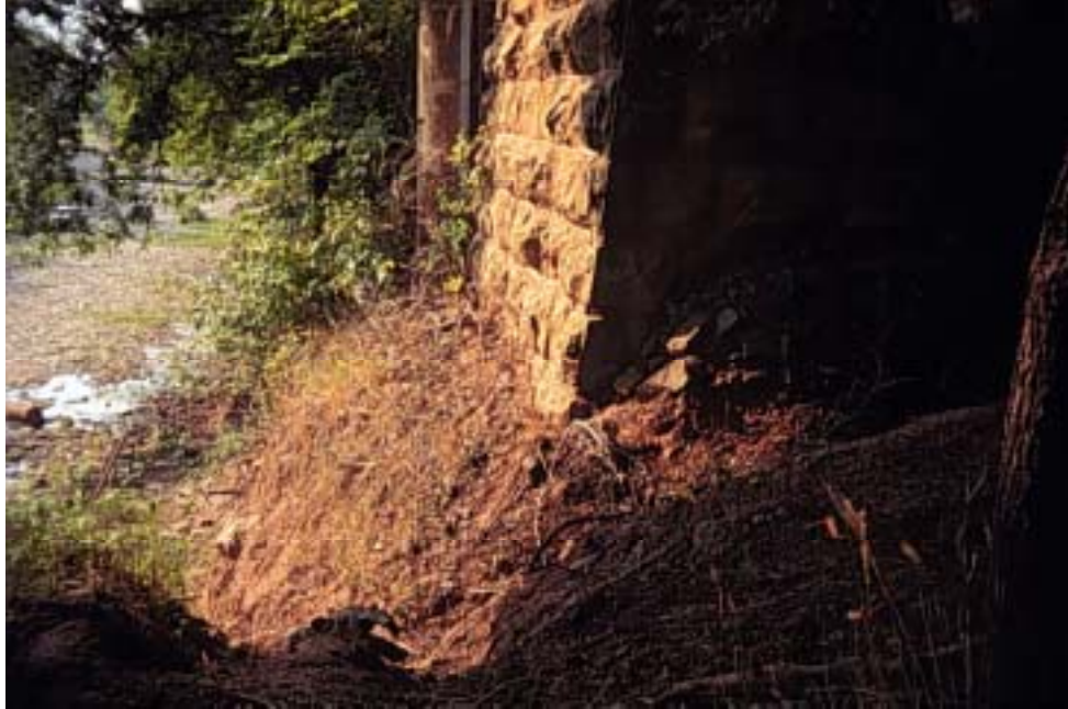
Figure A.30: Base of the south pier
