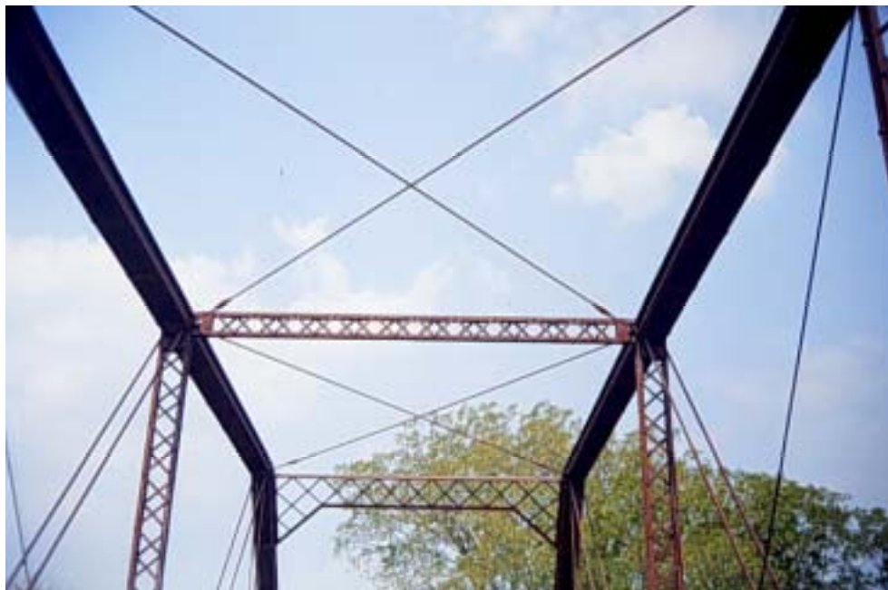
Figure A.21: Top lateral bracing system
