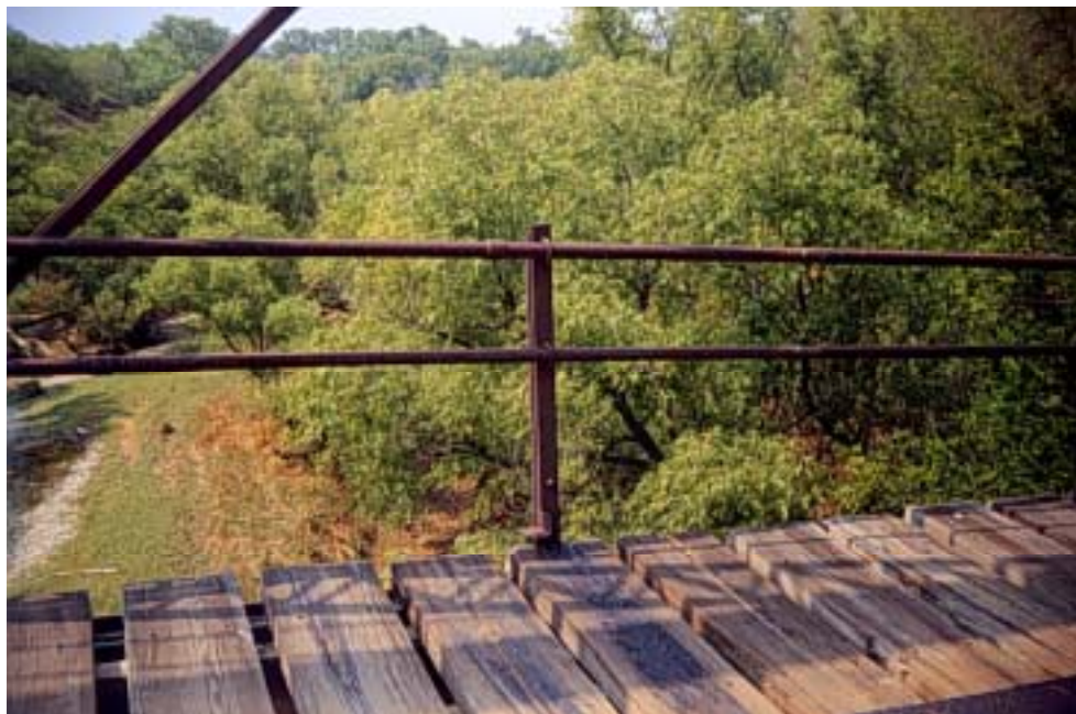
Figure A.23: Metal railing
