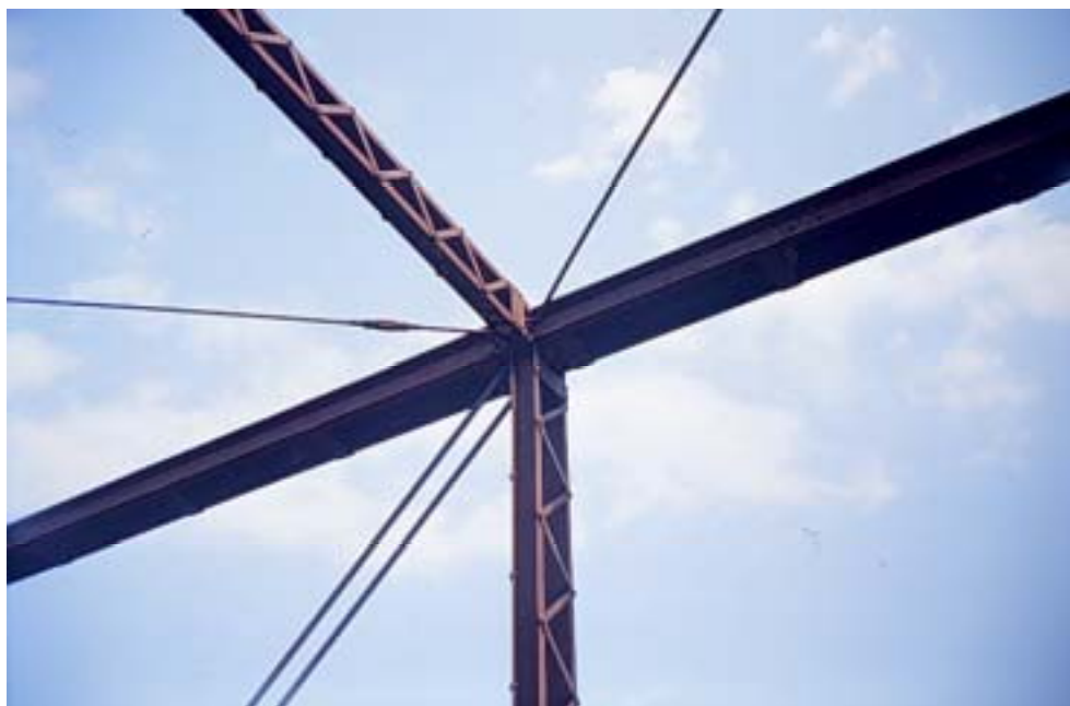
Figure A.15: Upper chord joint U2
