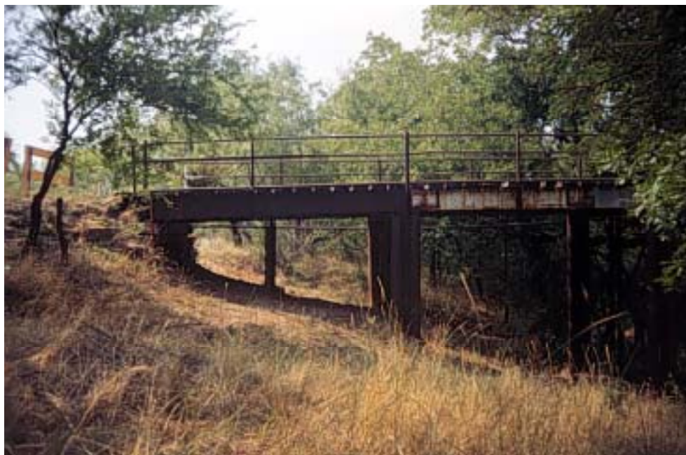
Figure A.2: South approach span
