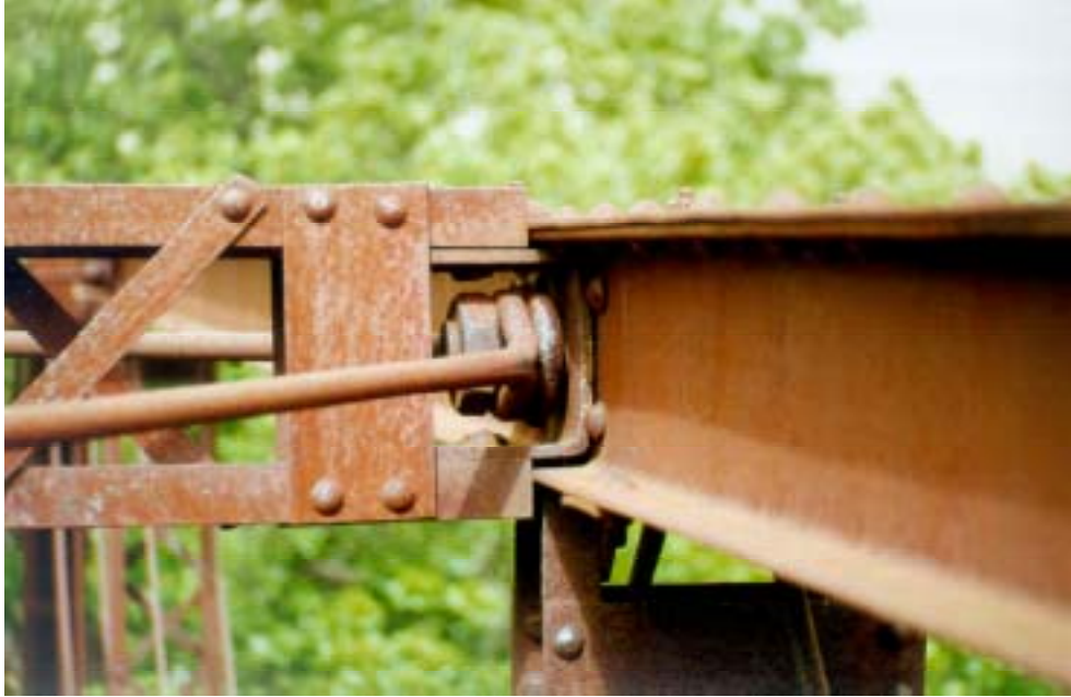
Figure A.16: Top bracing connection
