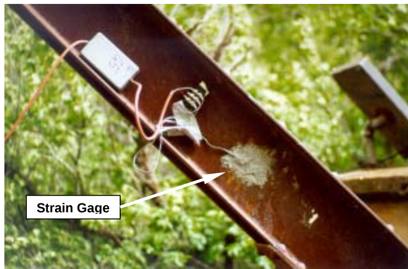
Figure 5.1: Typical strain gage installed on bridge member
