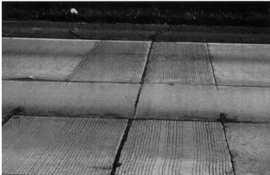
Figure 9.24 Photograph of Typical Patched Joint from IH-10 in Houston, Texas
