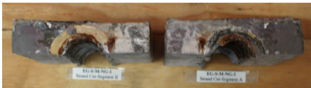
Figure 4.28 Incomplete Epoxy Coverage in Epoxy/Gasket Joint (EG-S-M-NG-1).
