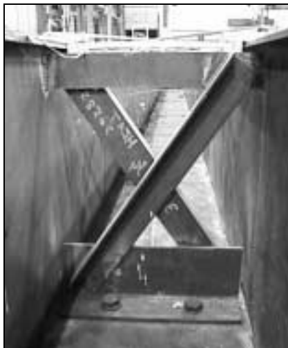
Figure 3.7 X-Brace at Support Location
