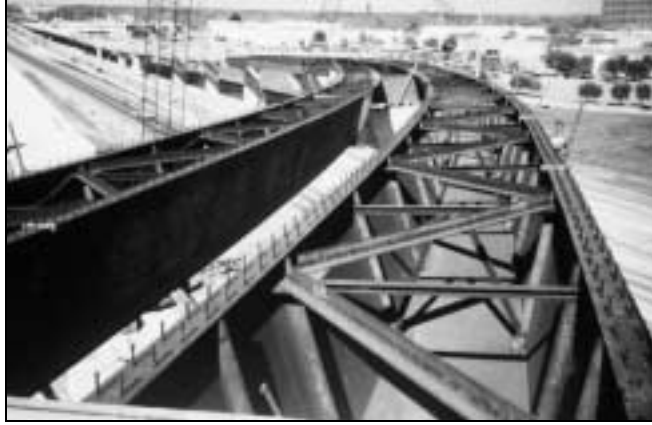
Figure 1.3 U-Shaped Girders During Erection (Gilchrist, 1997)
