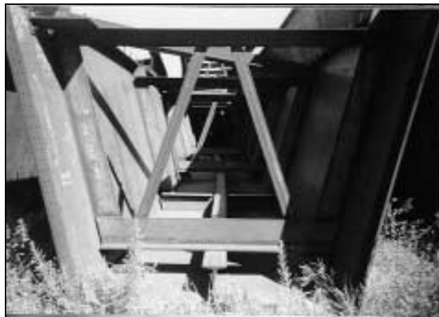
Figure 1.2 Cross Section of U-Shaped Girder Segment (Gilchrist, 1997)
