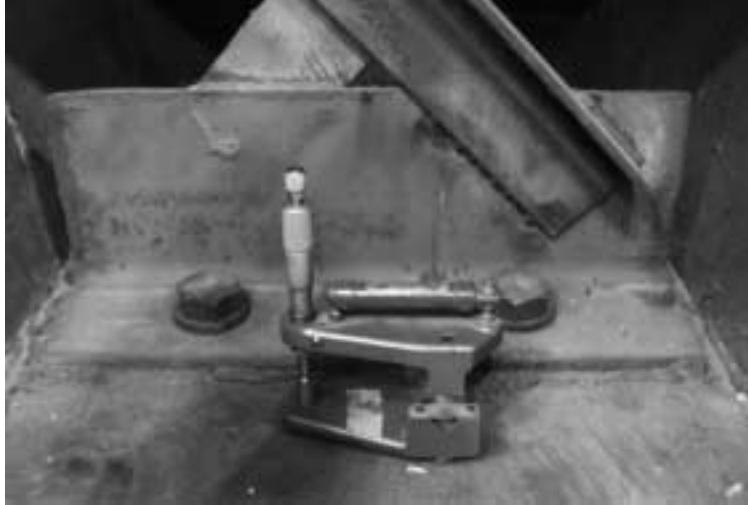
Figure 7.4 Bubble Level at South Support
