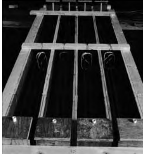
Figure A.9 Formwork for beam specimens.
