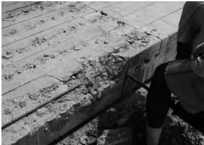
Figure A.59 Beam demolition for bar retrieval.
