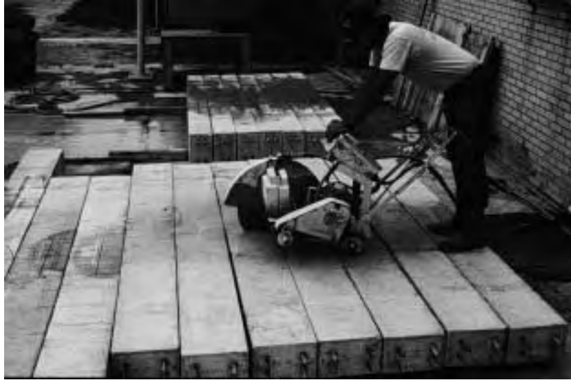
Figure A.58 Saw used to crosscut beams.
