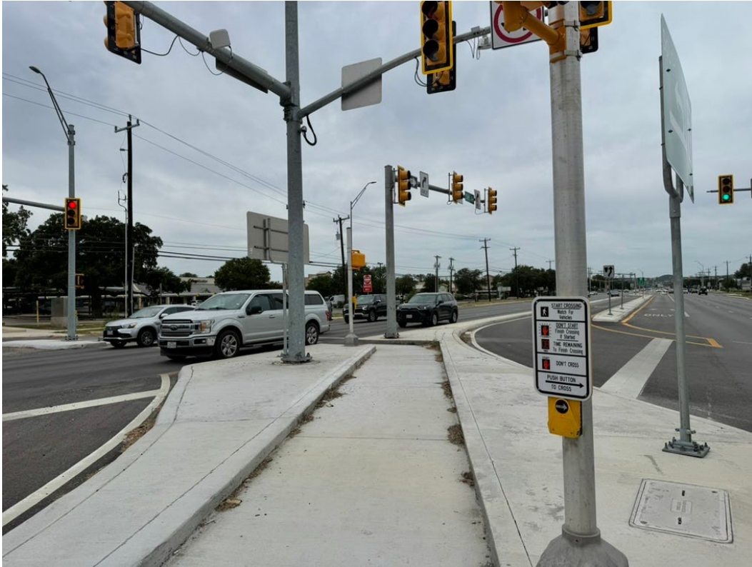
Figure 32. Image of the center pedestrian island at the RCUT (Bandera Rd & Cedar Drive, San Antonio, July 2025)
