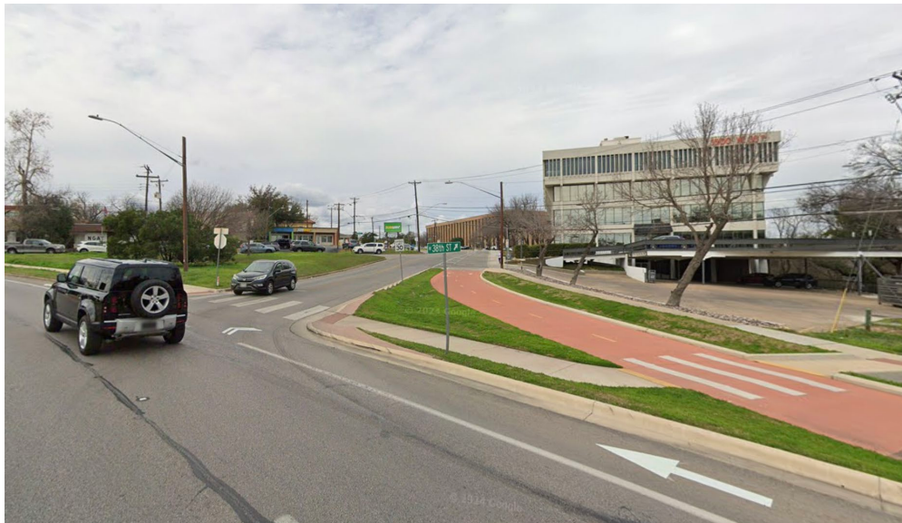
Figure 17. An example of a removed channelized turn lane transformed into a bike path at W 38th Street and W 35th Street, Austin, Texas (Google, n.d.).
