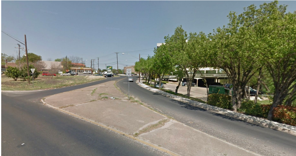
Figure 16. An example of a channelized turn lane before removal at W 38th Street and W 35th Street, Austin, Texas (Google, n.d.).
