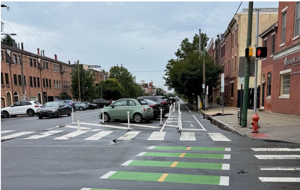
Figure 14. Curb extension with quick-build materials in Philadelphia (taken: Bainbridge Street & S 11 th Street, July 2024).
