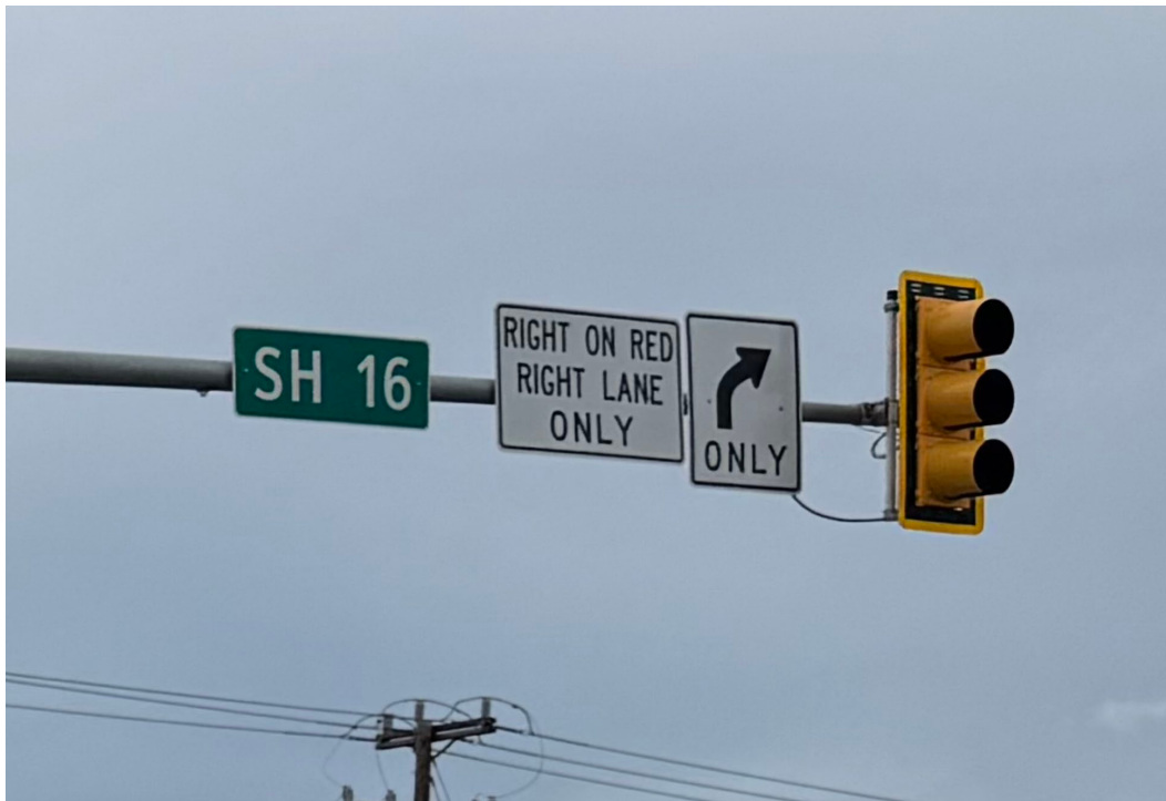
Figure 34. Right On Red Signage at RCUT Intersection (taken: Bandera Rd & Cedar Trl, San Antonio, Texas July 2025)
