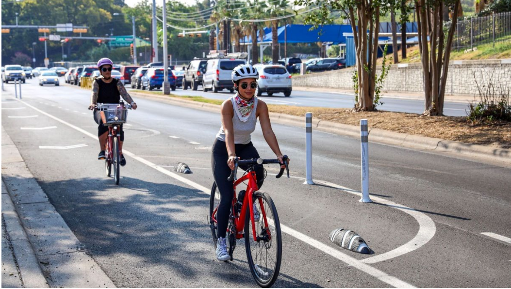
Figure 13. The City of Austin's Barton Springs Pilot Project, showing temporary materials used for a protected bicycle lane (James Rambin 2024).
