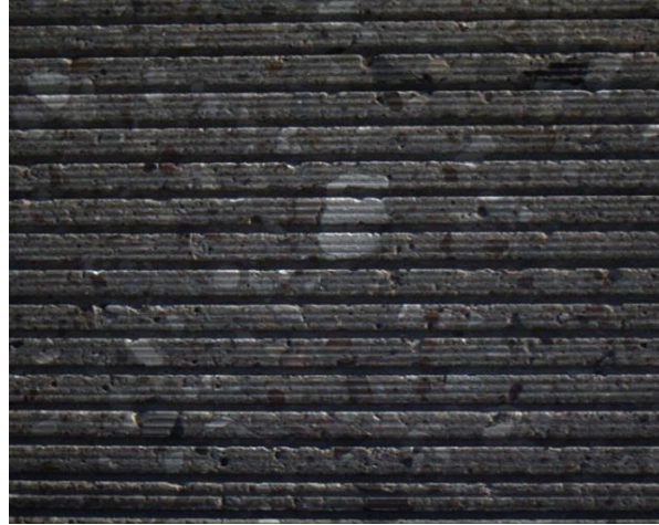
Figure 28: Field picture for texture constructed in hardened PCC using NGCS.
