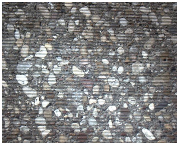
Figure 26: Field picture for texture constructed in hardened PCC using conventional diamond grinding
