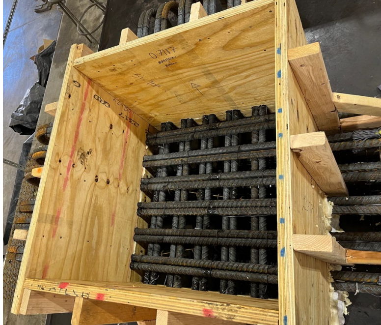
Figure 6-9 Wooden formworks with the bracings and the bottom mat reinforcement
