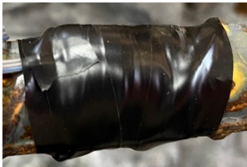
(e) Electrical tape wrapping
