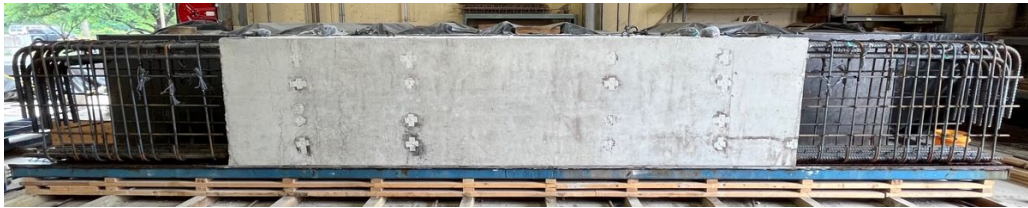
(c) Steel cage fabricated for the exterior section
