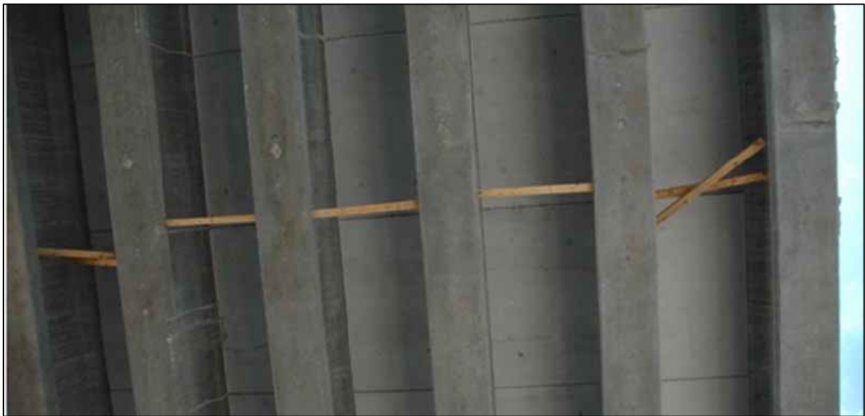
Figure 2.22. Underside of superstructure (looking up), temporary blocking, Yang et al. (2010)
