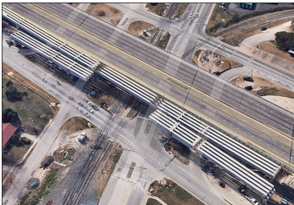
(b) Aerial view of the bridge during construction from Google Maps/Earth
