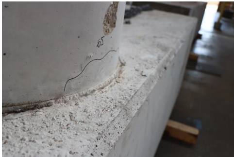
(a) Concrete crushing
