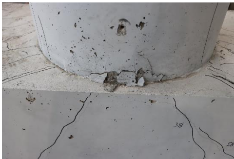
(a) Concrete crushing
