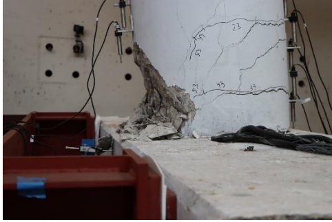
(a) Concrete crushing
