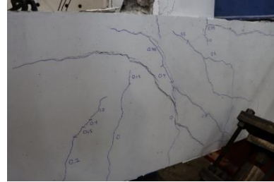
(b) Shear cracks in connection (S-NS-CIP-NH)
