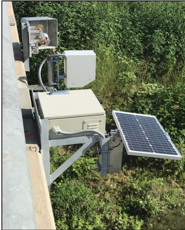
*Figure 2.2 Image of a completed RQ-30 gauge installation. Photograph by Scott Grzyb, U.S. Geological Survey.*
