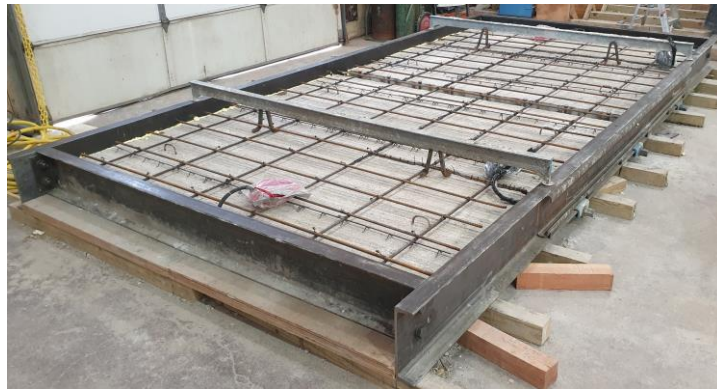
(b) Assembly of reinforcement and steel formwork
