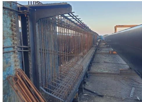
(d-1) Rebar caging for Tx-62
