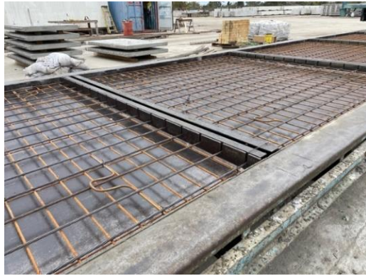
(a) PCP reinforcement
