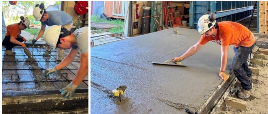
(c) Concrete casting
