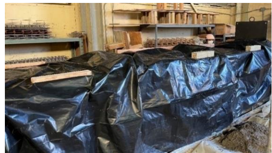
(f) Cure of concrete after casting
