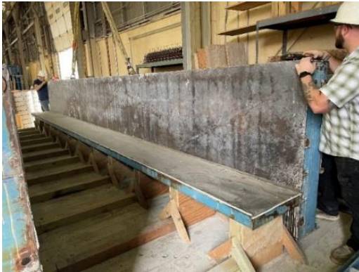
(c) Wood cribbing, soffit, and formwork
