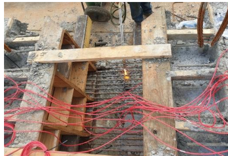
(h) Prestress releasing
