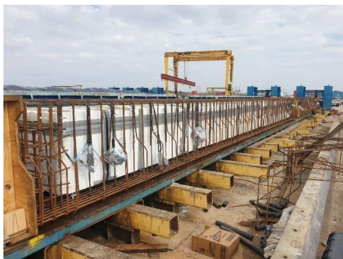
(d-2) Rebar caging for 5B40
