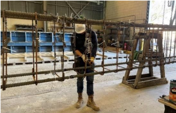
(a) Tying rebar cage
