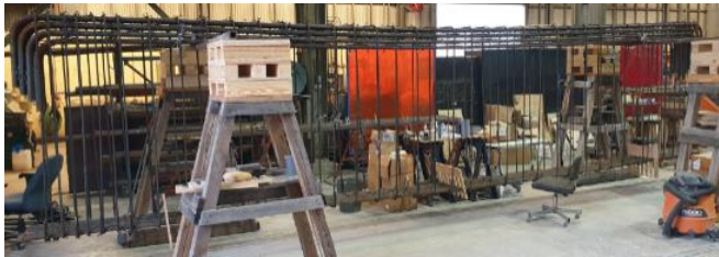
(a) Assembly of rebar cage
