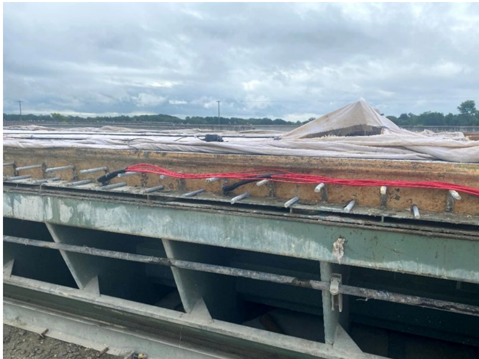
Figure 5.23 NEXT Beam Section RB2-2 After Casting with VWG Wires Exiting Side of Beam and Running along Rebar Located within Future Closure Joint
