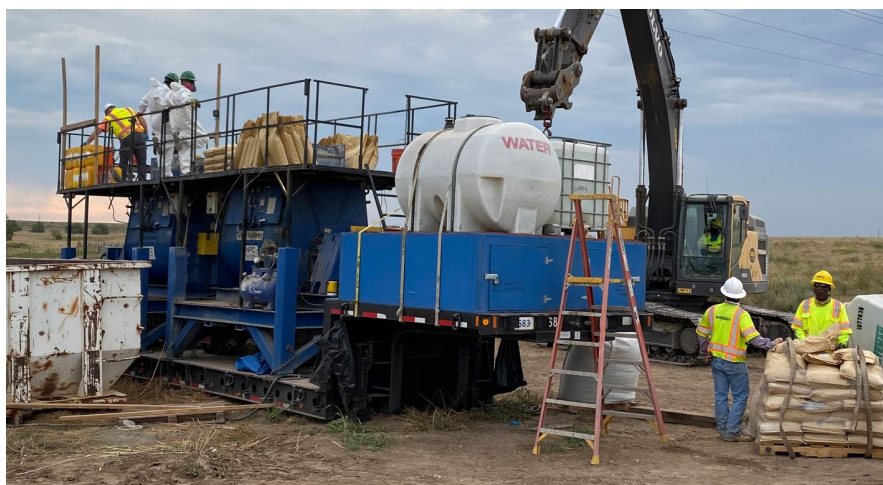
Figure 5.77 Proprietary UHPC Mixer
