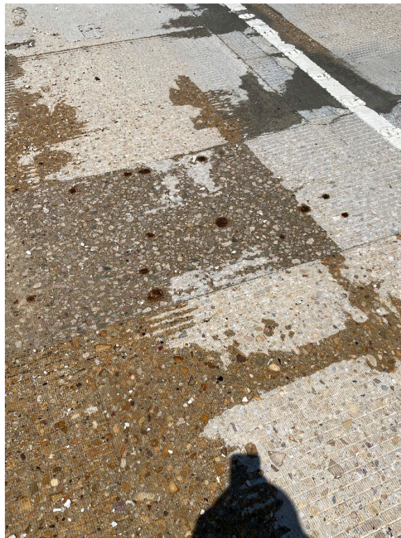
Figure 5.69 Fiber Clumping on Surface of Closure Pours
