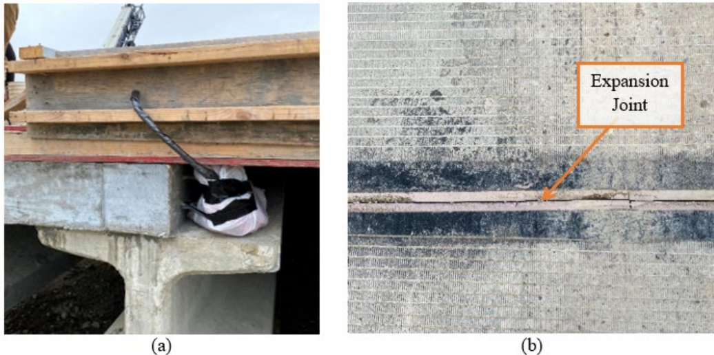
Figure 5.35 Navasota River Bridge Drop-In Deck Panel Lost Gauges. (a) Gauge wires shown exiting front-end of panel near future location of expansion joint; (b) Installed expansion joint.
