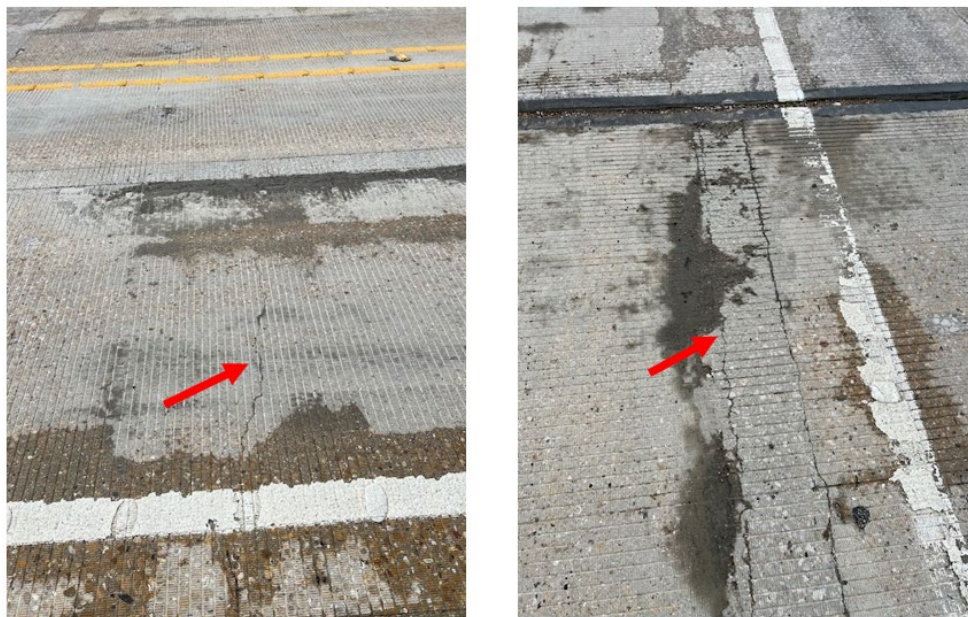
Figure 5.73 Cracking of Bridge Deck
