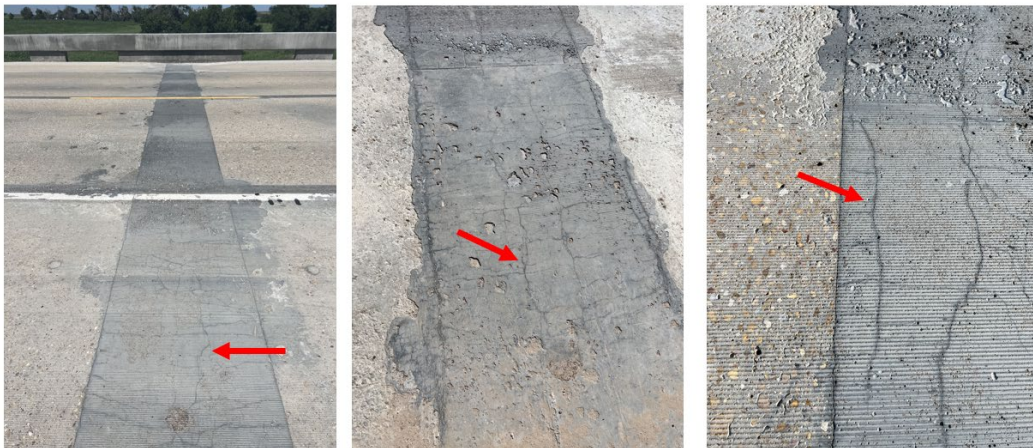
Figure 5.86 Cracking at Transverse Joints
