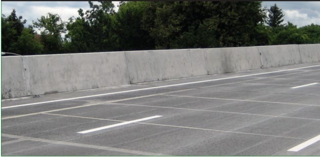
Figure 2.16 Finalized Bridge Deck after UHPC Grinding and Grooving (Graybeal, 2019)
