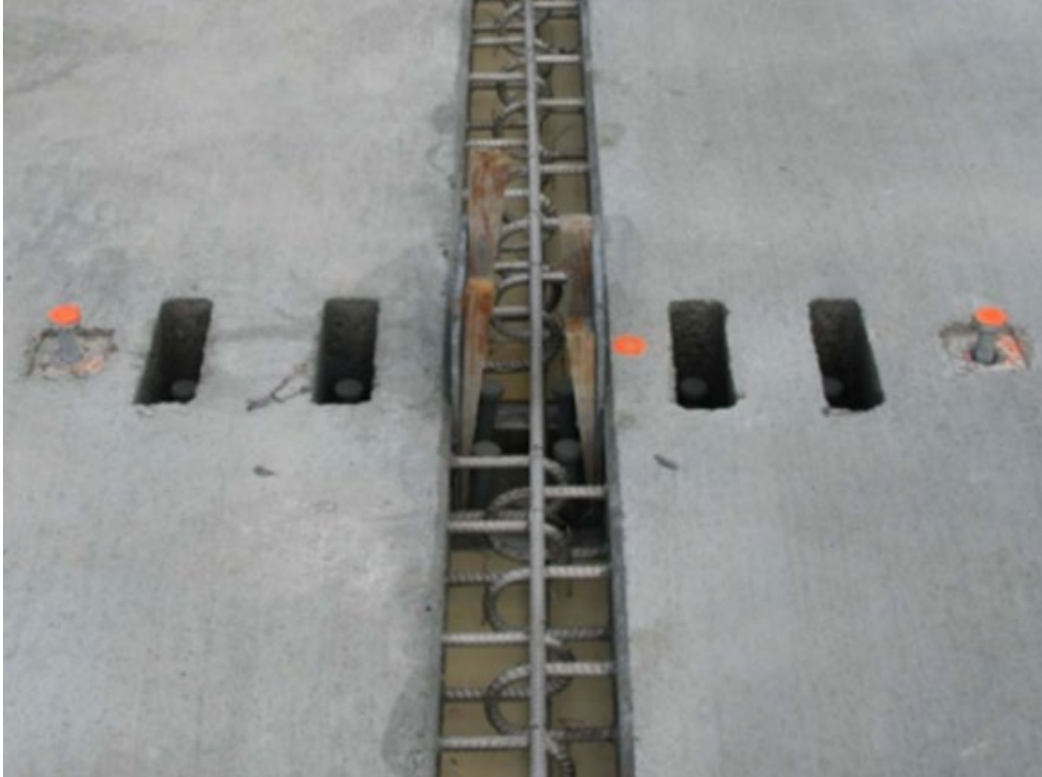
Figure 2.13 Close-Up of Pulaski Skyway Transverse Closure Joint Between Precast Full-Depth Concrete Panels Prior to UHPC Placement (Leidos & WSP, 2018)
