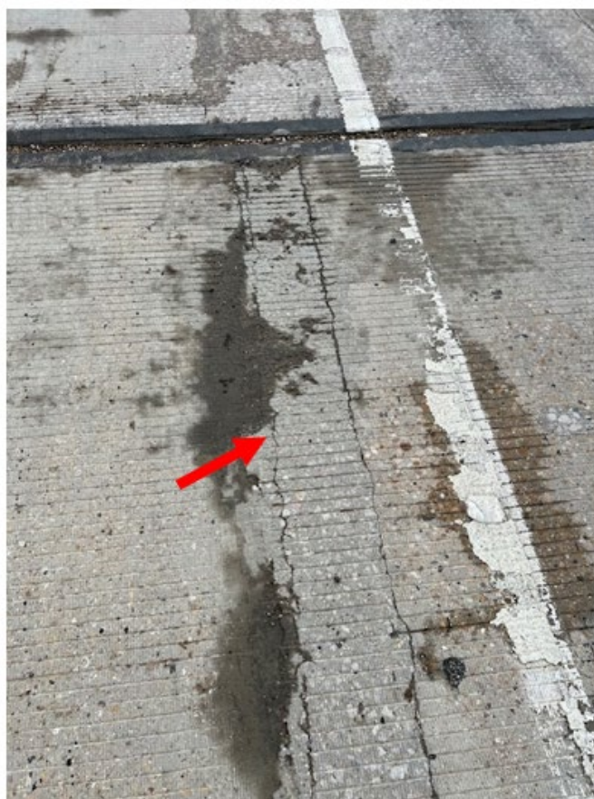
Figure 5.74 Debonding Between Closure Pour and Bridge Decks
