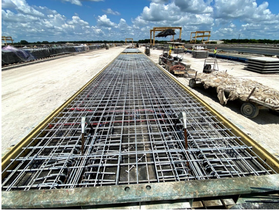
Figure 5.22 Overview of NEXT Beam Section RB2-2 Prior to Casting and After Instrumentation Installed
