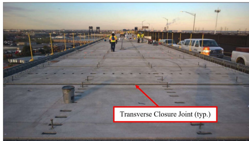
Figure 2.12 Transverse Closure Joints of Pulaski Skyway to be filled with UHPC (Leidos & WSP, 2018)
