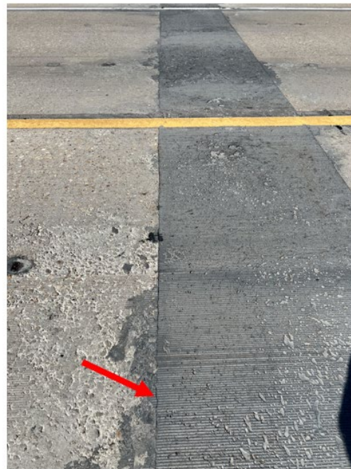
Figure 5.88 Debonding Between Closure Pour and Bridge Deck
