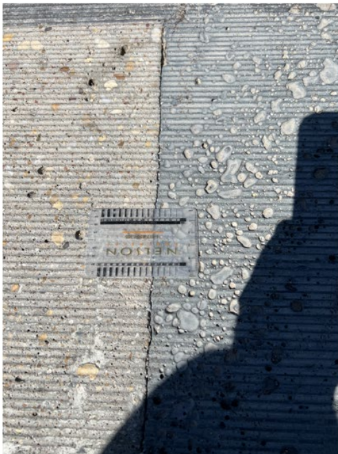
Figure 5.88 Debonding Between Closure Pour and Bridge Deck
