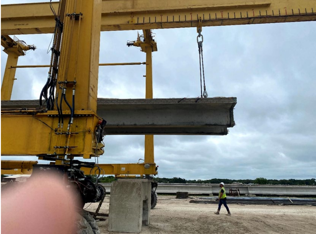
Figure 5.25 NEXT Beam RB2-2 Being Transported to Curing Area
