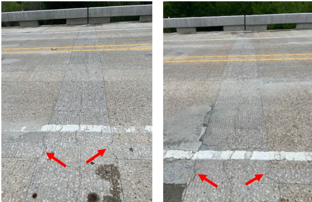
Figure 5.72 Cracking at Interface of Transverse Joint and Bridge Deck
