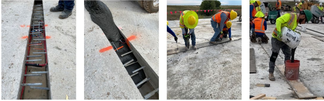
Figure 5.78 Procedure for Placement of Closure Joint
