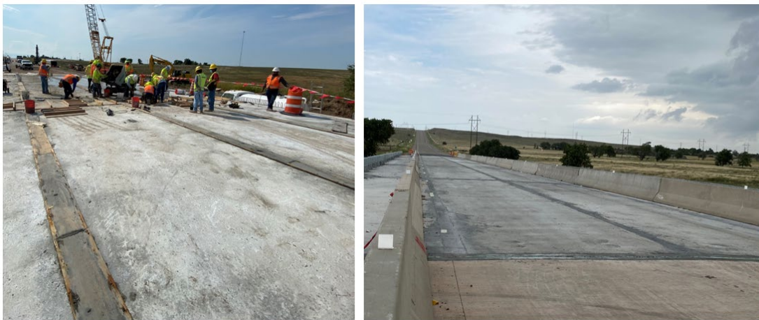
Figure 5.79 Bridge After Placement of Closure Pour
