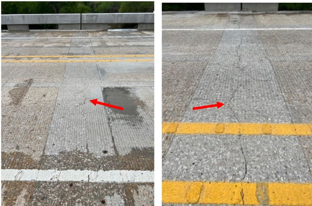
Figure 5.70 Cracking of Transverse Closure Pour
