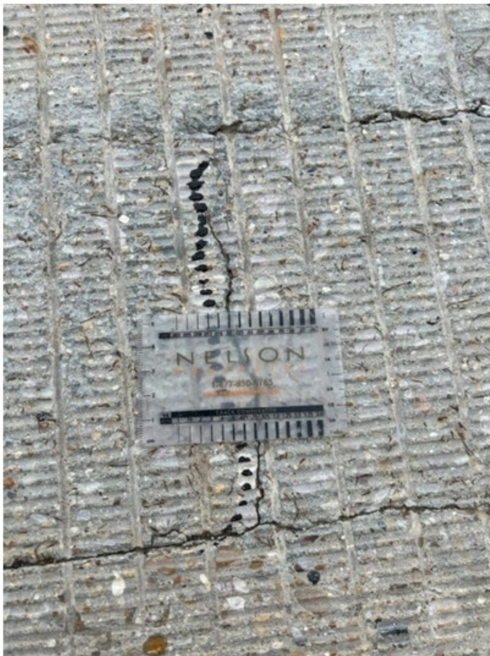
Figure 5.75 Common Crack Found in the Longitudinal Closure Pour
