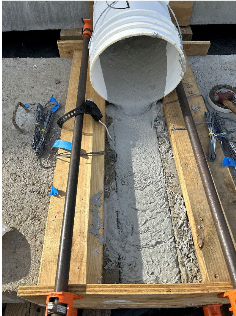
Figure 4.12 UHPC Closure Joint Cast
