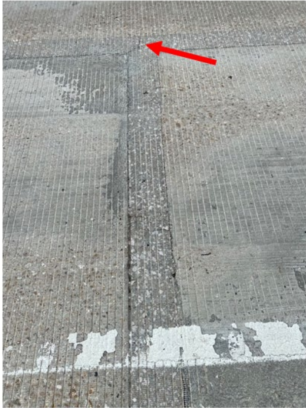
Figure 5.71 Cracking of Longitudinal Closure Pour
