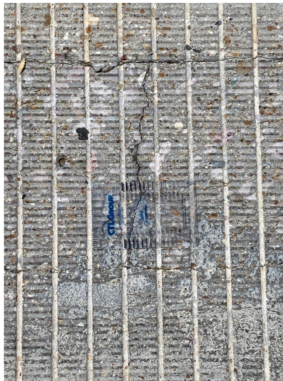
Figure 5.67 Common Crack Found in the Longitudinal Closure Pour
