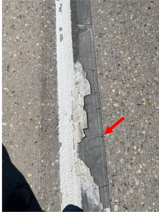
Figure 5.87 Debonding at Longitudinal Joint
