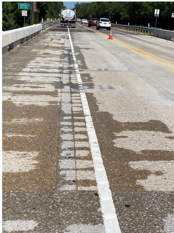
Figure 5.65 Visible Cracks After Pavement Drying
