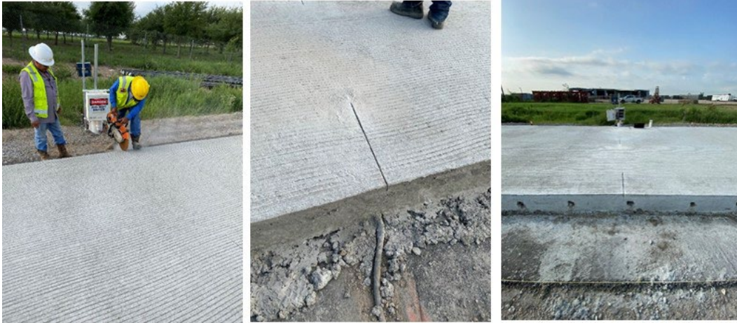
Figure 4.9: Saw cutting of pre-cut joints above vibrating wire gauges at each active monitoring station
