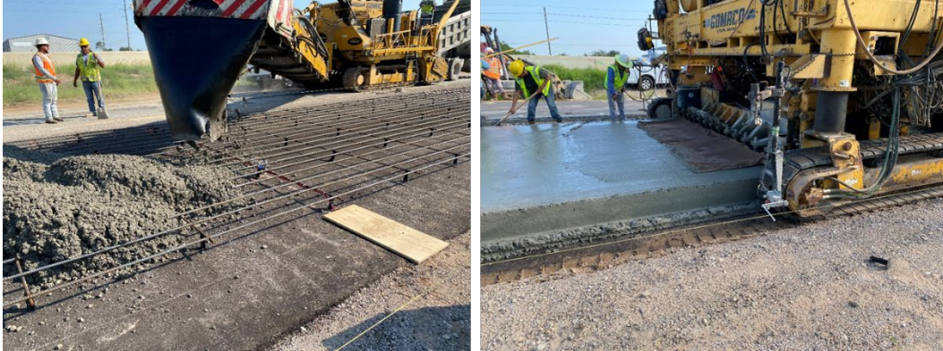
Figure 4.6: Photos showing control mixture being placed, vibrated, and screeded
