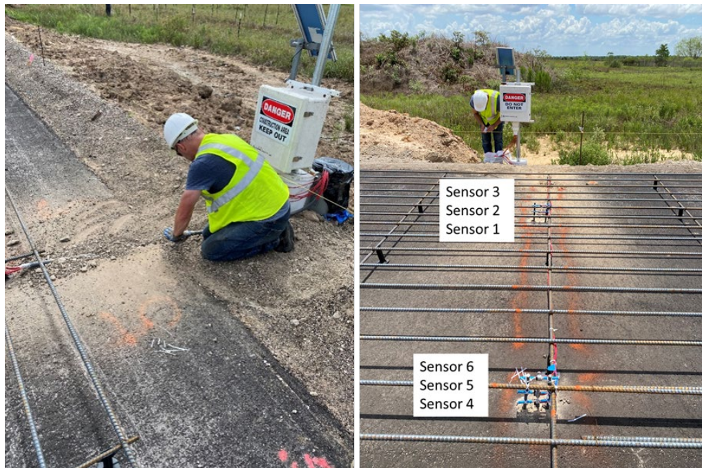
Figure 4.3: Installation of Vibrating Wire Gauges for the measurement of strain and temperature
