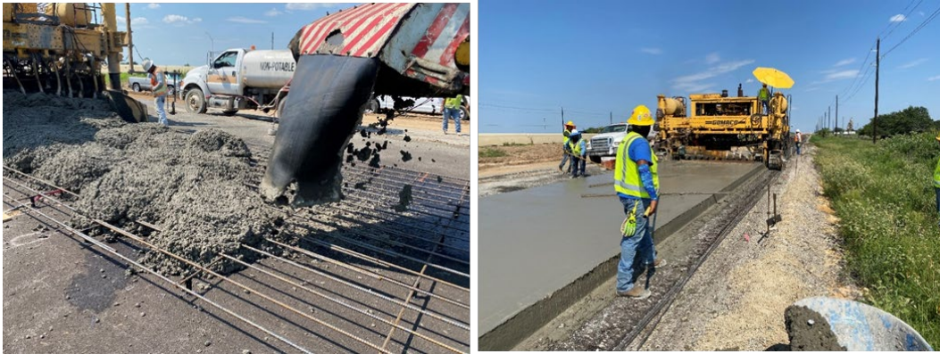
Figure 4.7: Photos showing 50% RCFA mixture being placed, vibrated, and screeded
