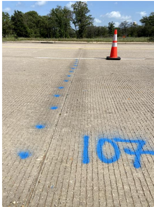
Figure 3.1 Paint Marking along Joint 107 as an Example
