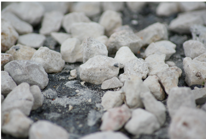
Figure 2.1. Photograph showing excess fines / dust on aggregate particles on a seal coat (emulsion based before rolling)
