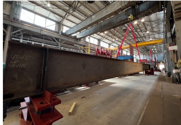
(b) Girder on the supports
