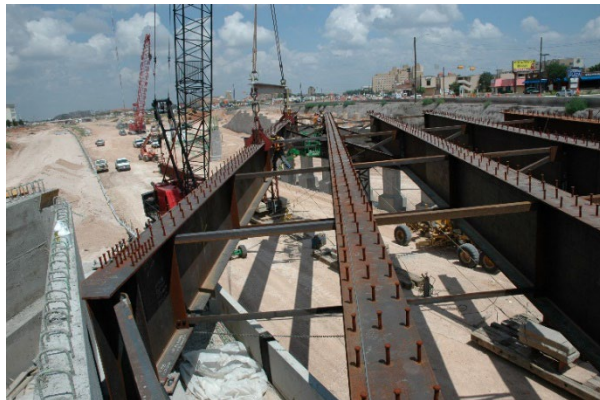
Figure 1.1 - Steel Bridge Girders with Shear Studs
