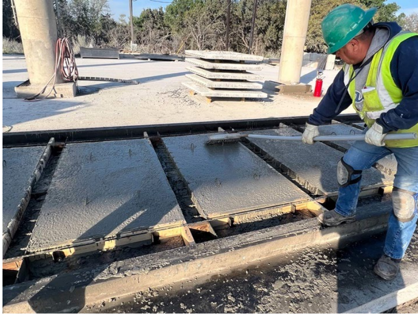
Figure 8.18 – Broom Finishing of Top Surface of PCPs
