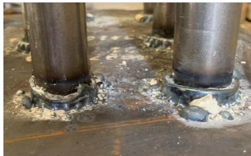
Figure 4.31 - 1" Diameter Shear Stud Welded Without Surface Preparation
