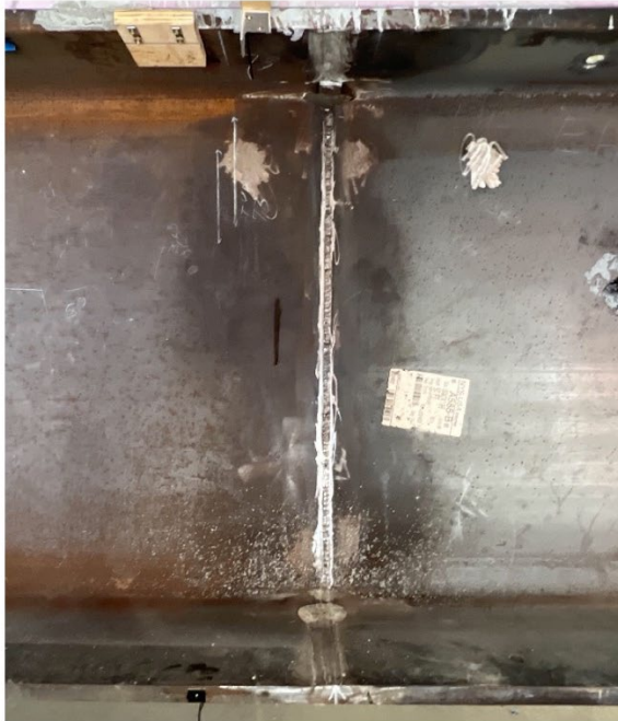
Front view of the splice
