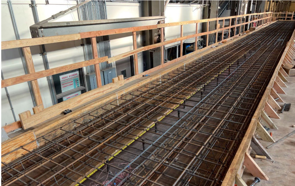
Figure 8.38 – Finished Deck Reinforcement for Beam Specimen No. 1
