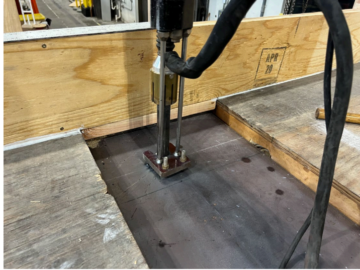
Figure 8.33 – Shear Stud Welding Gun with Stud Installed
