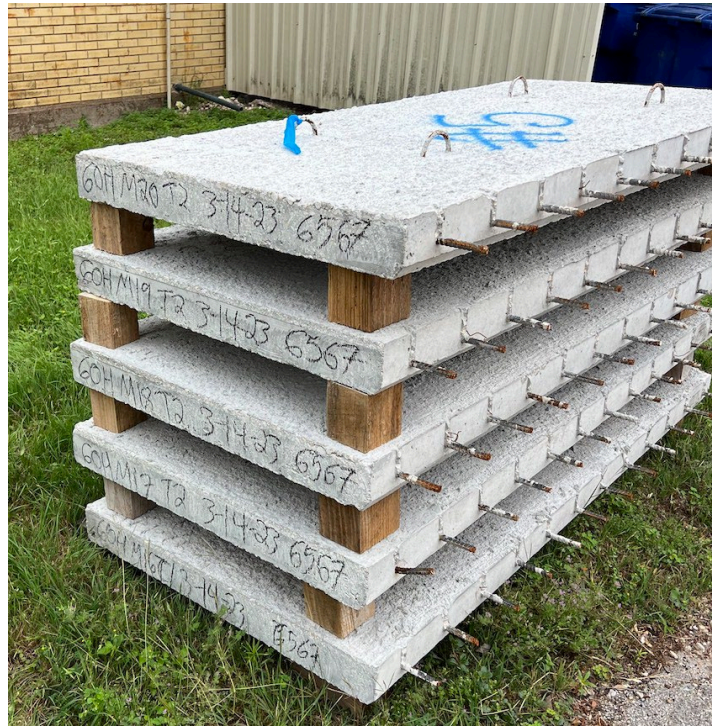
Figure 8.40 – PCP Panels Prior to Placement
