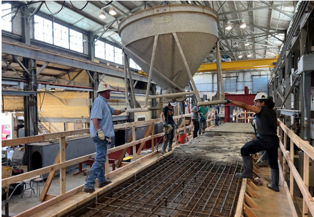
Figure 8.45 – Concrete Placement for Beam Specimen No. 1
