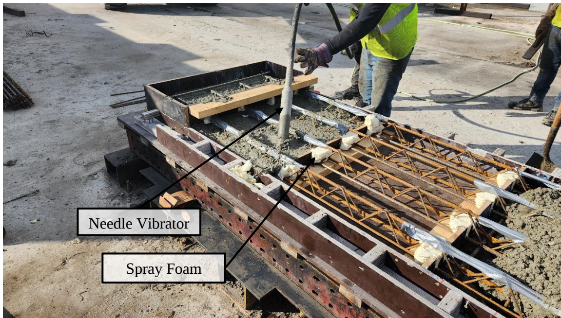
Figure 5-6: Precast Panel Cast
