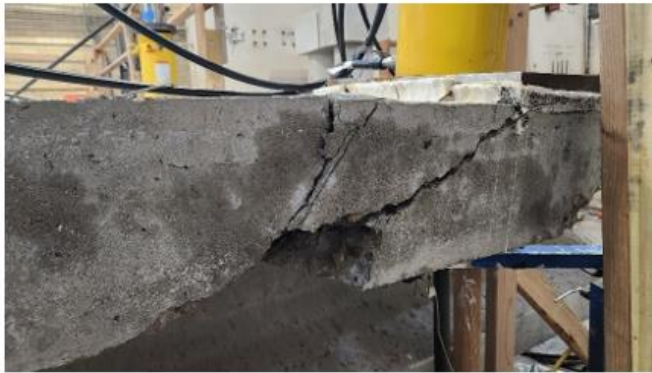
(a) Shear crack from free edge
