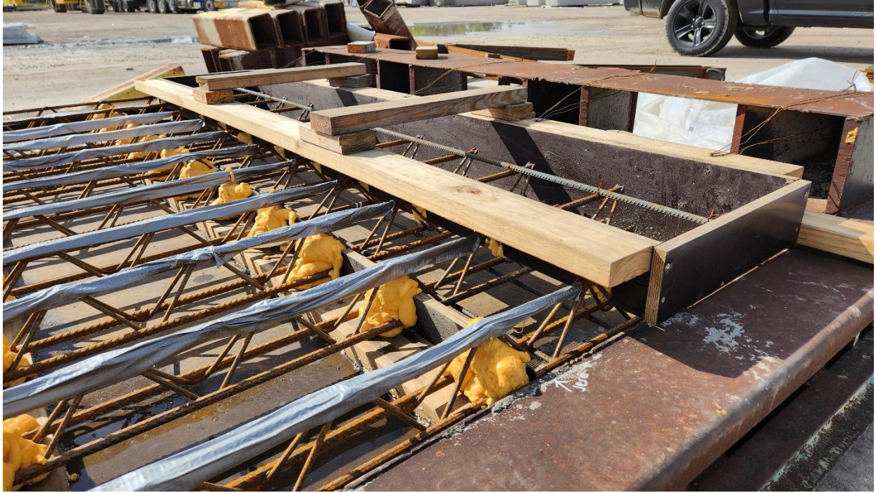
Figure 6-3: Lumber overhang curb formwork
