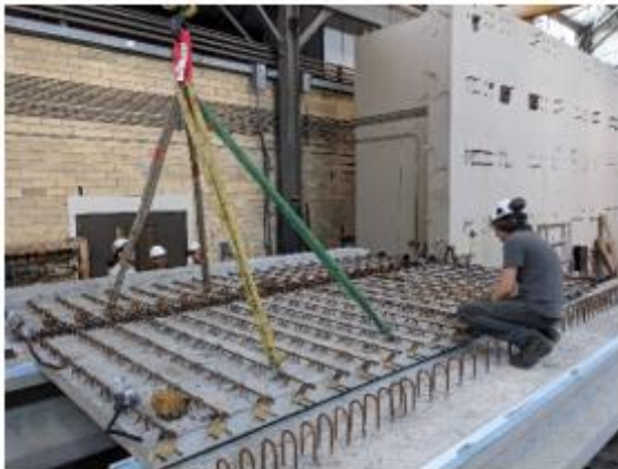
Figure 4-13: Placement of panel pairs
