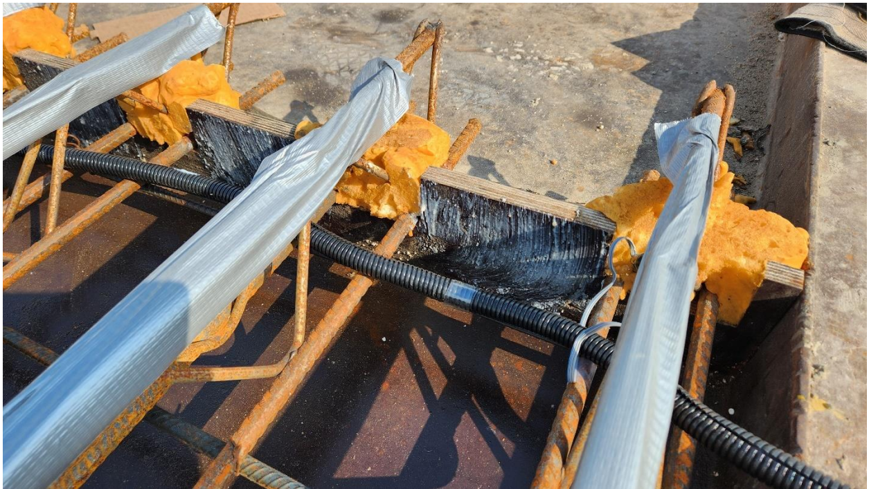
Figure 6-4: Lumber end form and spray foam
