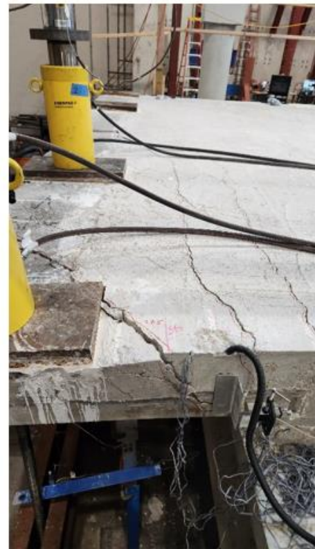
(c) Shear crack from top view
