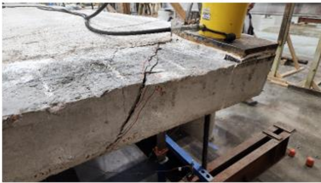
(a) Shear crack from free edge
