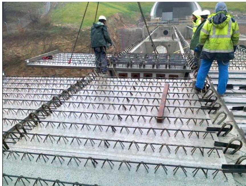
Figure 2-9 Lattice girders continuous over the fascia girder (a)courtesy of Roads and Bridges LLC, (b) courtesy of Dr. David Fernández-Ordóñez
