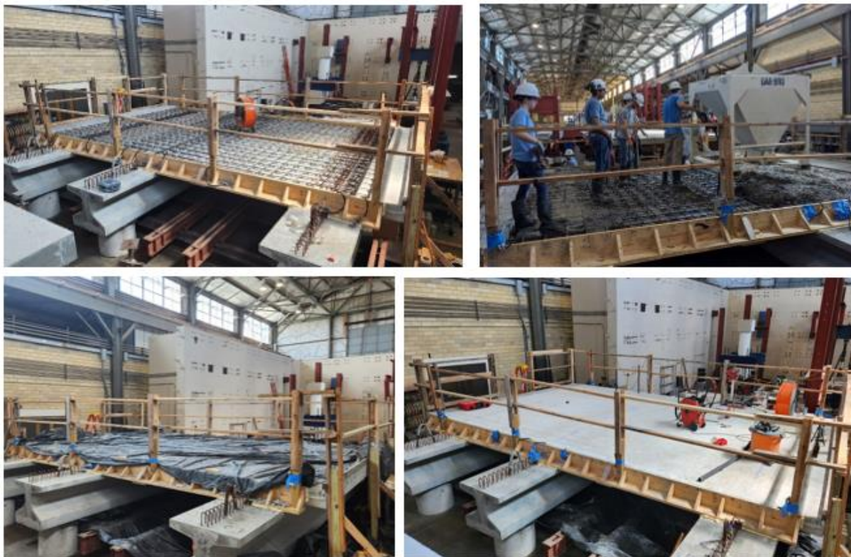
Figure 4-15: Casting and finished WTPD deck specimen
