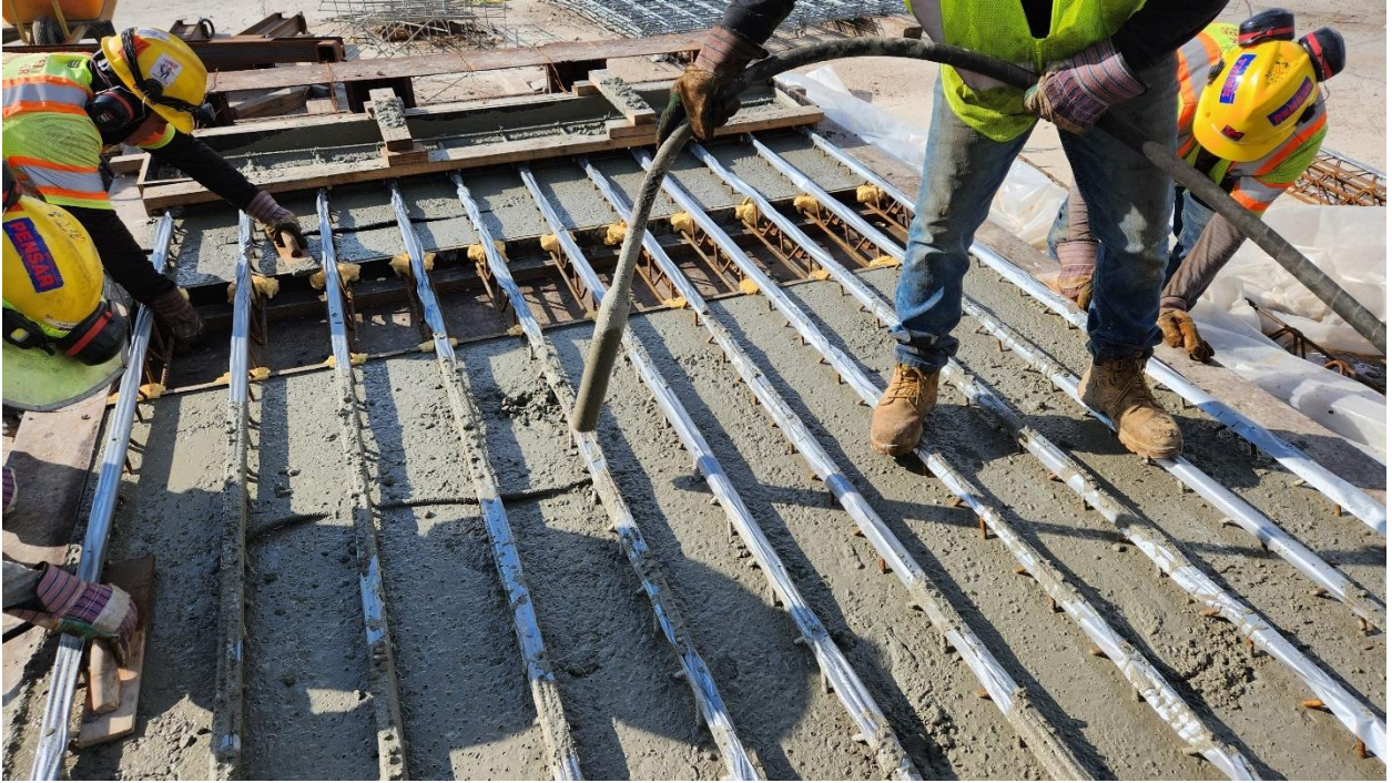
Figure 6-2: Finishing and troweling
