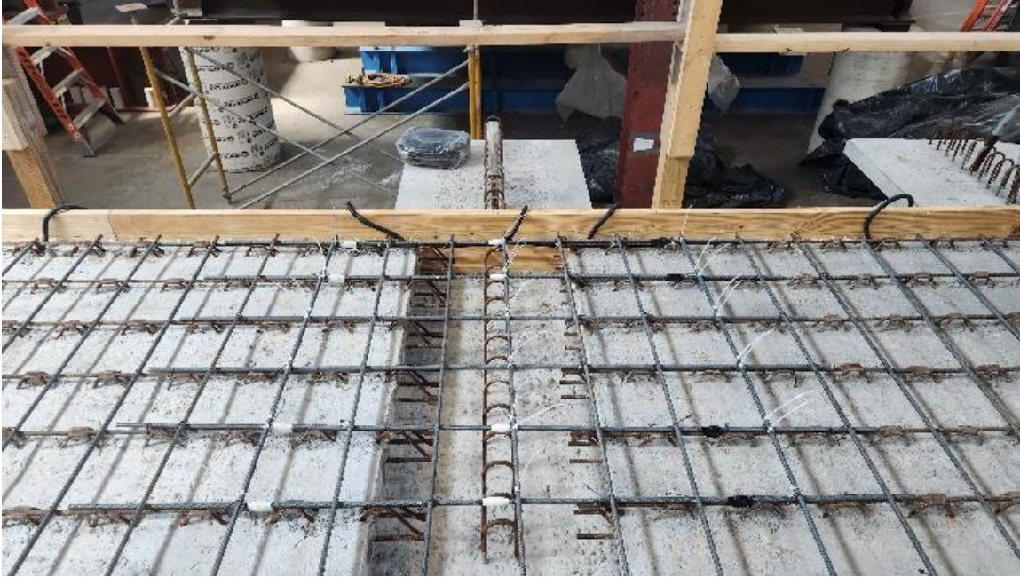
Figure 4-14: Reinforcement and lap-splice
