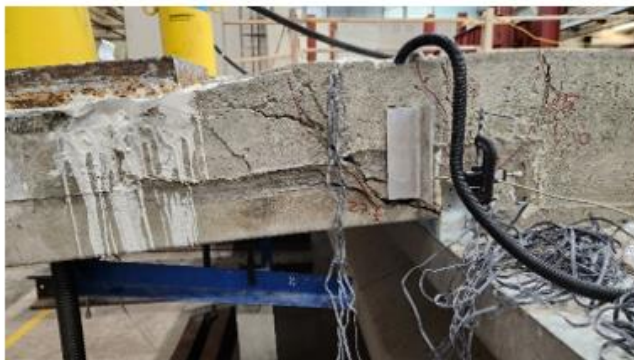
(b) Shear crack from transverse joint
