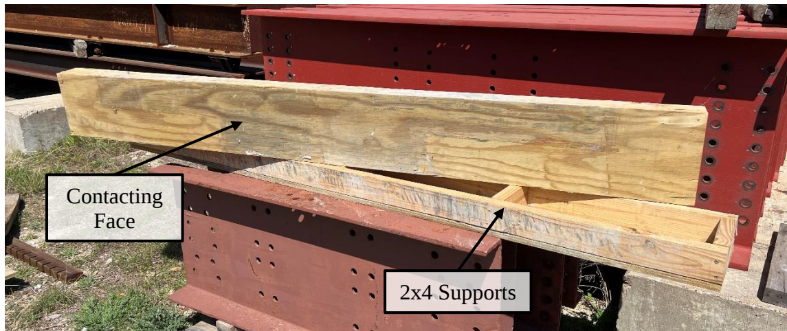
Figure 5-7: Wooden Formwork
