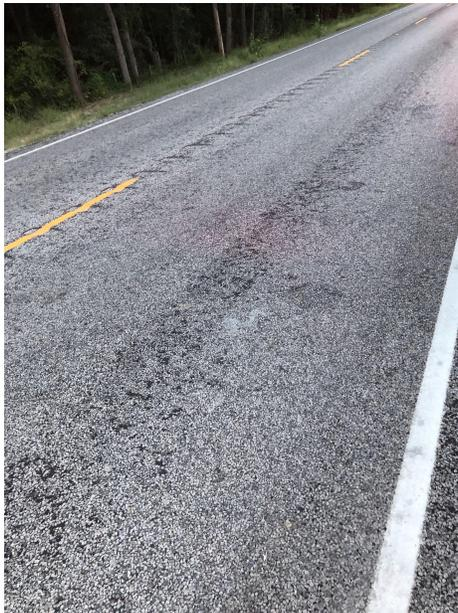
**Figure 4.39. Site Visit Picture of Type D mixture Section 40 (2) (the pavement surface being investigated appears to have an overlay/chip seal and is 4 years old).**
