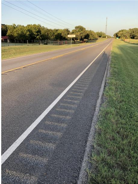
**Figure 4.31. Site Visit Picture of Type D mixture Section 47 (1) (the pavement surface being investigated appears to have an overlay/chip seal and is 4 years old).**
