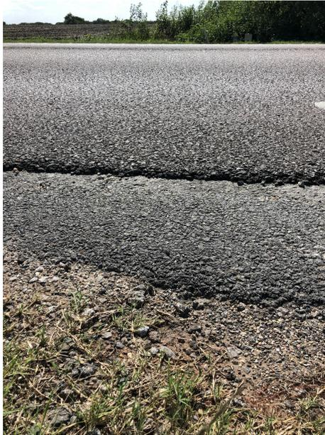
**Figure 4.28. Site Visit Picture of Type C mixture Section 14 (2) (the pavement surface being investigated appears to have an overlay/chip seal and is 3 years old).**
