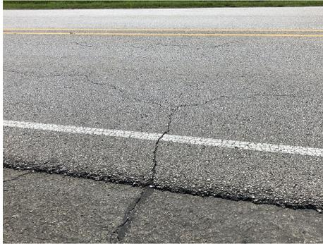
**Figure 4.18. Site Visit Picture of Type C mixture Section 29 (2) (the pavement surface being investigated appears to have an overlay/chip seal and is 5 years old).**
