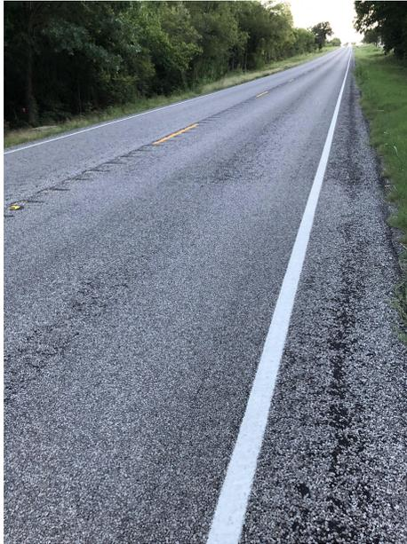
**Figure 4.38. Site Visit Picture of Type D mixture Section 40 (1) (the pavement surface being investigated appears to have an overlay/chip seal and is 4 years old).**
