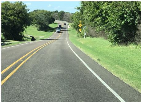
**Figure 4.29. Site Visit Picture of Type C mixture Section 14 (3) (the pavement surface being investigated appears to have an overlay/chip seal and is 3 years old).**
