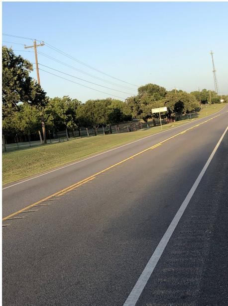
**Figure 4.32. Site Visit Picture of Type D mixture Section 47 (2) (the pavement surface being investigated appears to have an overlay/chip seal and is 4 years old).**
