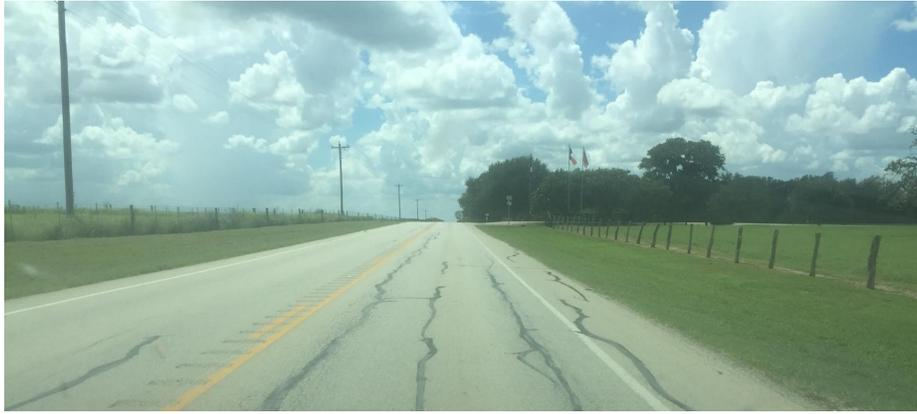
**Figure 4.36. Site Visit Picture of Type D mixture Section 4 with longitudinal cracks.**
