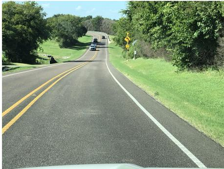
**Figure 4.27. Site Visit Picture of Type C mixture Section 14 (1) (the pavement surface being investigated appears to have an overlay/chip seal and is 3 years old).**
