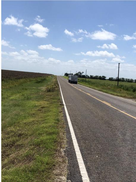
**Figure 4.22. Site Visit Picture of Type C mixture Section 18 (2) (the pavement surface being investigated appears to have an overlay/chip seal and is 11 years old).**
