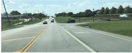
**Figure 4.17. Site Visit Picture of Type C mixture Section 29 (1) (the pavement surface being investigated appears to have an overlay/chip seal and is 5 years old).**
