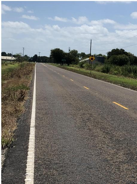
**Figure 4.21. Site Visit Picture of Type C mixture Section 18 (1) (the pavement surface being investigated appears to have an overlay/chip seal and is 11 years old).**
