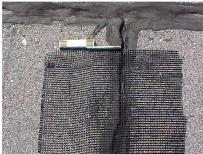
*Figure 2.20. Photograph showing close-up of glass grid installed on a transverse crack (ME 01-3).*
