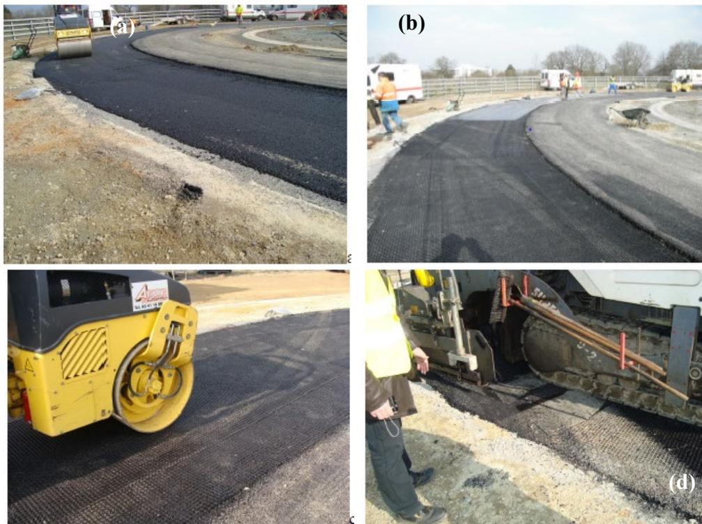
Figure 2.27. Photographs showing: (a) construction of 20-mm-thick bituminous layer; (b) fiberglass grid installation; (c) compaction of grid; and (d) paving of 50-mm-thick bituminous layer (IFSTTAR, 2012).
