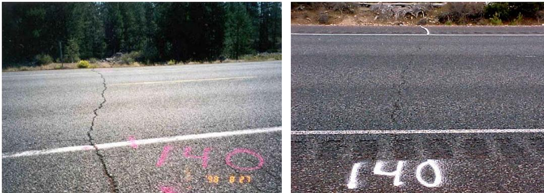
*Figure 2.23. Photographic comparison of crack 140 before overlay construction (left) and reflection of crack through overlay after construction (right) (OR-RD-08-01).*
