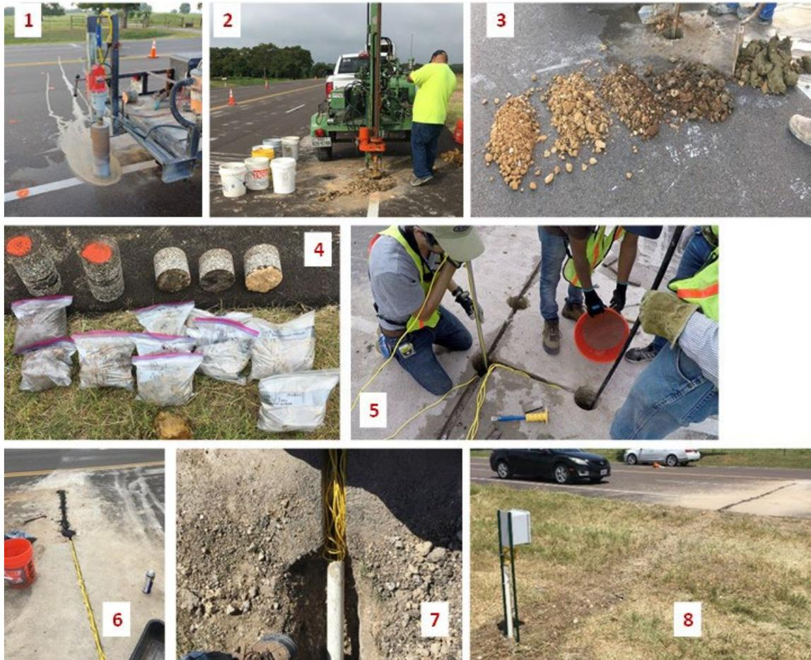
Figure 5.15. Photographs summarizing sequence of moisture sensor installation.
