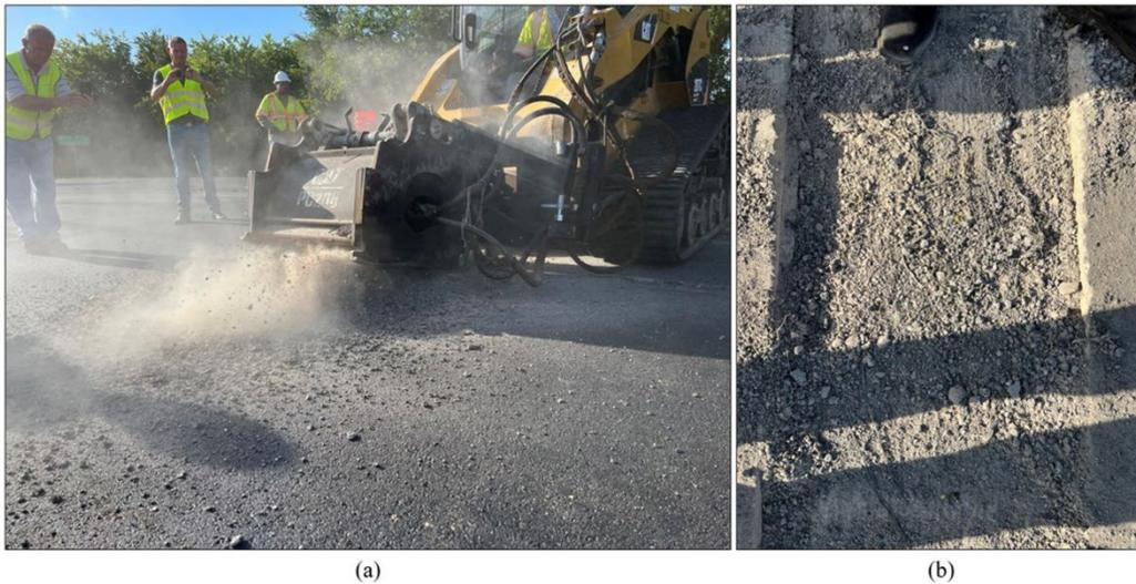
Figure 9.14. Milling of asphalt layer that had polyester (PET) geogrid: (a) milling operation performed at site; and (b) presence of PET geogrid fibers at the site.
