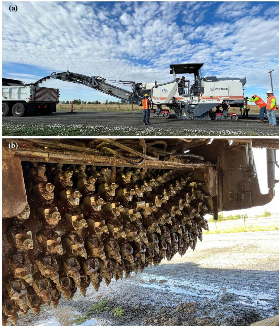
Figure 9.2. Milling operation to collect RAP and GRAP samples: (a) view of equipment during operations; and (b) detail of milling drum.
