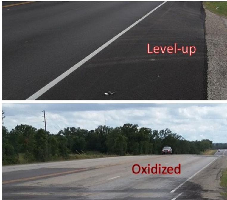
Figure 3.8. Asphalt surface condition: (a) level-up; and (b) oxidized.
