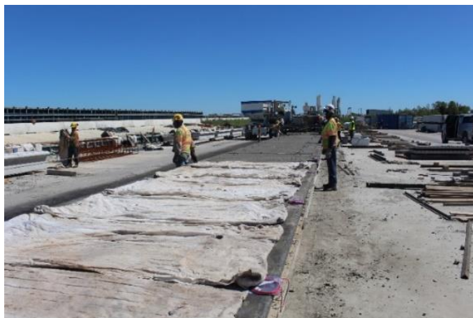
Figure 4.5 Concrete panel curing
