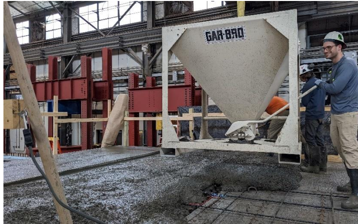
Figure 6.3 Concrete casting procedure
