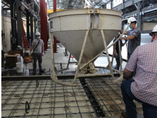
Figure 4.7 Concrete casting using concrete bucket
