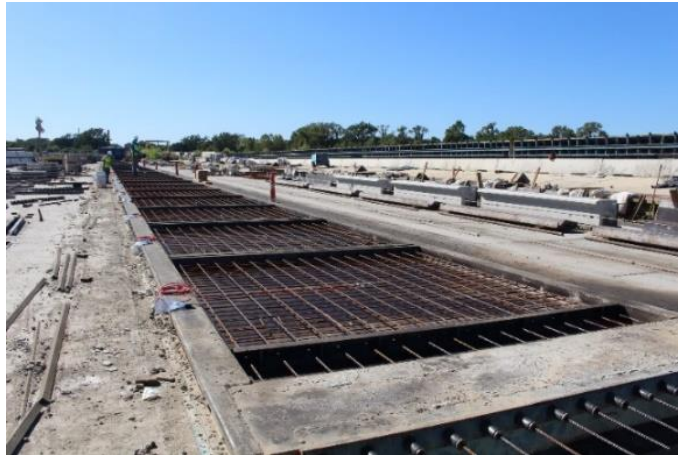
Figure 4.3 Precast panels before concrete casting
