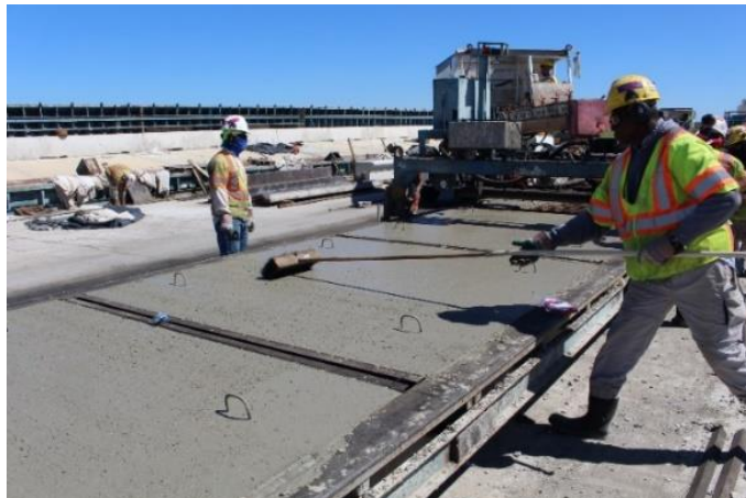
Figure 4.4 Roughened panel surface using brooms
