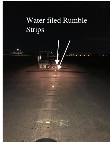
Visibility of water-filled rumble inserts (100 ft)
