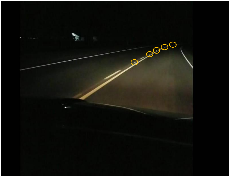
Figure 6-15 Qualitative visibility of RPMs in Location 2 (SL 335, Amarillo District), illuminated markers circled
