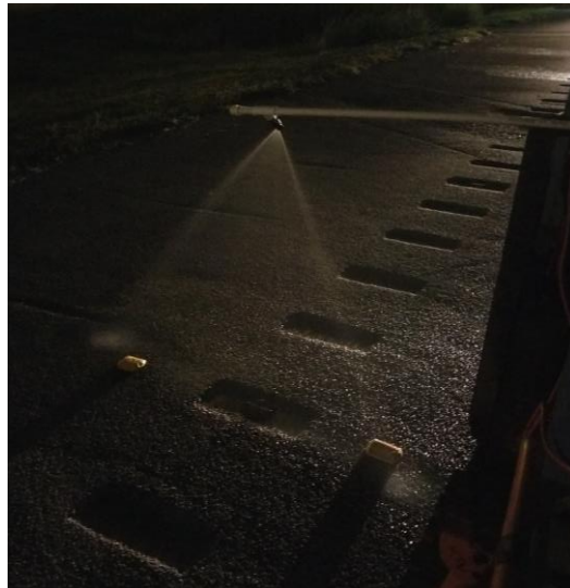
Figure 6-18 Water spraying on an RPM installed in rumble strip using the rain simulator
