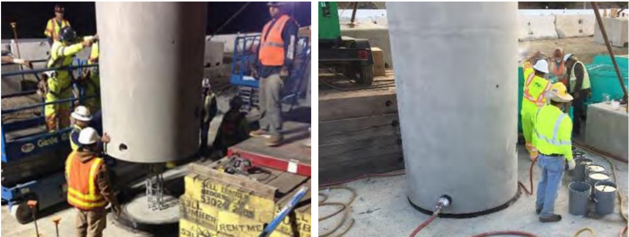
Figure 2-42: Erection of precast column in Laurel Street Overcrossing (Mellon 2018)
