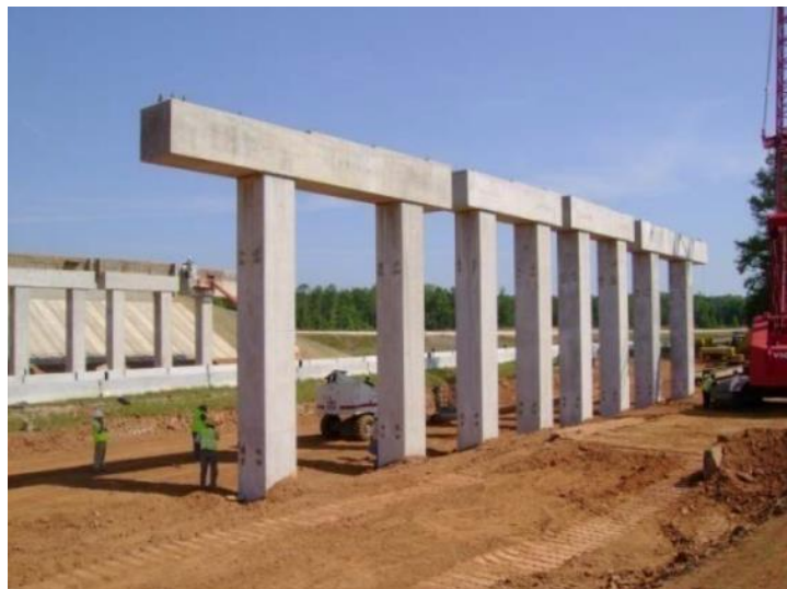
Figure 2-50: Precast columns and pier caps in the IH-85 Interchange project (Mallela et al. 2013)
