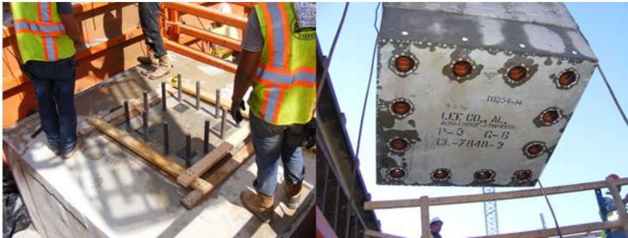
Figure 2-38: Connection bars in footing (left) and coupler in column (right) in Moore's Mill Road Bridge (City of Auburn 2019)
