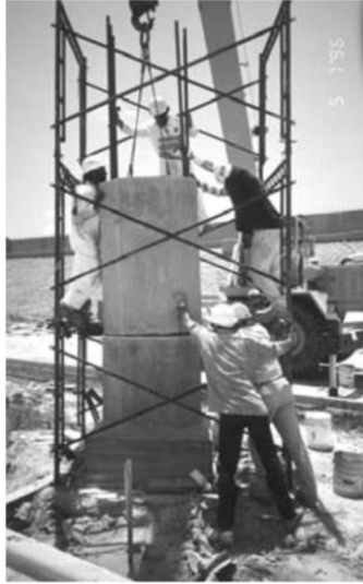
(b) example of precast segmental column
