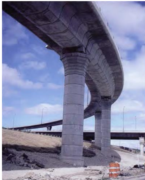
Figure 2-71: Completed US 183 Elevated Highway (Billington et al. 1998)
