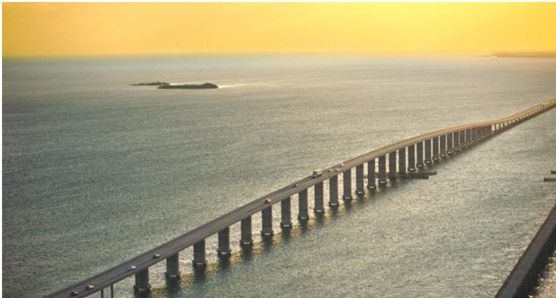
Figure 2-45: Seven Mile Bridge after construction (FIGG Bridge Group- www.figgbridge.com )
