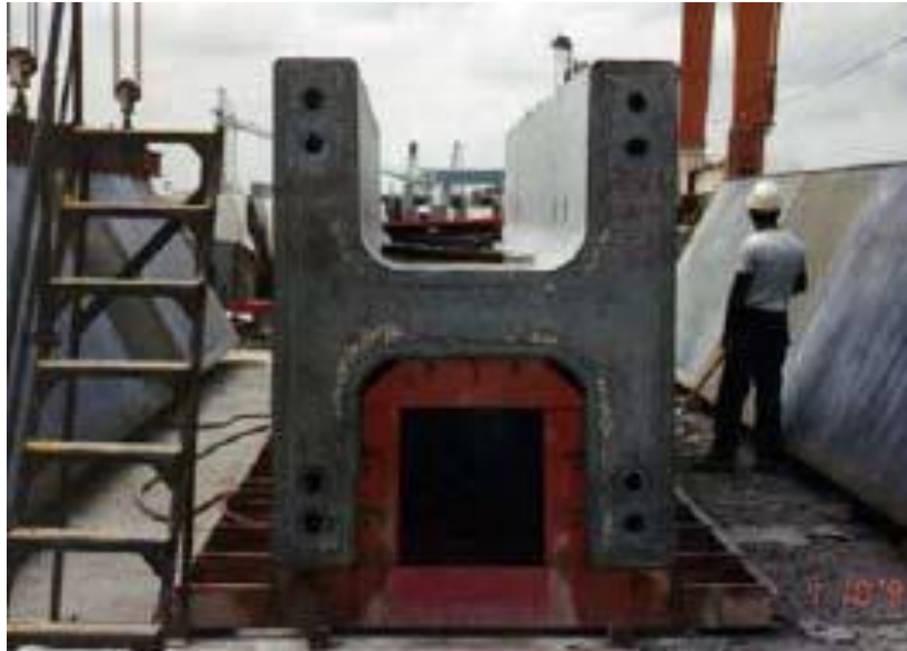
Figure 2-46: H-shaped precast Concrete Column used in Edison Bridge (FHWA 2009)
