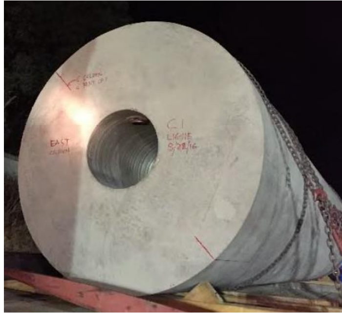
Figure 2-41: Precast column in Laurel Street Overcrossing (Mellon 2018)
