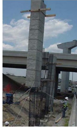
(c) example of precast column shell
