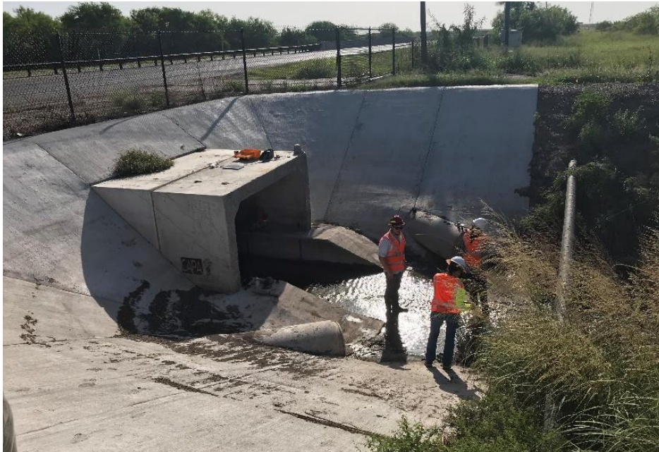
Figure 3.2. FM 106 wildlife crossing box culvert with ledges and ramps, which facilitate animal use of structure. Photo Courtesy of L. Loftus-Otway
