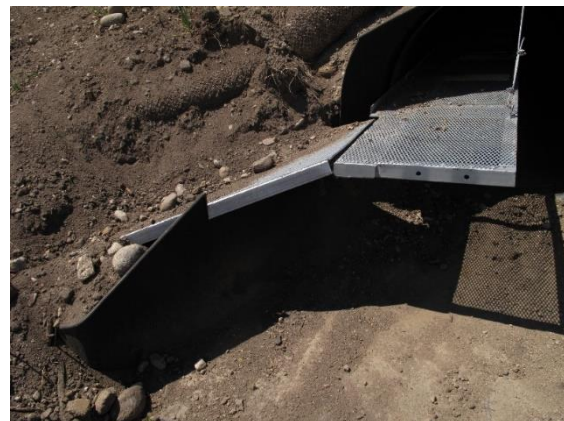
Figure 4.4. Left: Minnesota DOT wildlife path created in rip rap; Right: Montana DOT wildlife shelf and an entrance ramp for smaller wildlife. Photos courtesy of P. Cramer.
