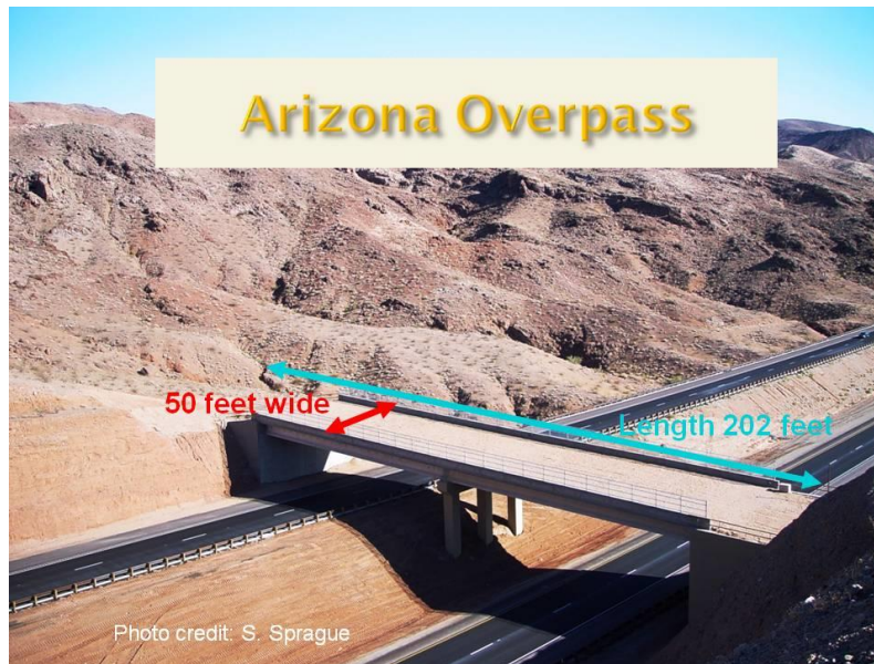
Figure 4.3. Desert bighorn sheep overpass on US 93 in Arizona. Photo courtesy of S. Sprague, Arizona Game and Fish Department.
