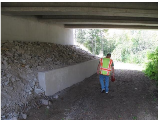
Figure 4.4. Left: Minnesota DOT wildlife path created in rip rap; Right: Montana DOT wildlife shelf and an entrance ramp for smaller wildlife. Photos courtesy of P. Cramer.
