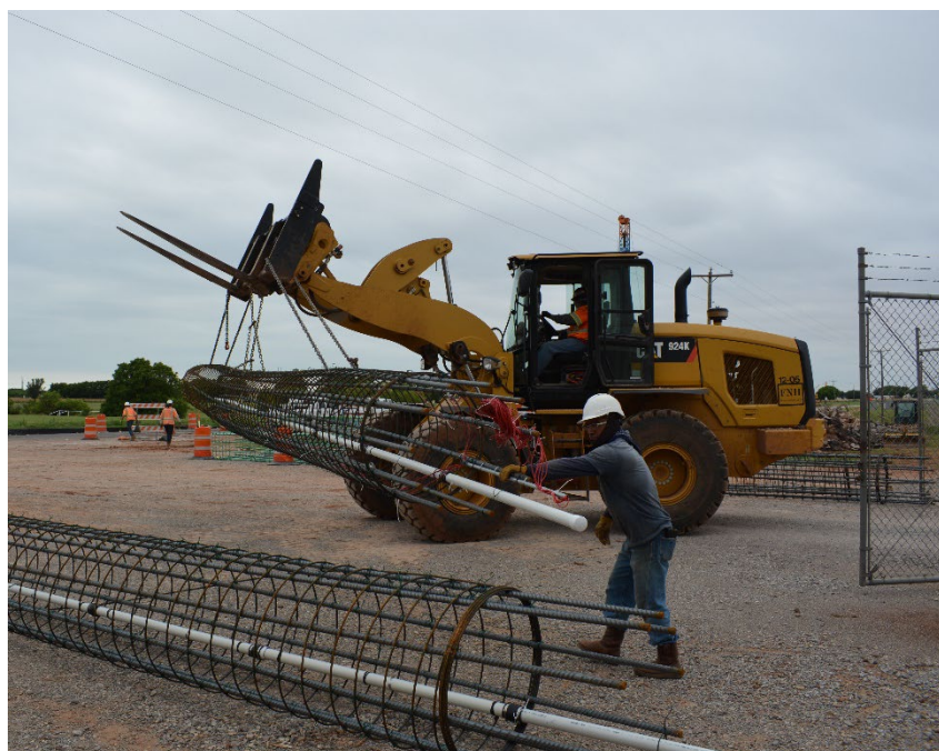
Figure 8.60: Instrumented rebar cage intended for China Creek Bridge east-center drilled shaft, phase 2
