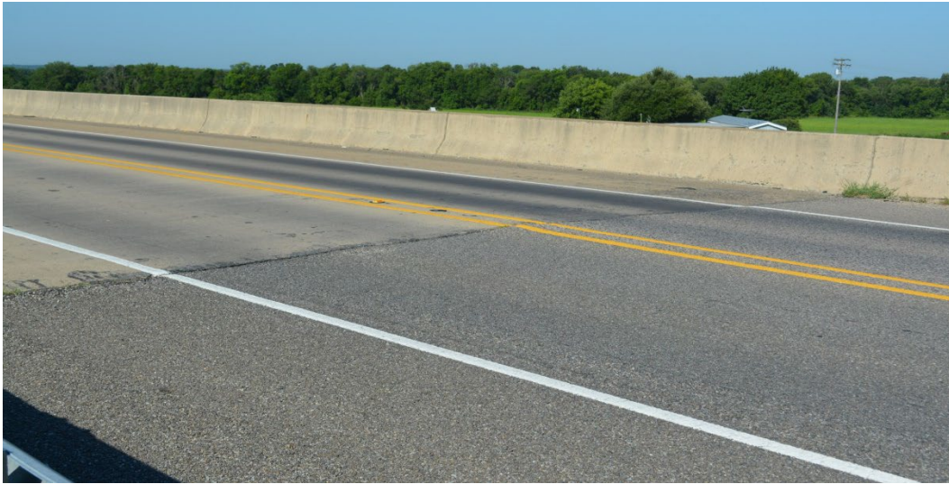
Figure 2.5: Fannin County SIAB roadway-to-bridge-deck transition (from north end looking southwest)
