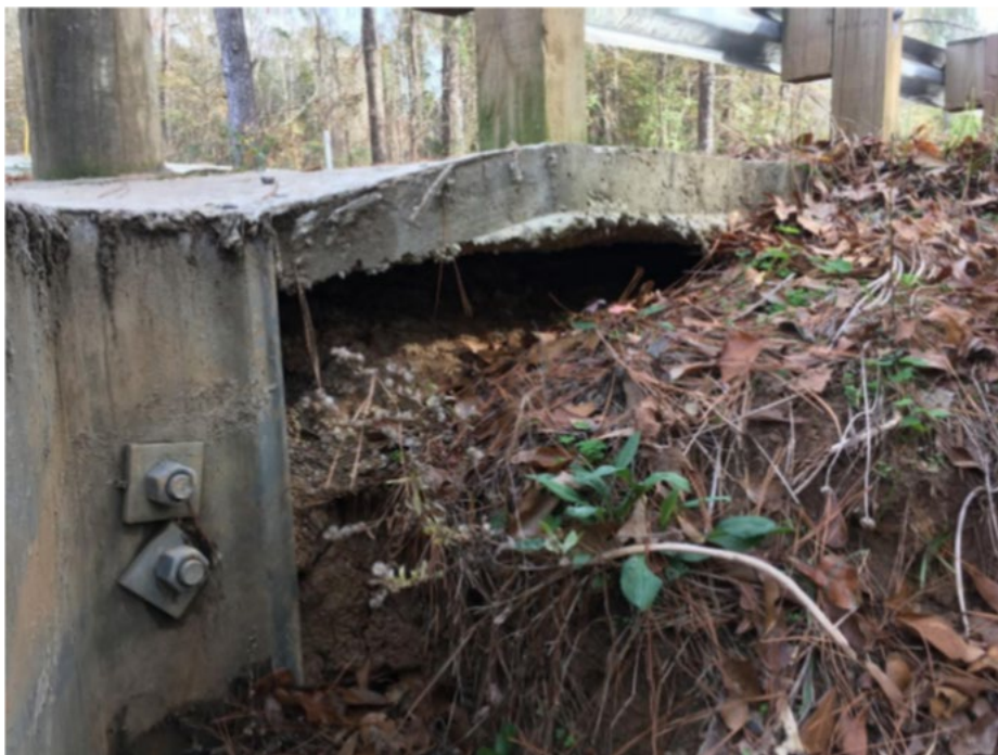
Figure 4.21: Void caused by erosion of fill under shoulder of southern approach
