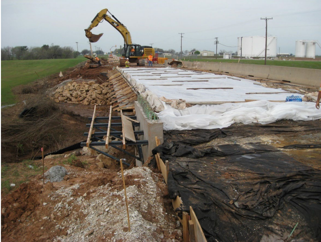
Figure 8.53: Covered deck surface after concrete placement, phase I, March 2020
