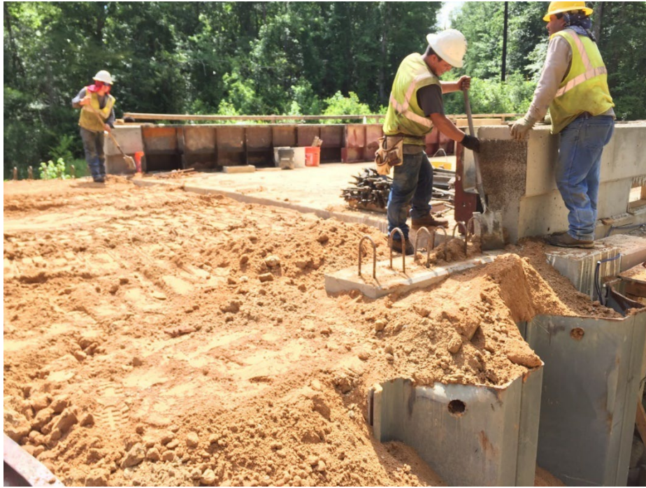
Figure 11.3: Sandy/clayey soil excavated from the site was used as base material for the approach roadway
