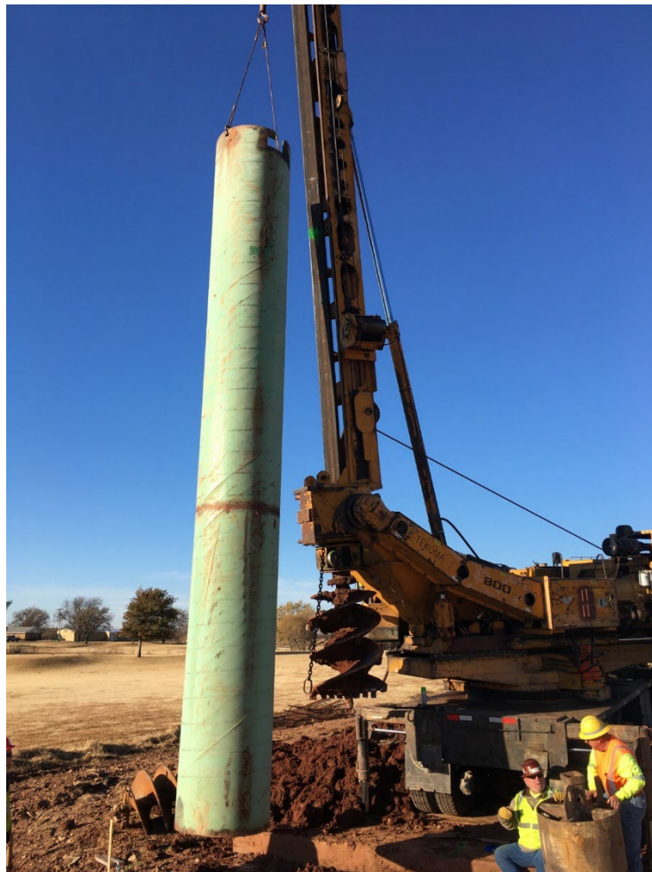
Figure 8.38: Casing used for top 20 ft of drilled shafts
