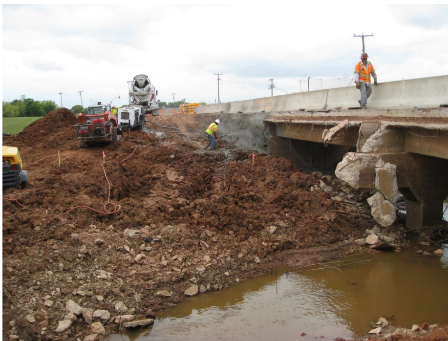
Figure 8.35: Installation of soil nail wall as temporary support for active roadway crossing the undemolished half of China Creek Bridge (Picture provided by Samuel Groves)
