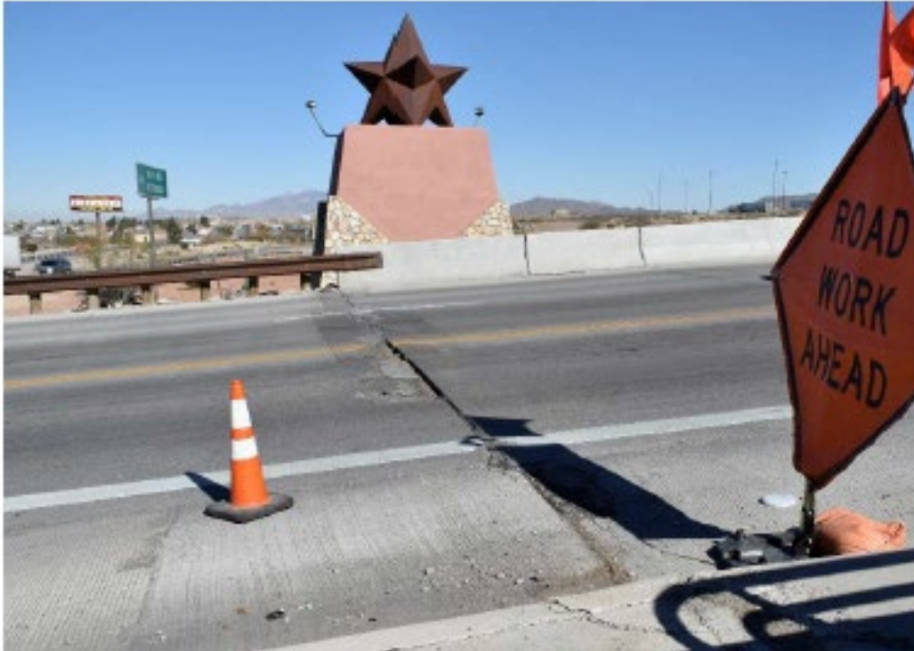
Figure 4.8: Photograph of west transition from approach road (left) to approach slab (right) on Anthony IAB
