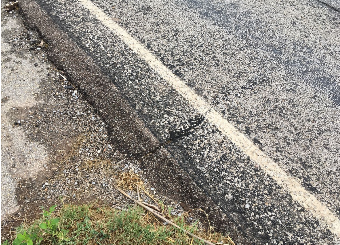
Figure 8.5: Cracked edge of pavement at end of the approach slab due to backfill settlement
