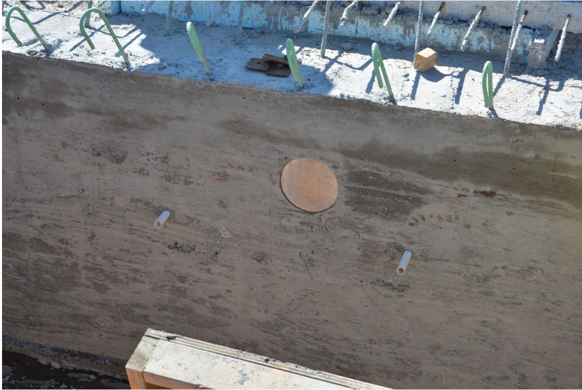
Figure 8.45: Finished surface of east abutment backwall with pressure cell (GK-4810) installed between two girders on left, March 2020
