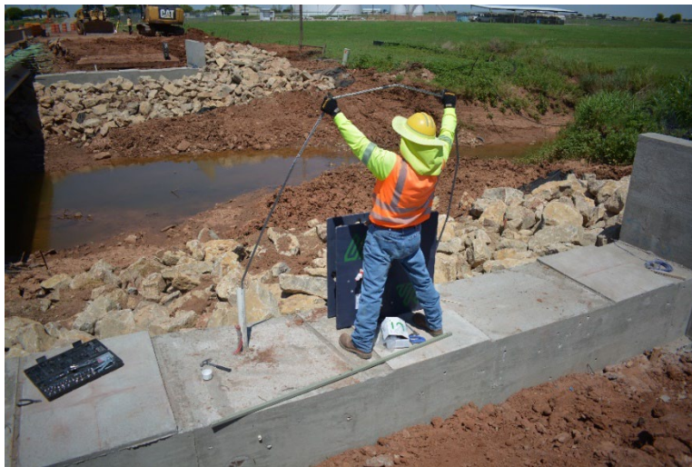
Figure 8.67: SAAV installation in east abutment center drilled shaft
