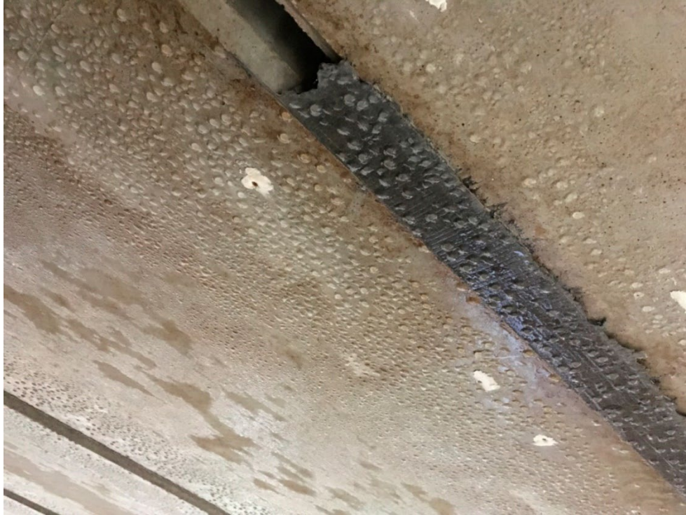
Figure 4.18: Water droplets gathered underneath the girders
