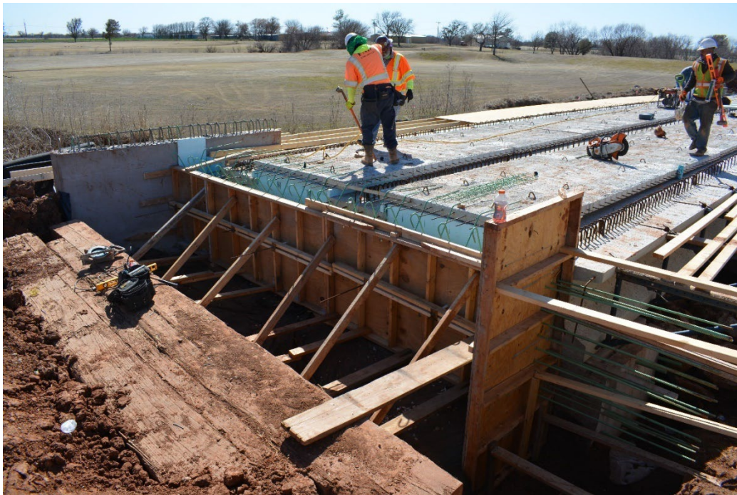
Figure 8.43: Forming of abutment backwalls after placement of girders and precast panels, March 2020 (east abutment)
