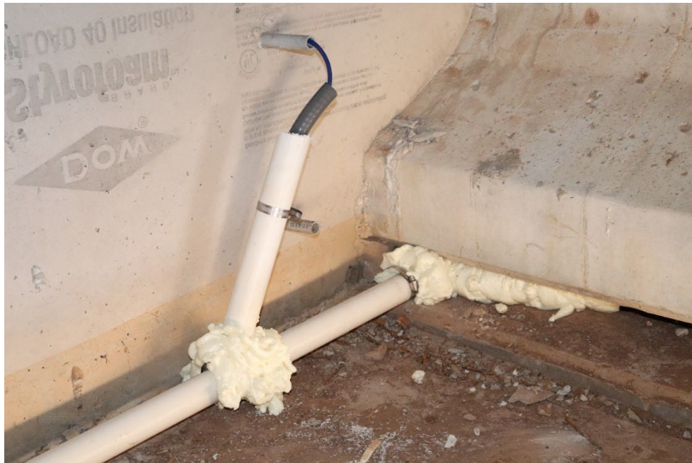
Figure 8.92: PVC pipes to protect cables routed on top of abutment caps
