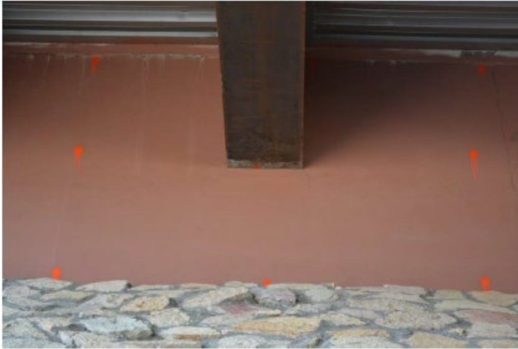
Figure 4.4: Photograph of survey points (orange dots) on Anthony IAB east abutment face
