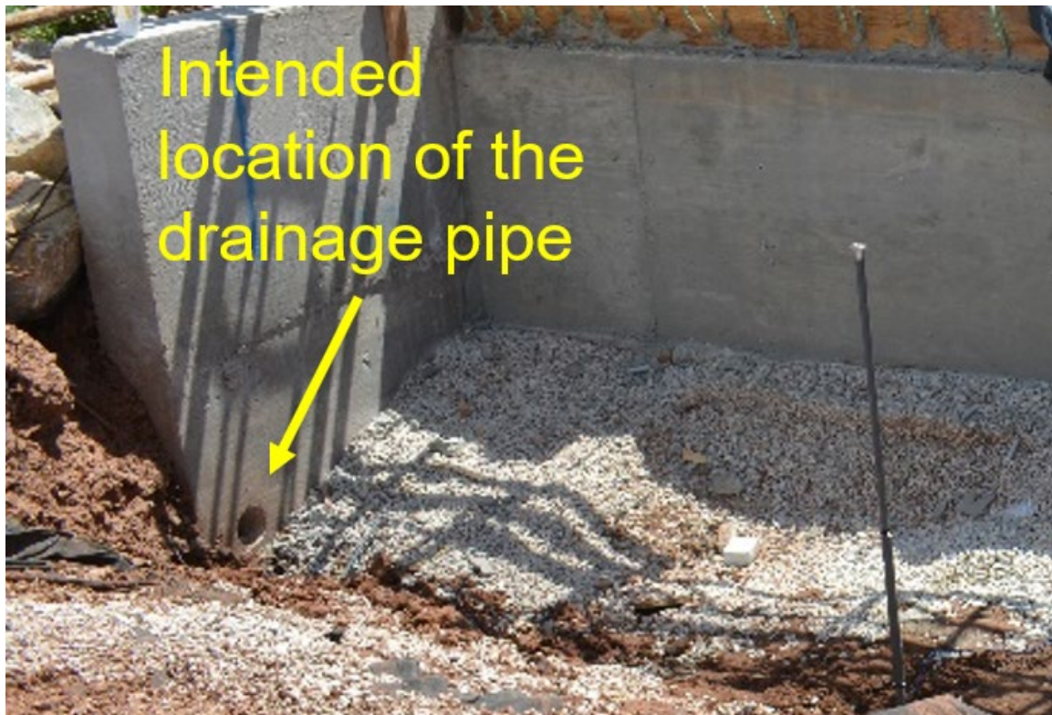
Figure 11.5: According to drawings, a perforated drainage pipe was planned to pass through the wingwall (west abutment view, phase 2)
