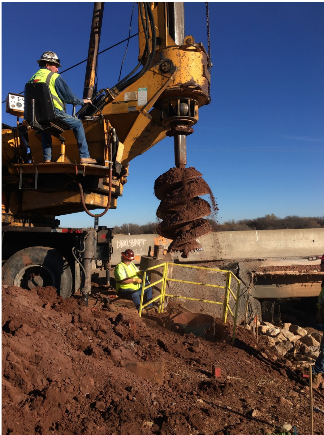
Figure 8.36: Drill bit exiting hole to dump excavated soil
