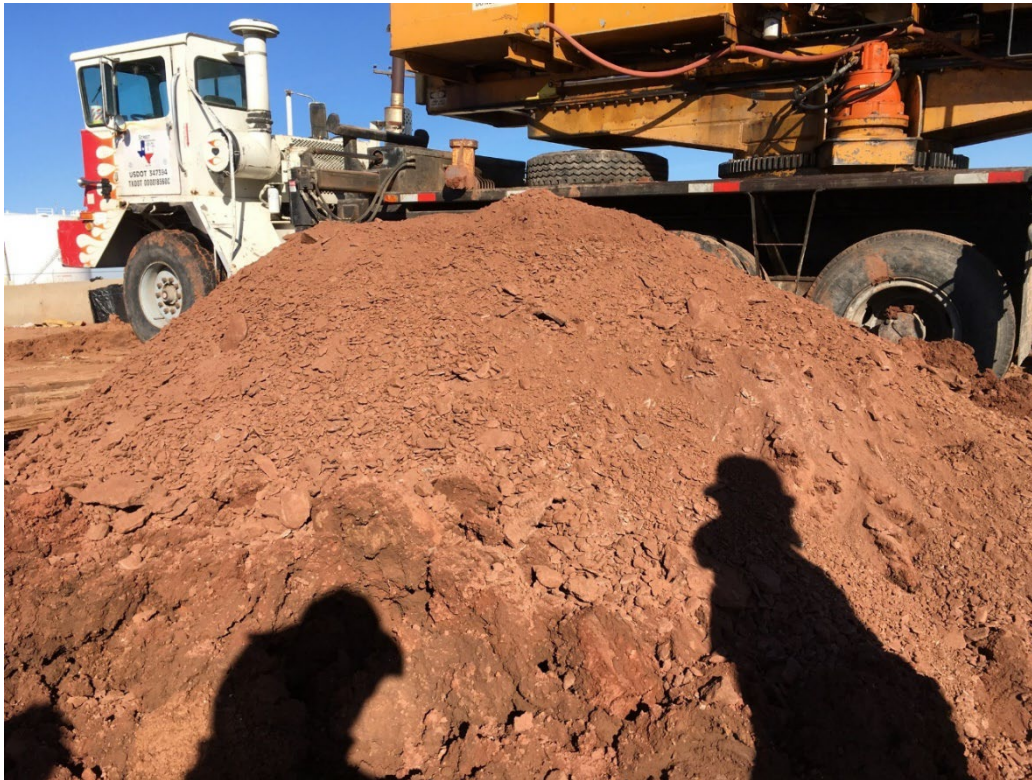
Figure 8.40: Heap of soil excavated from drilled shaft (Note broken shale pieces on top (25 ft and below) and wetter/plastic material removed beforehand)
