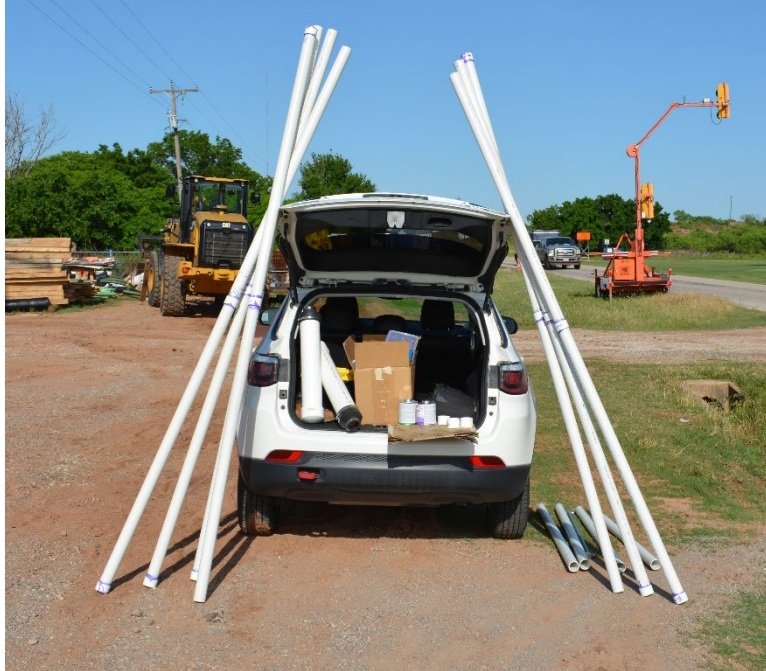
Figure 8.54: Five-ft PVC conduits transported to China Creek Bridge to house SAAV sensors in drilled shafts (conduits pictured have been assembled into 10-ft sections using PVC cement and couplers)
