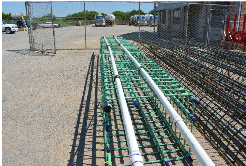
Figure 8.55: PVC conduits assembled into 40-ft sections using additional couplers and joint reinforcement
