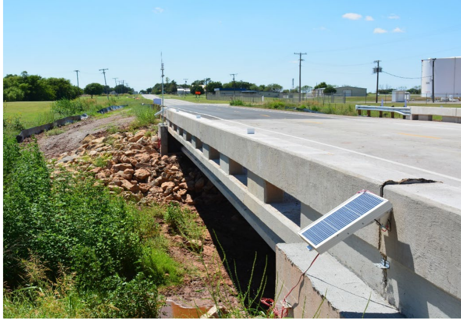
Figure 8.88: Solar panel mounted on south railing of east end of China Creek Bridge
