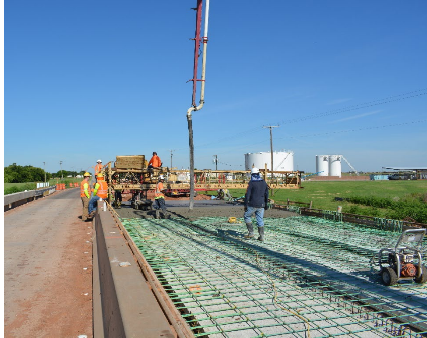
Figure 8.76: Phase 2 deck concrete placement
