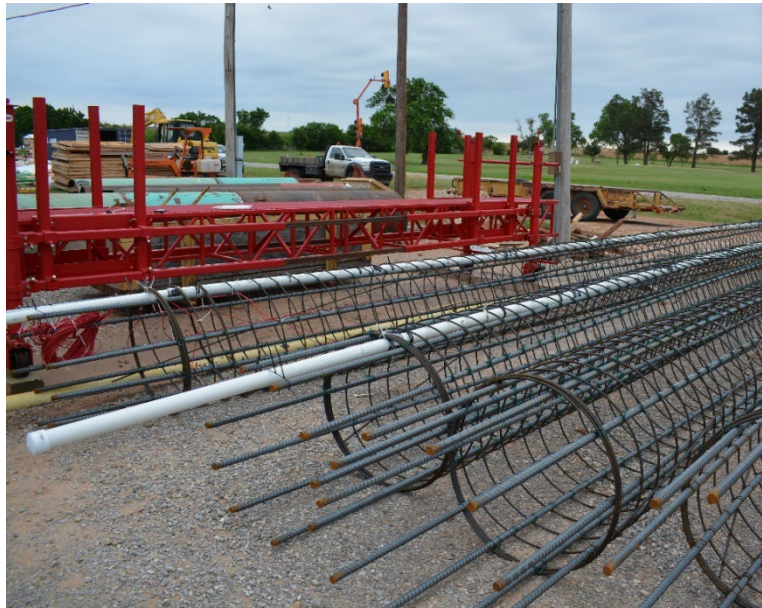
Figure 8.58: Assembled PVC conduits attached to drilled shafts to serve as SAAV housing
