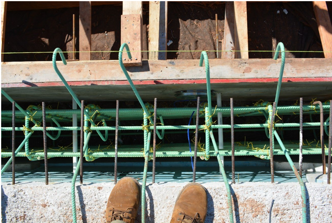
Figure 8.44: Top view of earth pressure cell (GK-4810) installed on inside of form on west abutment backwall, March 2020 (photographer standing on one precast panel placed on deck)
