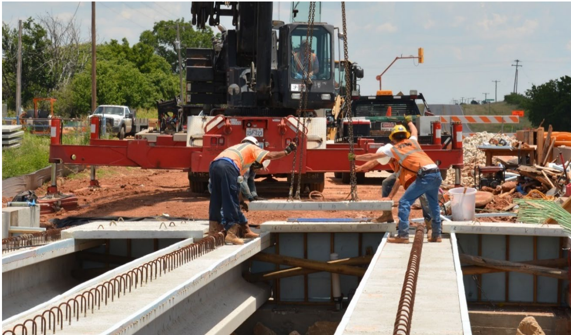
Figure 8.75: Placement of precast concrete panels on deck
