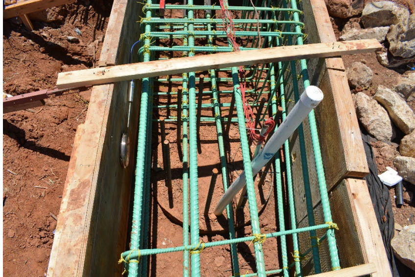
Figure 8.64: (a) West abutment cap pressure cell (before formwork completion); and (b) east abutment pressure cell (after formwork completion)
