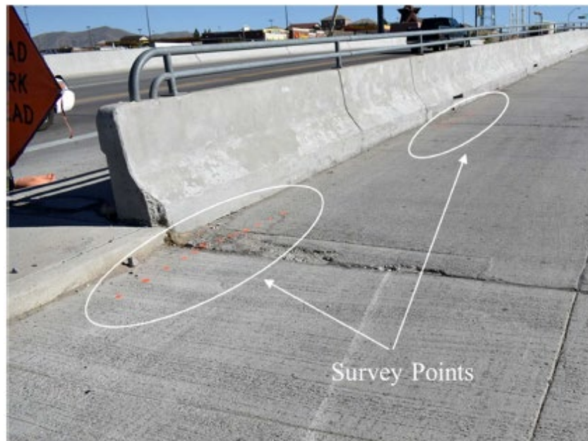
Figure 4.5: Photograph of survey points (orange dots) on Anthony IAB west transition from roadway to approach slab and approach slab to bridge deck
