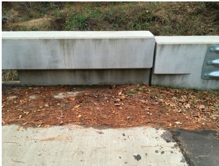
Figure 4.13: Differential settlement revealed by the difference in height of guardrails between approach slab and bridge deck
