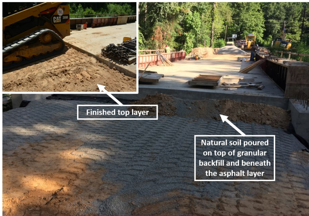
Figure 4.15: Use of clayey natural soil as base material for asphalt pavement in approach slabs
