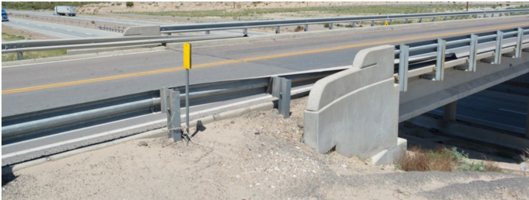
Figure 2.7: El Paso County SIAB roadway-to-bridge-deck transition (from west end looking northeast)
