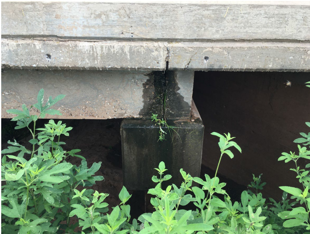
Figure 8.4: Seepage of water through deck joints
