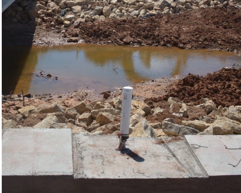
Figure 8.69: Capped SAAV conduit on east abutment
