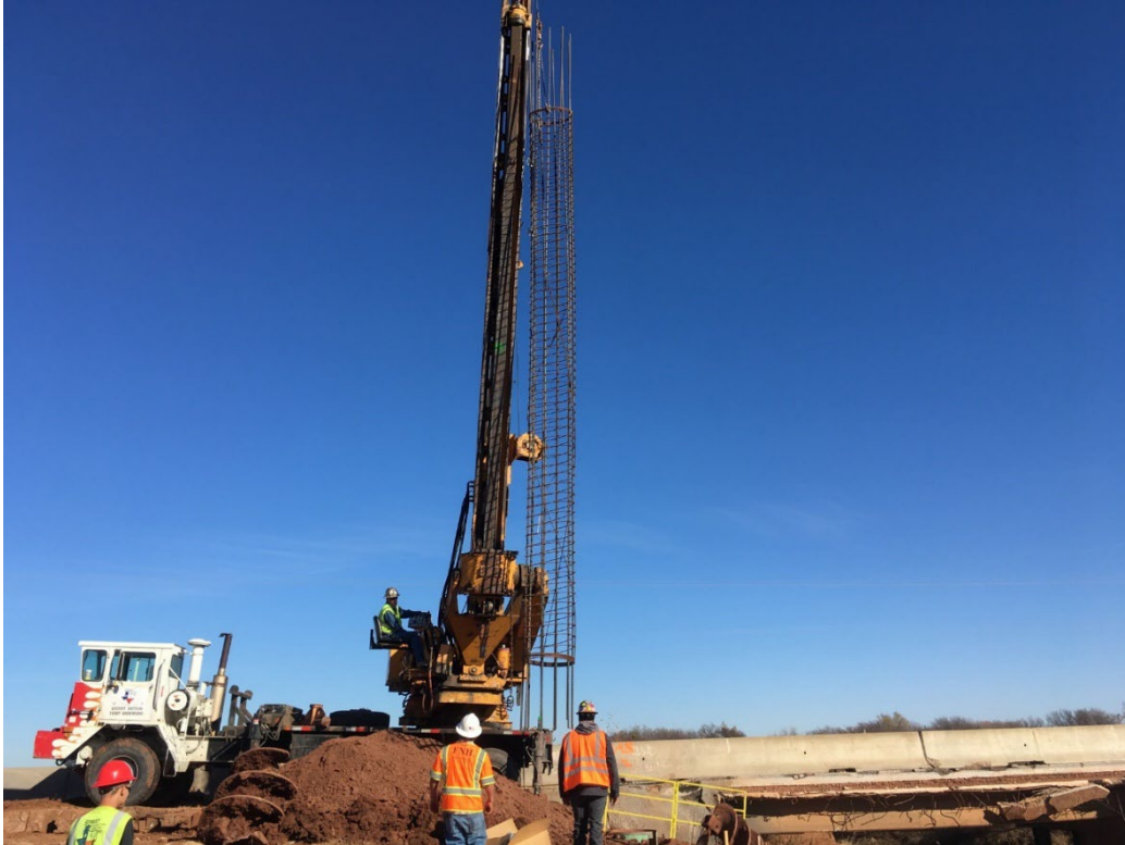
Figure 8.41: Lowering of rebar cage
