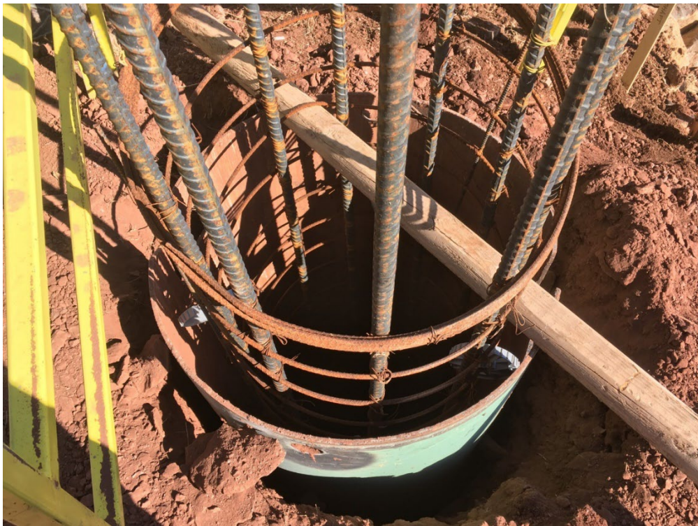
Figure 8.42: Propping rebar cage to keep it off the bottom of the hole before concrete pouring
