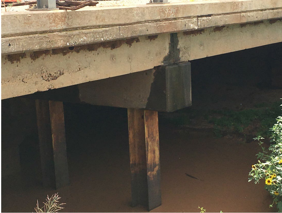
Figure 8.3: Corroded bents under China Creek Bridge to be replaced
