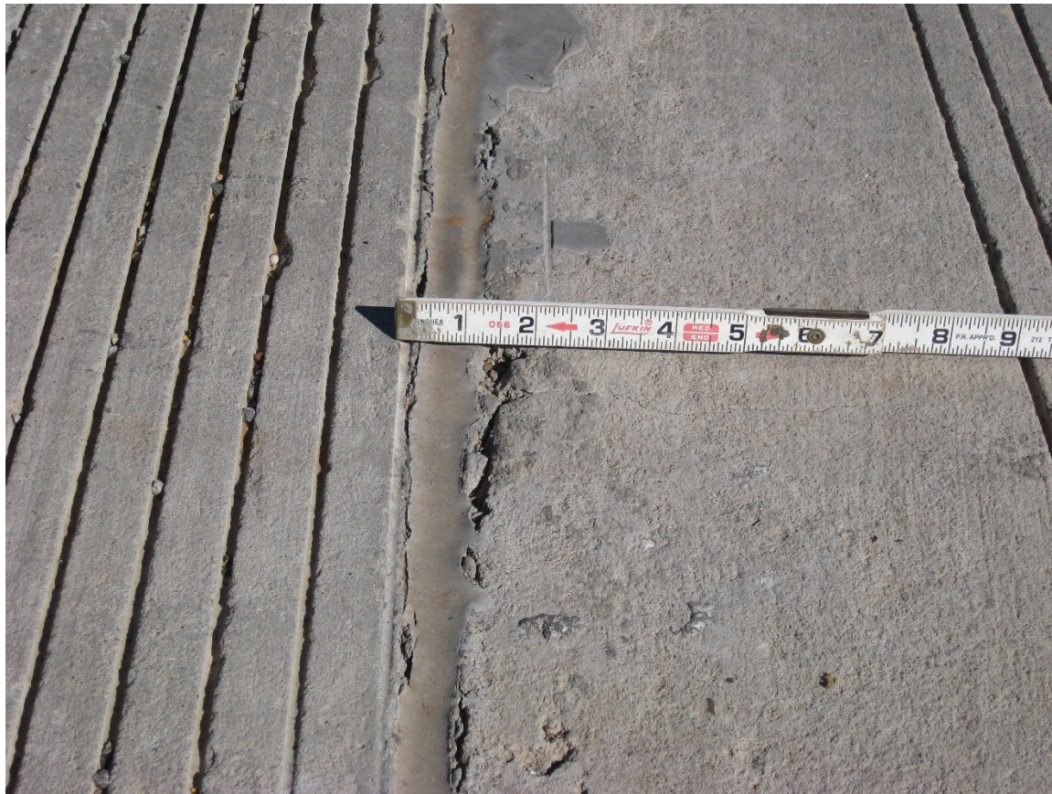
Figure 8.116: West approach expansion joint appears to be intact and undamaged (photograph taken by Samuel Groves, TXDOT, on February 22, 2021)
