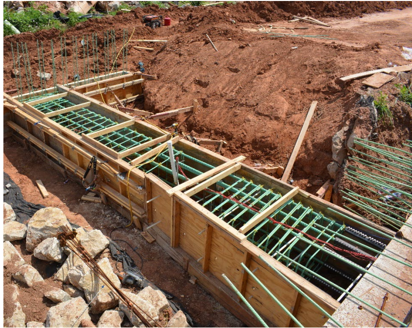
Figure 8.63: Formwork for construction of pile caps and wingwalls
