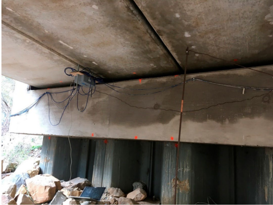
Figure 4.16: Traces of water on the northern abutment cap under the bridge deck
