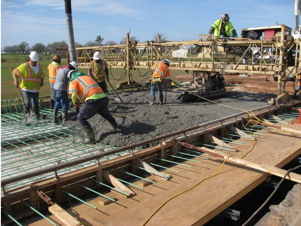
Figure 8.51: Concrete placement on deck, phase I, March 2020
