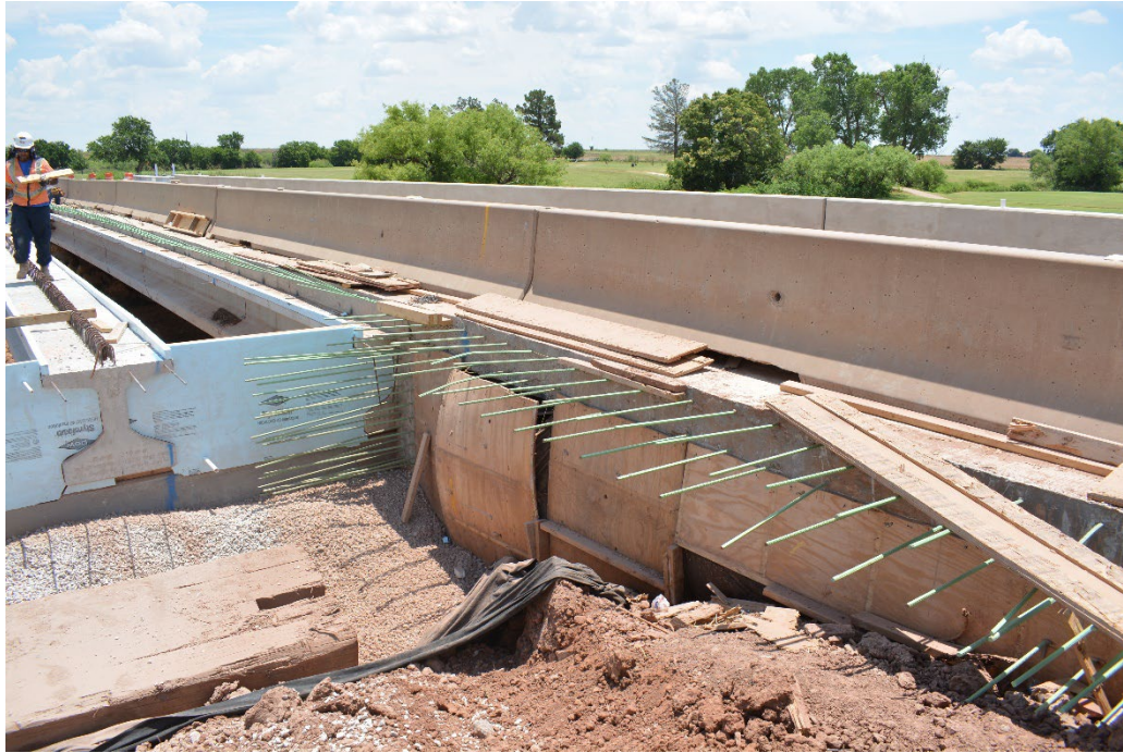
Figure 11.2: Buckling of wooden forms retaining the backfill placed during phase 1 on the west end of the bridge
