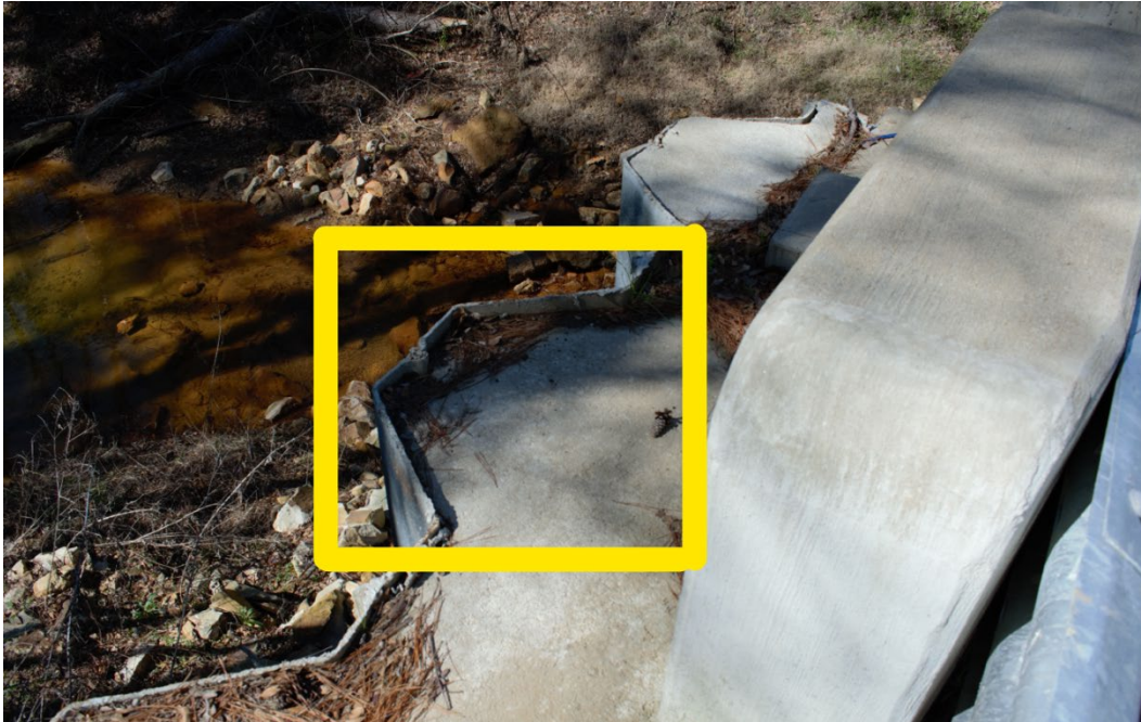
Figure 4.19: Settlement of concrete placed behind wingwalls (southwest wingwall)
