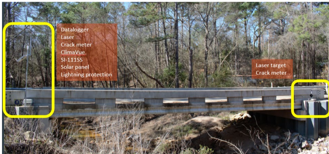
Figure 7.18: Equipment installed on Mack Creek SIAB in January 2020
