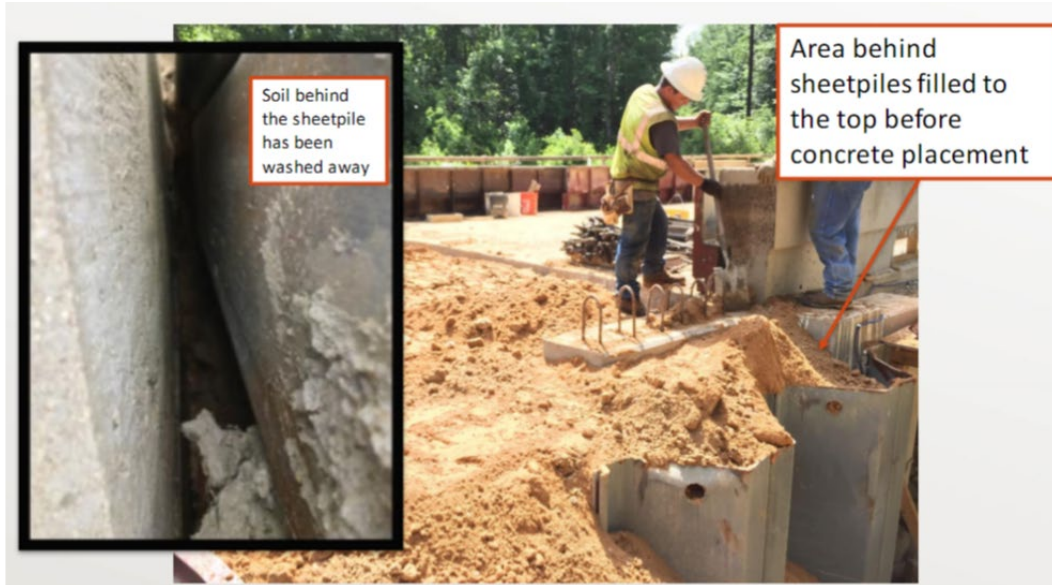
Figure 4.20: Loss of fill placed behind wingwalls due to erosion (left image shows an overhead view of the gap between sheetpile and pile cap)
