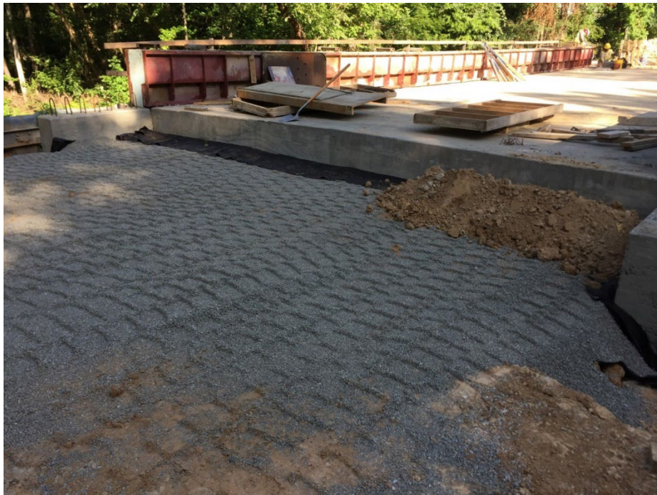
Figure 11.4: No separation between base material and backfill material
