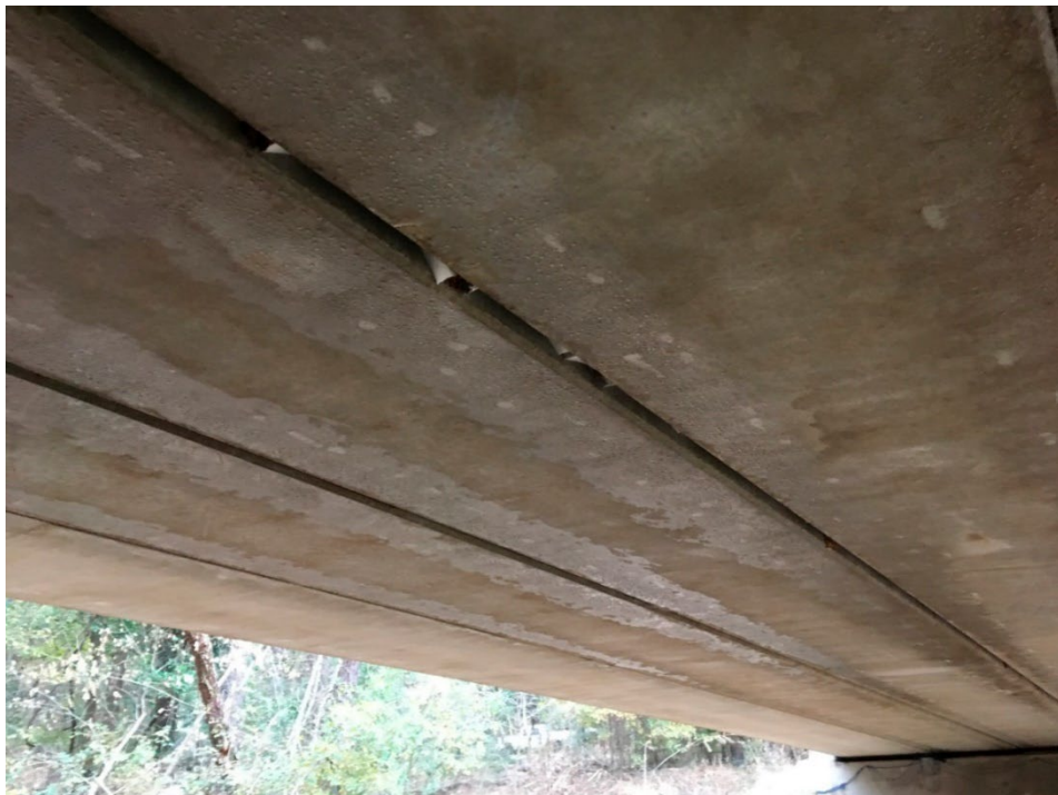
Figure 4.17: Water gathered under the box girders (view from south abutment)
