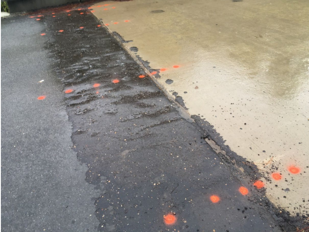
Figure 4.12: Repaved approach slabs of Mack Creek Bridge (orange dots are survey points)
