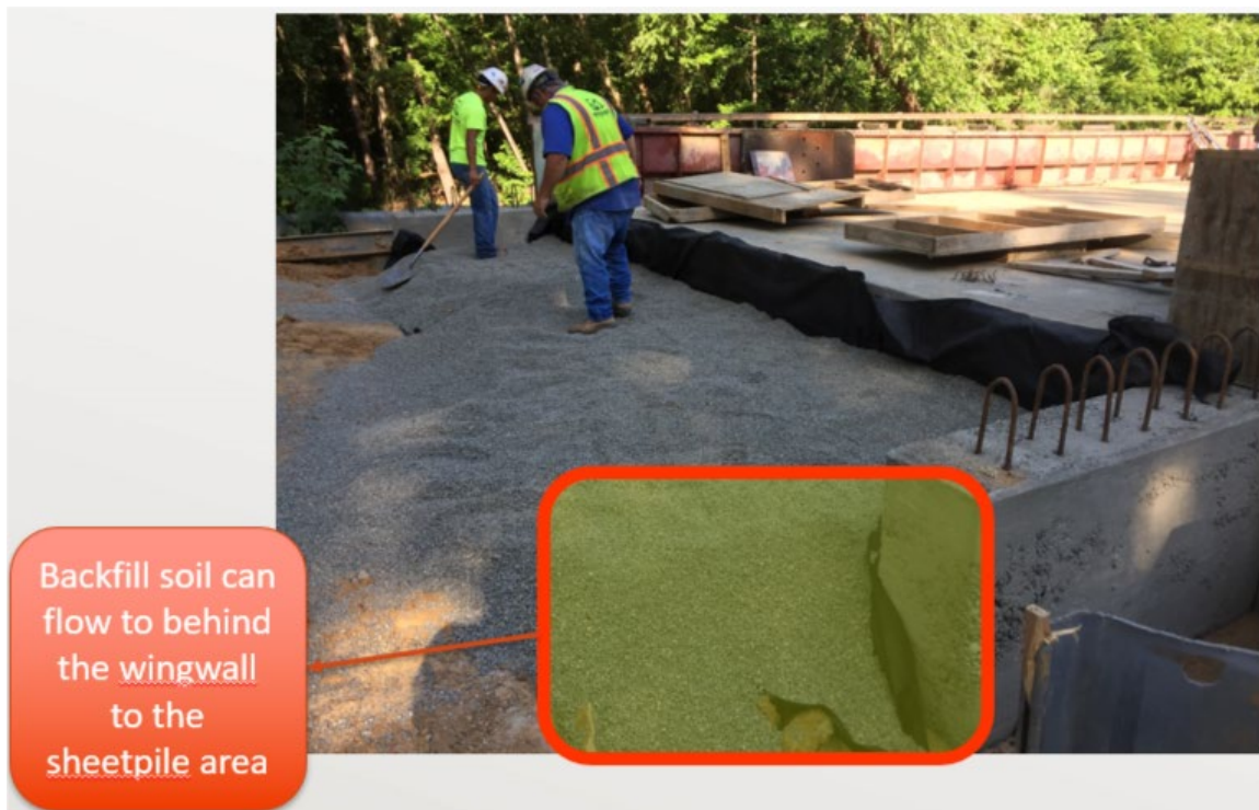
Figure 11.1: Backfill material flowing behind wingwall
