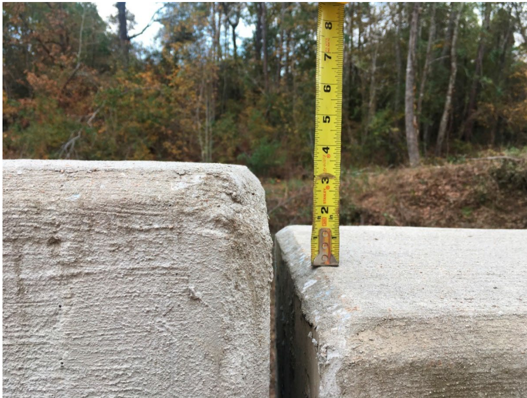
Figure 4.14: Differential settlement between guardrails constructed on top of the deck and south approach slab (November 2019)
