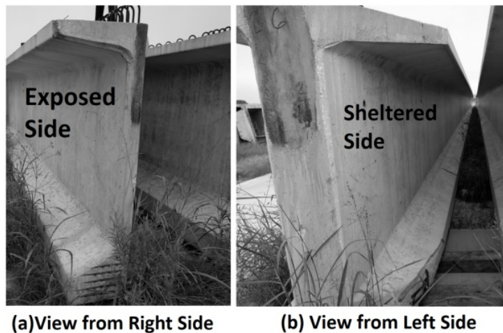
Figure 3.1: Typical overcast girder showing (a) exposed face and (b) sheltered face
