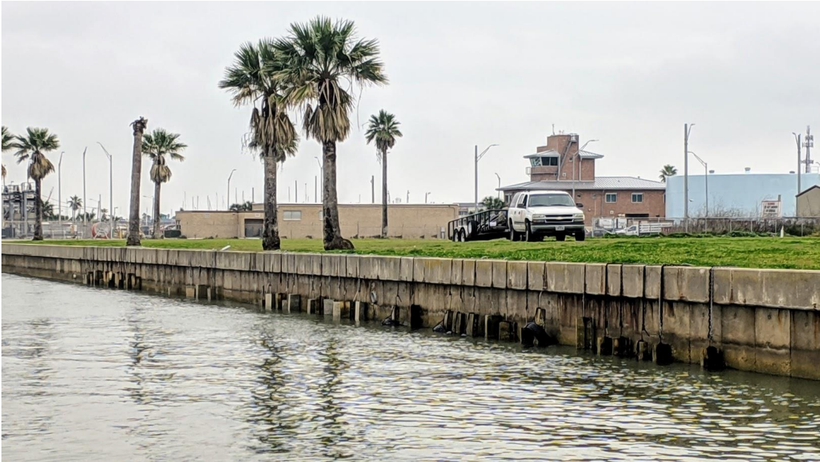
Figure 2.5 Texas Marine Exposure Site in Port Aransas
