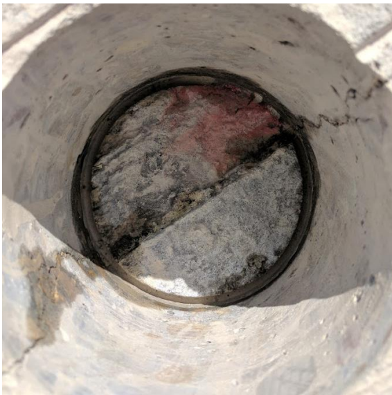
Figure 7.12 Intersection of two precast panels below cast-in-place slab (left), and cracking visible throughout core and around aggregate (right)
