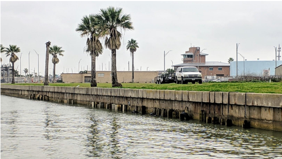
Figure 3.1 Marine Exposure Site in Port Aransas
