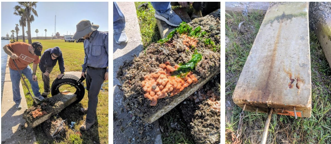
Figure 3.37 Exposure block visual examination: biological growth (left and middle) and rust staining (right)
