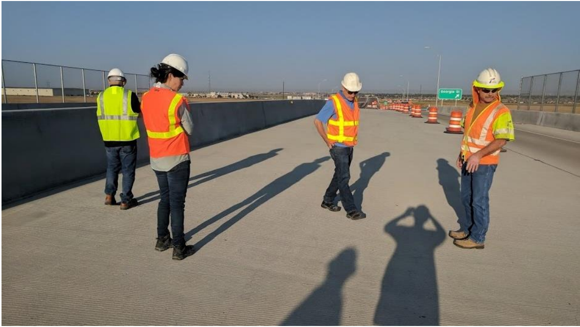
Figure 7.6 Loop 335 at BNSF RR inspection
