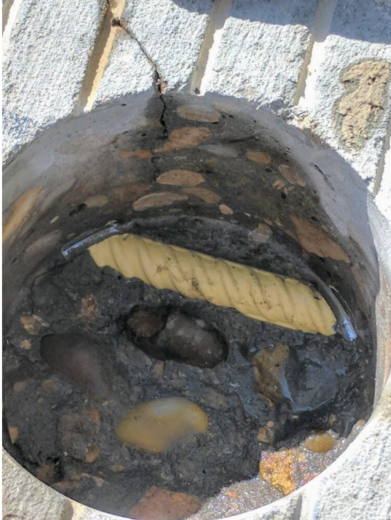
Figure 7.11 Rebar struck while coring
